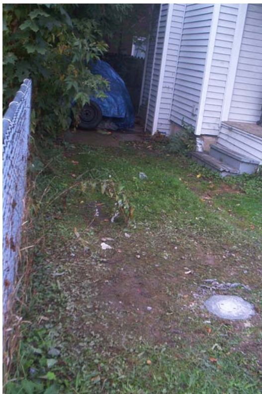
Microwell surface completion.
