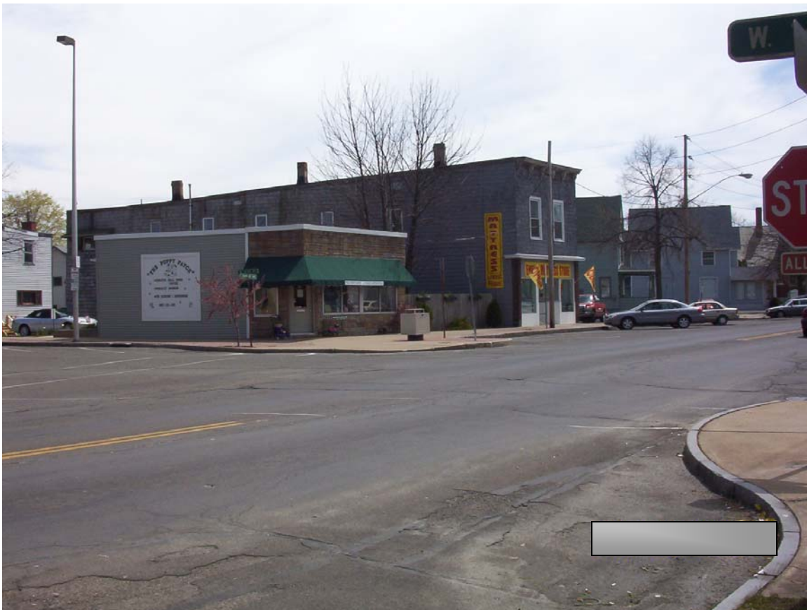
Looking southeast at property (two story gray building).
