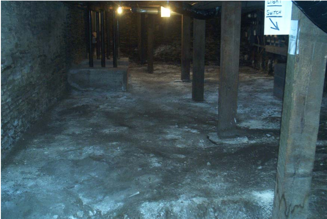
Looking west into basement. Concrete base and metal supports on left side reportedly installed to support former dry cleaning equipment on floor above.
