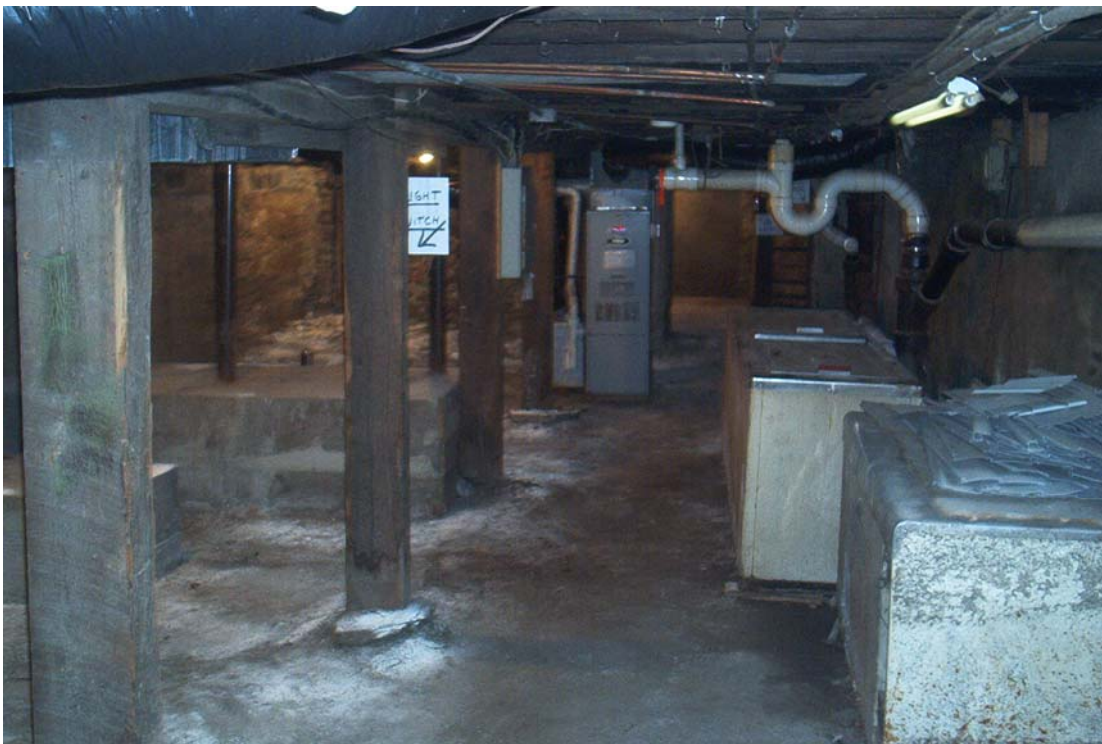
Looking east across basement.
