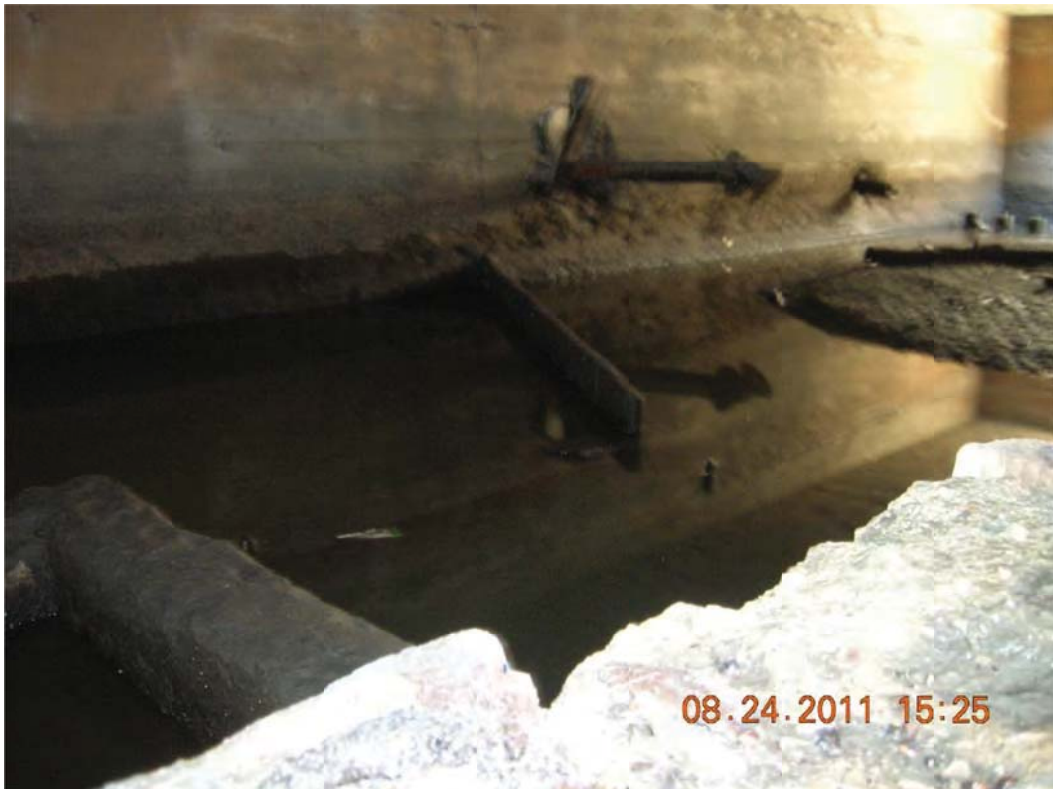
Picture #9- Inside Oil Skimmer looking NW at pipe penetrations and internal baffles
