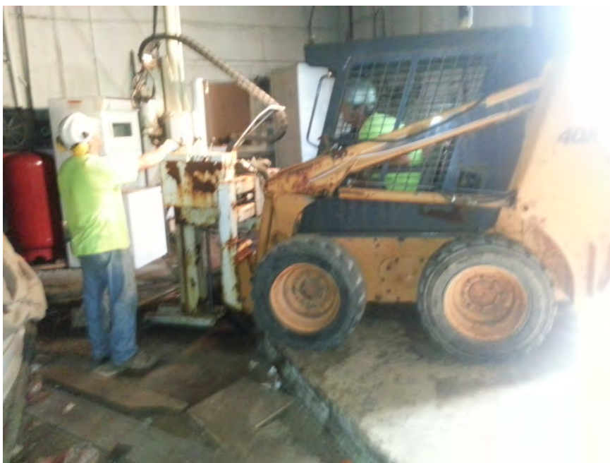
Photo 14: 08/29/13 – Hydraulic direct-push unit (geoprobe) location GS-01/CC-01.
