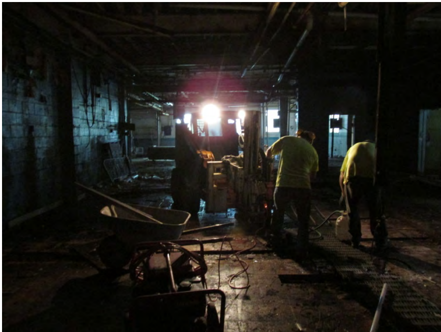
Photo 15: 08/29/13 – Hydraulic direct-push unit (geoprobe) location GS-02/CC-02.
