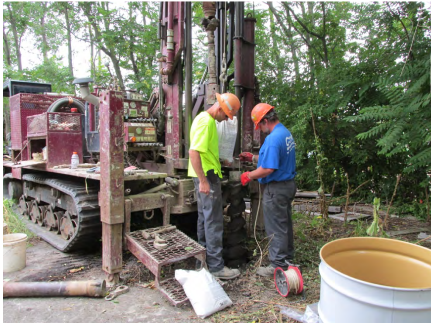
Photo 8: 08/28/13 – Drilling at location MW-02.
