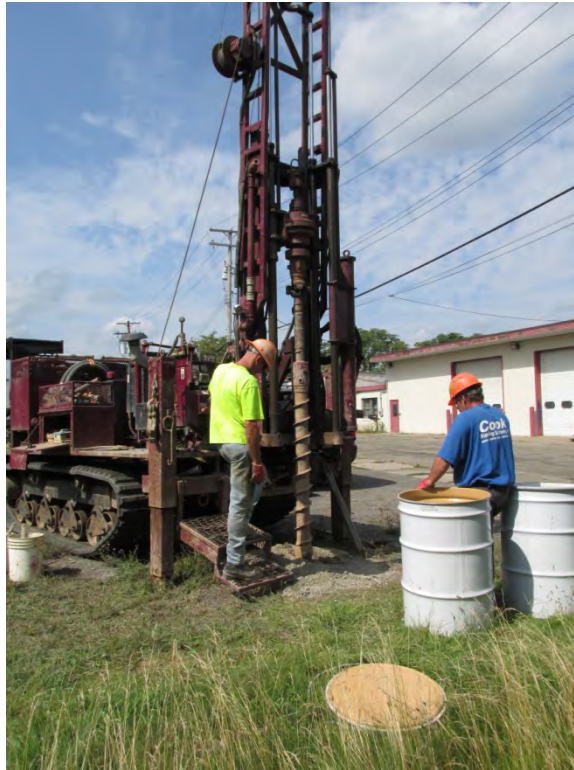
Photo 5: 08/27/13 – Drilling at location MW-01.
