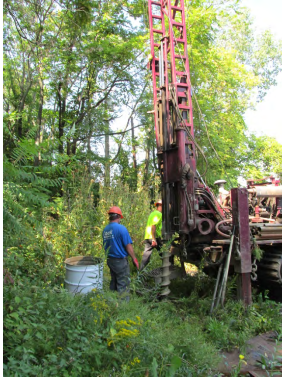
Photo 11: 08/28/13 – Drilling at location MW-03.
