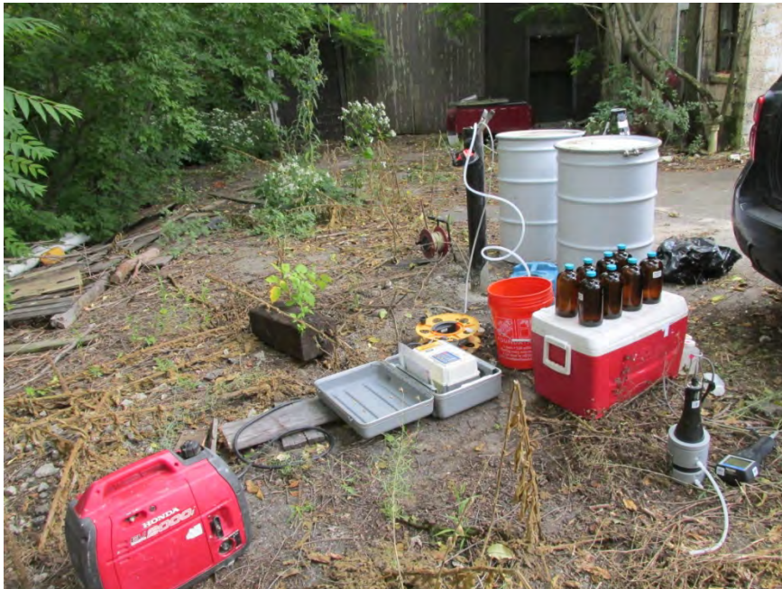
Photo 10: 09/05/13 – Sampling equipment setup at monitoring well location MW-02.
