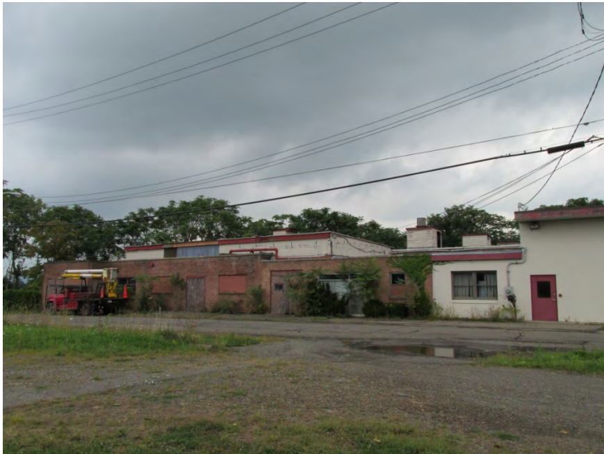
Photo 2: 08/26/13 – Triple Cities Metals Finishing building – north end.
