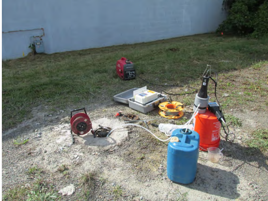
Photo 7: 09/05/13 – Equipment setup at monitoring well MW-01.
