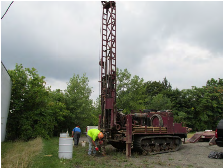
Photo 4: 08/26/13 – Setting up drill rig at location MW-01.
