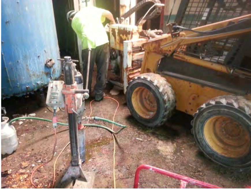
Photo 17: 08/29/13 – Hydraulic direct-push unit (geoprobe) location GS-06.
