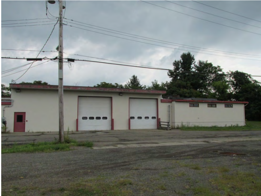
Photo 1: 08/26/13 – Triple Cities Metals Finishing building – south end.
