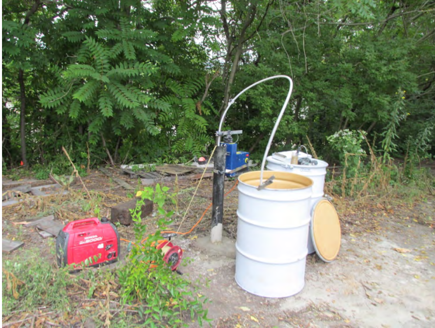
Photo 9: 08/29/13 – Well development at monitoring well location MW-02.
