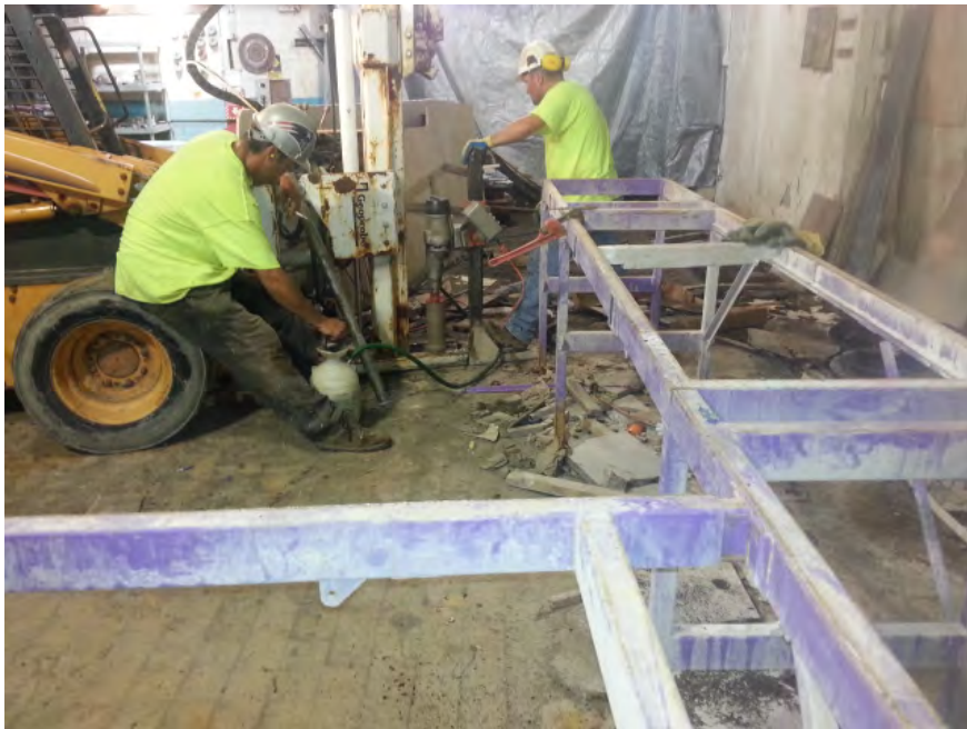
Photo 18: 08/29/13 – Hydraulic direct-push unit (geoprobe) location GS-08.
