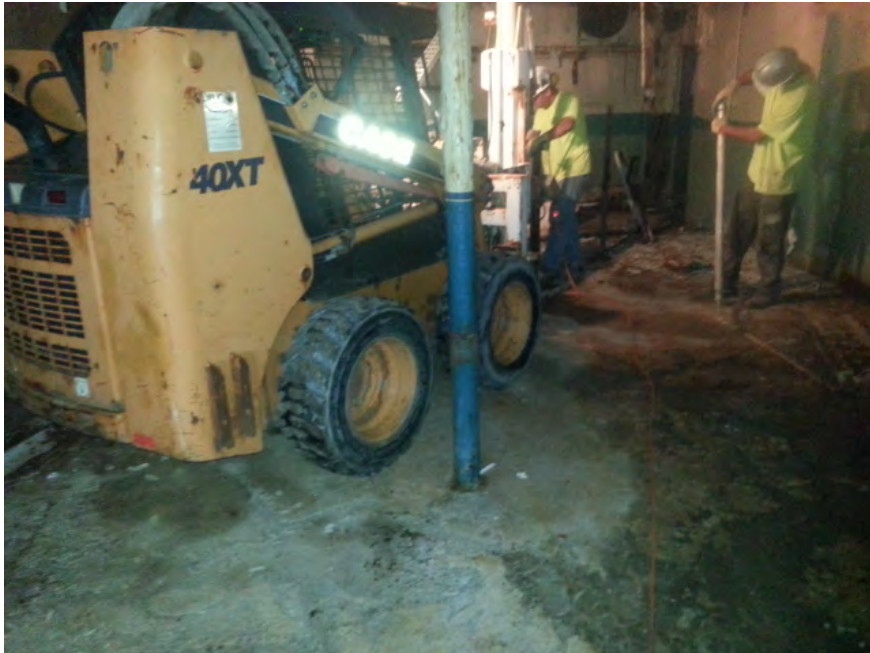
Photo 15: 08/29/13 – Hydraulic direct-push unit (geoprobe) location GS-02/CC-02.
