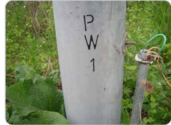
Shot 9: Pumping Well PW-1 Date: May 24, 2012
