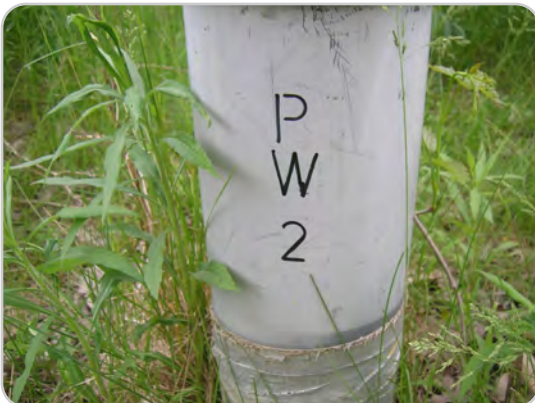
Shot 10: Pumping Well PW-2 Date: May 24, 2012
