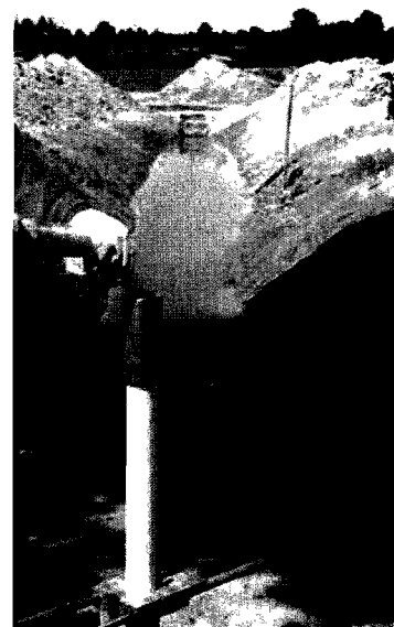
Underground oil pipeline leak assessment. Three 150 ft. (45m) installations. Two point rising head permeability tests were conducted in each interval of the Multilevel System. (See diagram showing contaminant distribution at left.)
