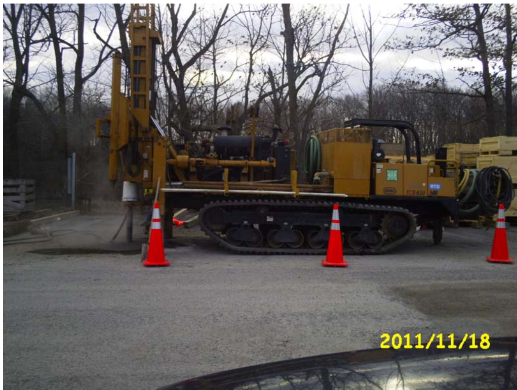
Drilling of BRW-1 after casing was installed (completion to depth through bedrock).
