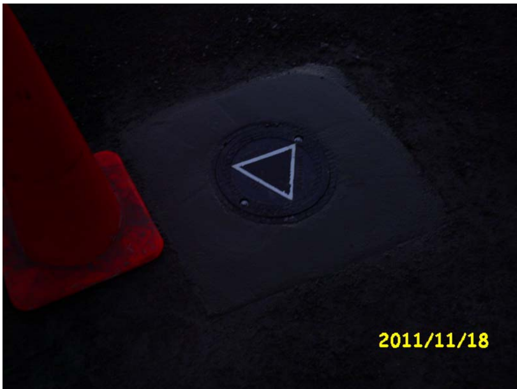
View of BRW-2 completed with well pad.
