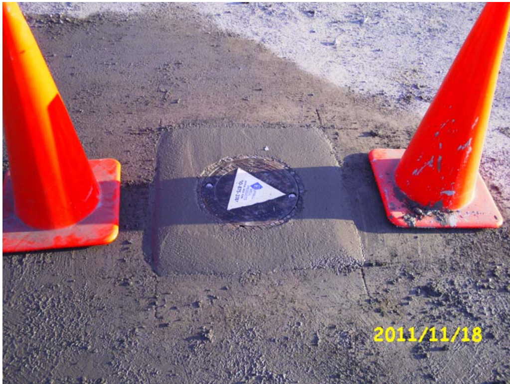
View of BRW-1 completed with well pad.
