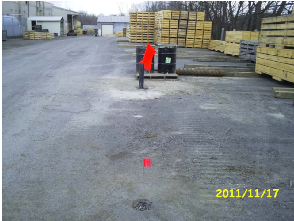
View of BRW-1 after casing was installed, flag in the casing stick up for visual purposes (GESB-14 is the boring depicted by the pink flag at the bottom of the picture).
