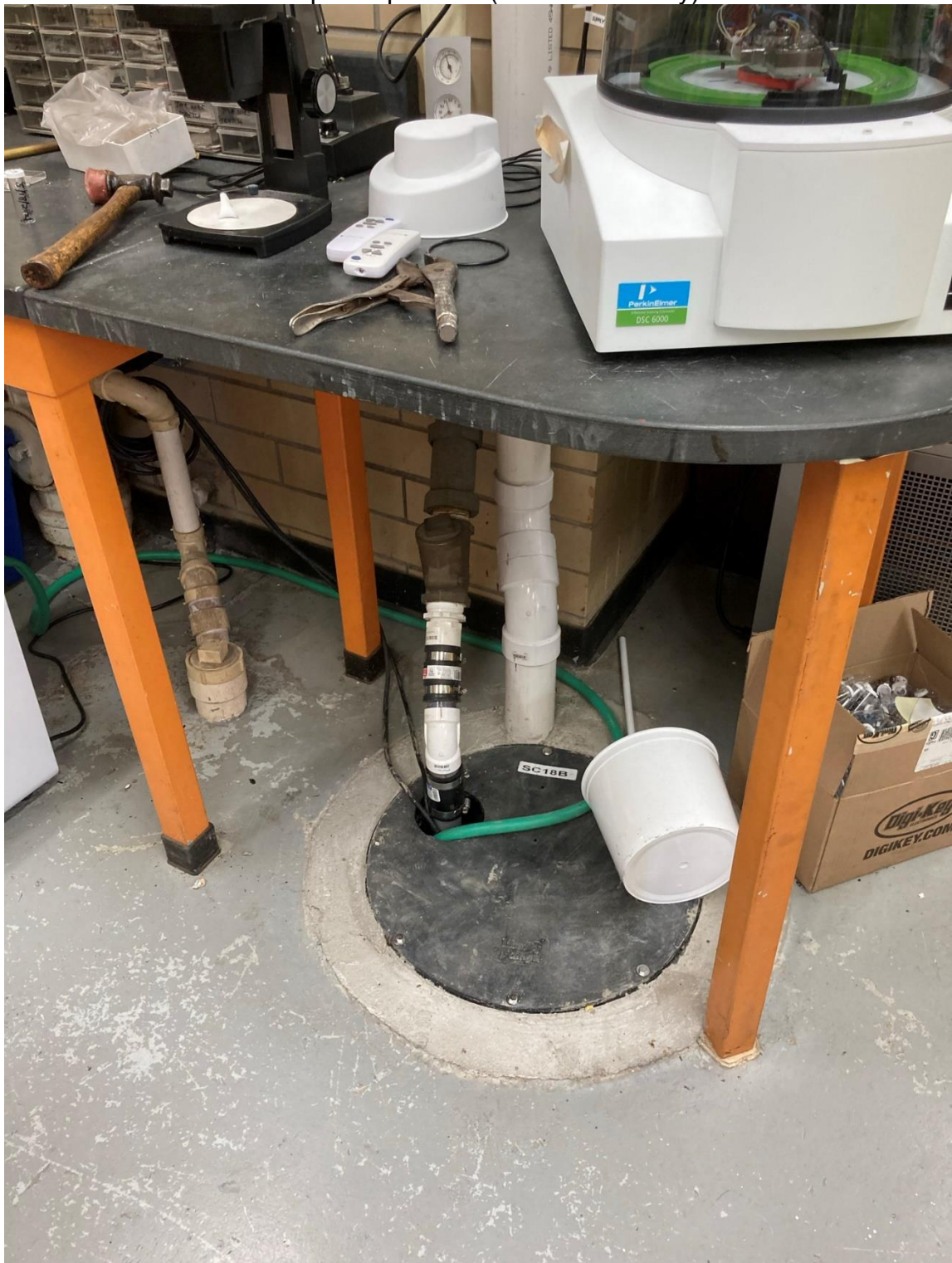
Sump Pump in Lab (condensate only)
