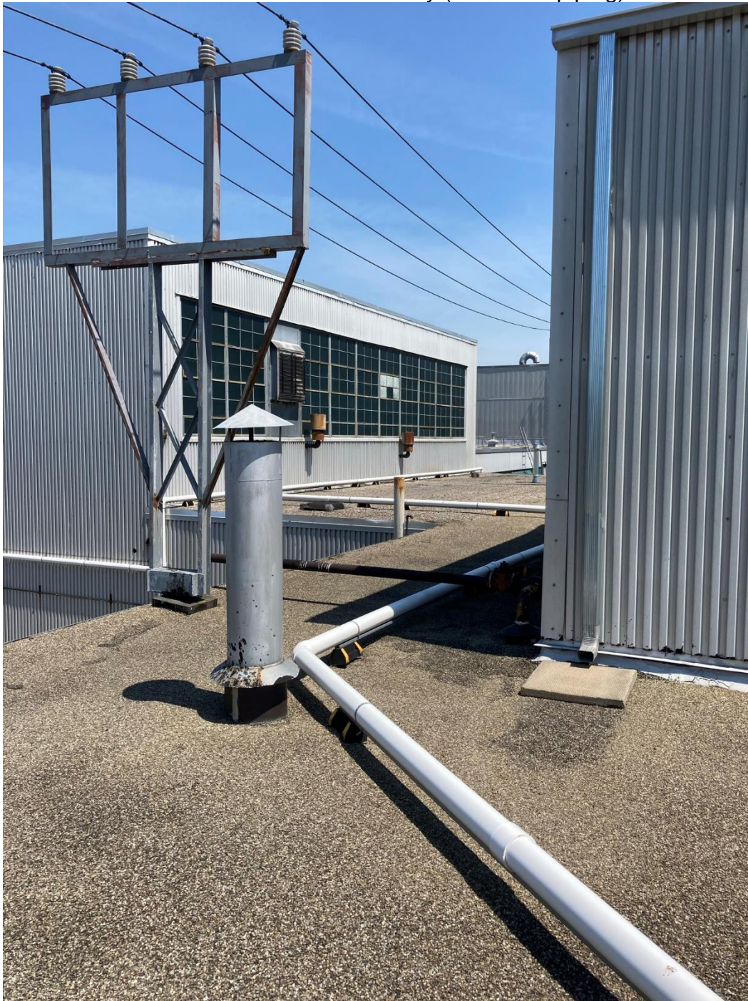
Roof of PCORE Facility (extraction piping)
