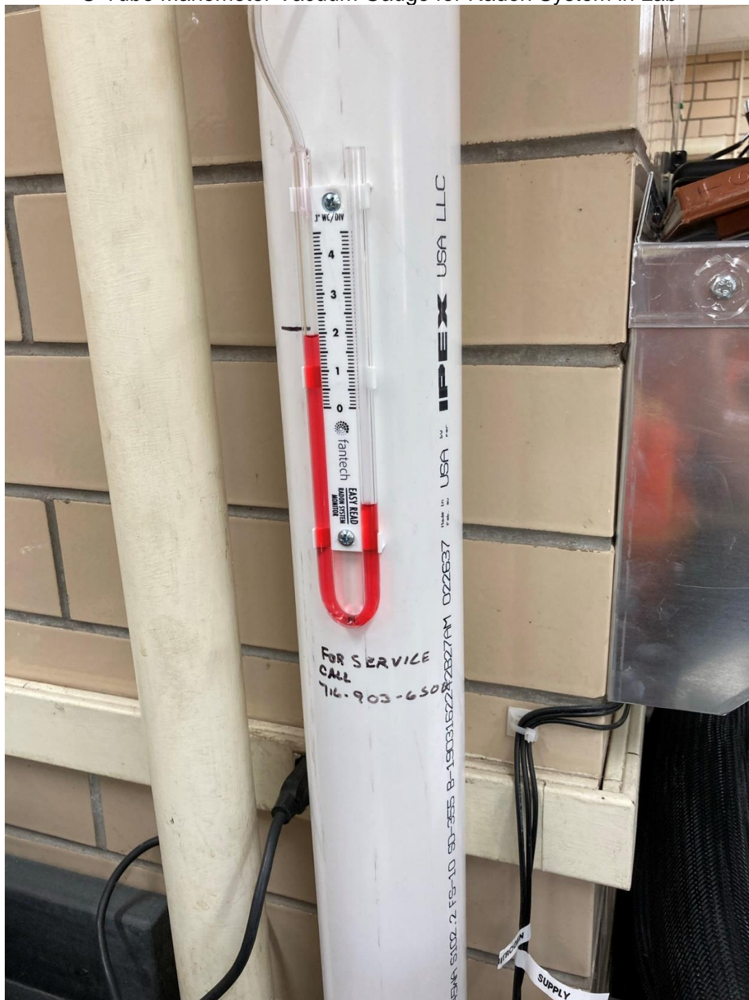
U-Tube Manometer Vacuum Gauge for Radon System in Lab
