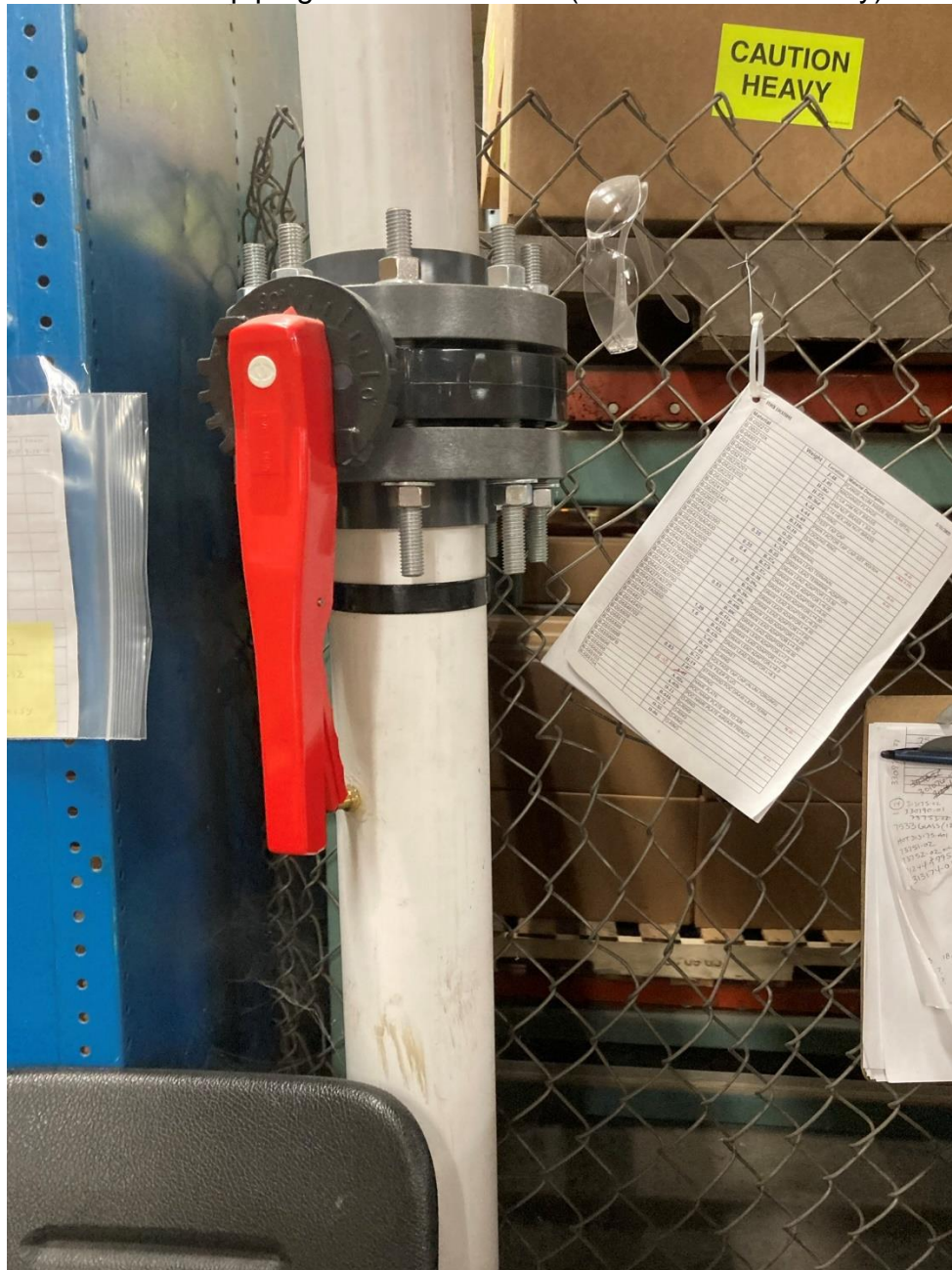
Extraction piping and shutoff valve (within PCORE facility)
