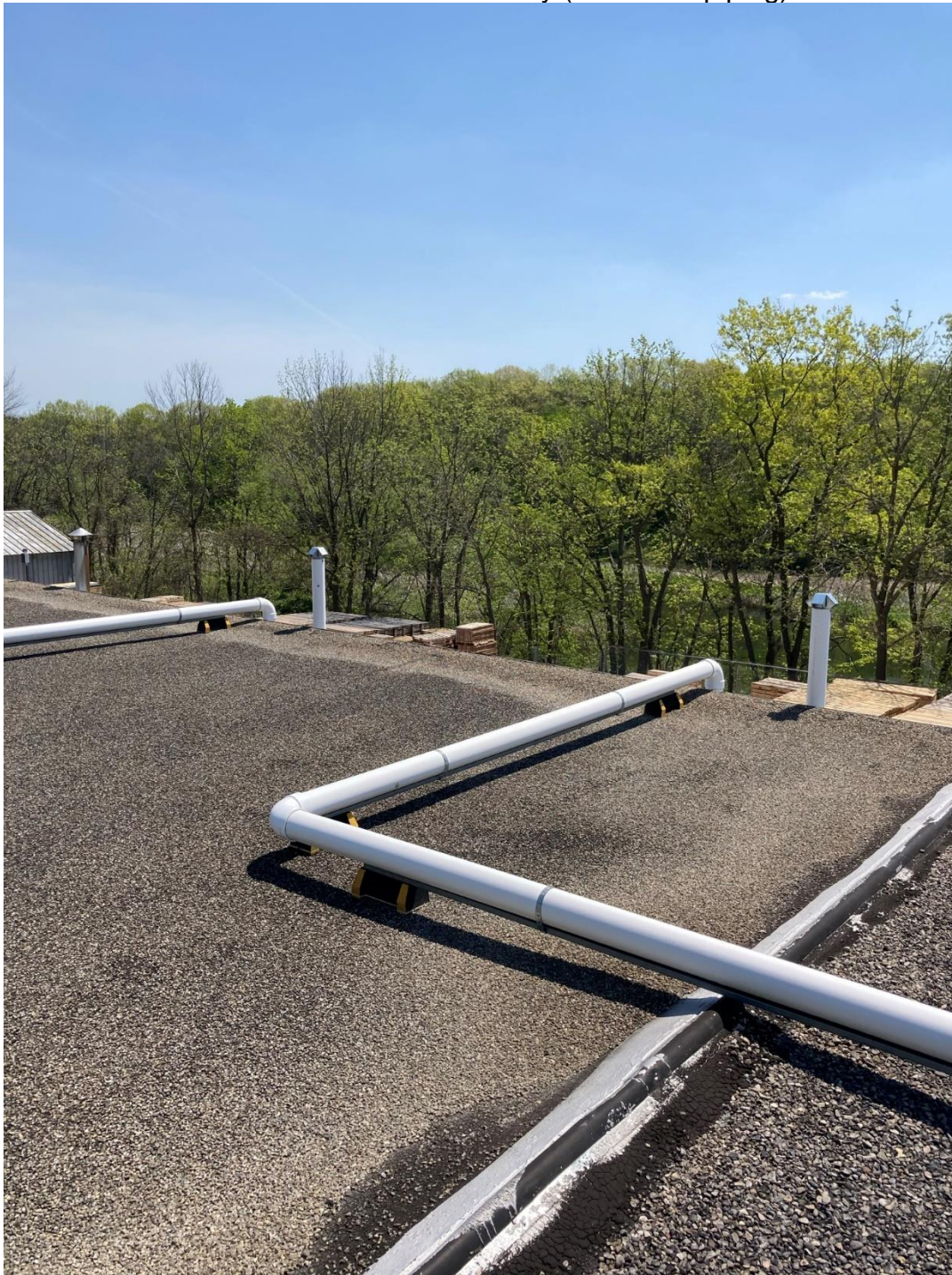
Roof of PCORE Facility (extraction piping)
