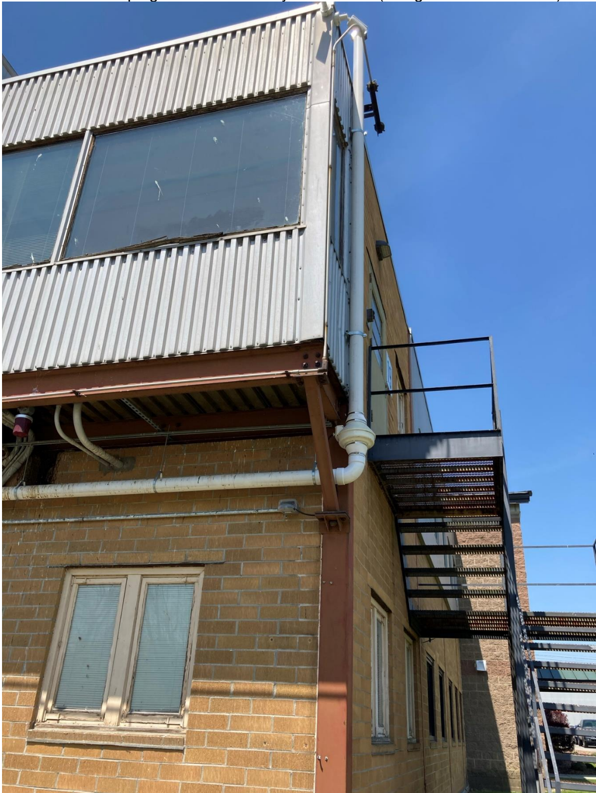
Extraction Piping for Radon Fan System in Lab (along back corner of lab)
