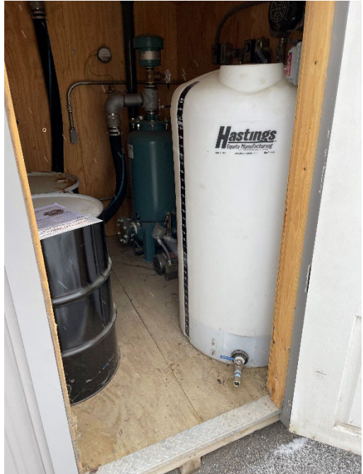
Knockout tank PCORE Shed 1
