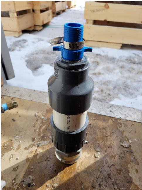
Fittings used for vacuum testing
