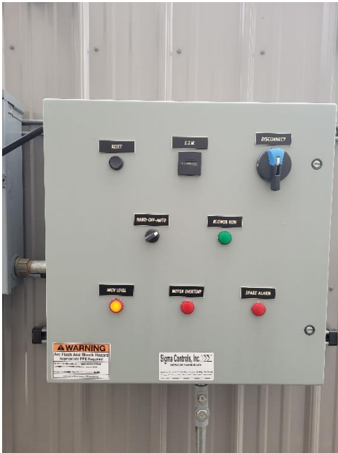
PCORE-02 system off upon arrival due to High Level alarm.
