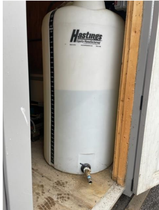
Knock out tank in right shed (SSDS-2)
