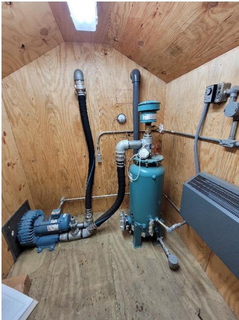
Collecting O&M readings in B-35 SSDS.
