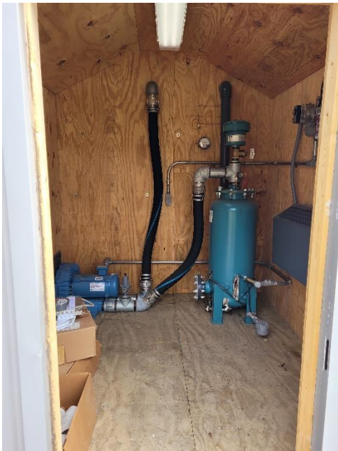
Collecting O&M readings in B-35 SSDS.
