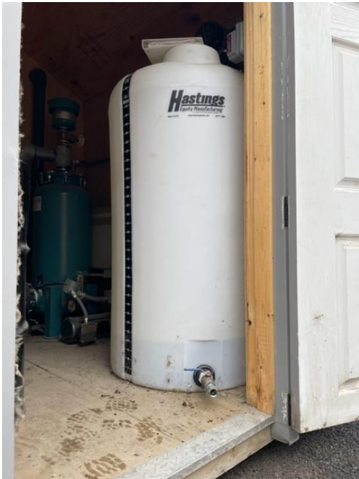
Knock out tank in left shed (SSDS-1)
