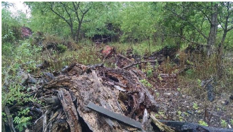
Photo 19. Homogeneous area P12-2; Dark brown composite wood material and general setting in P12; Trace Amount Asbestos Detected.
