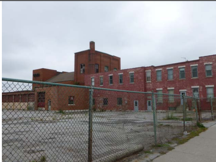
East side of the Main Building.
