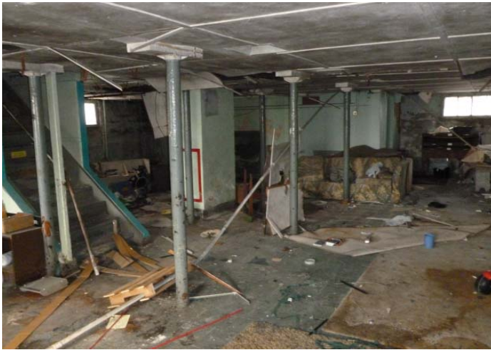
Basement in from area of Main Building.
