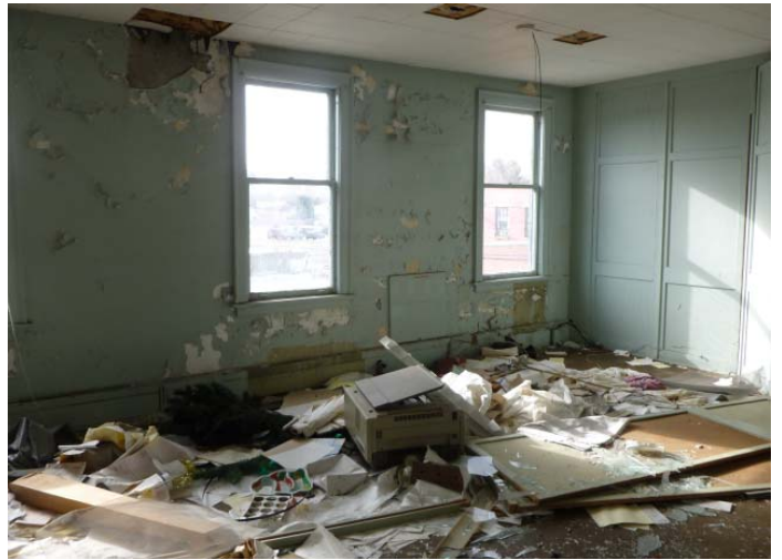
Second floor former office area in Main Building.
