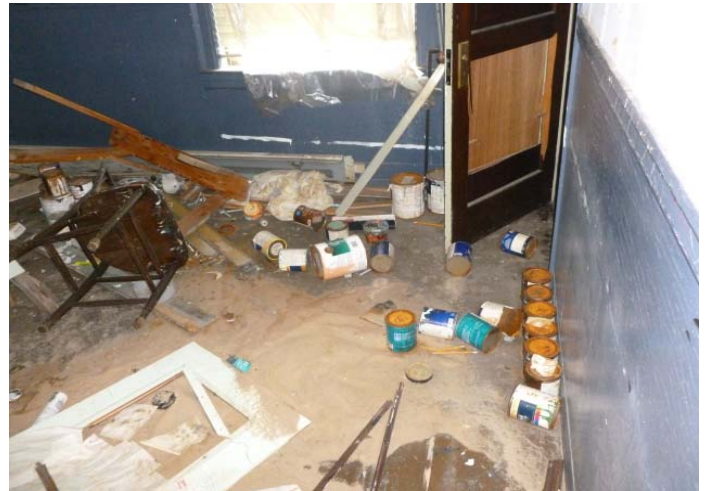
Second floor former office area in Main Building; several paint cans.
