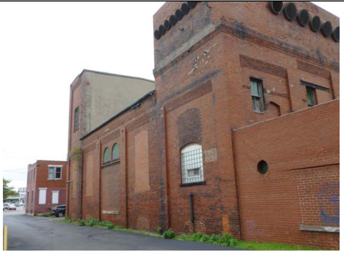
West side of the Main Building.
