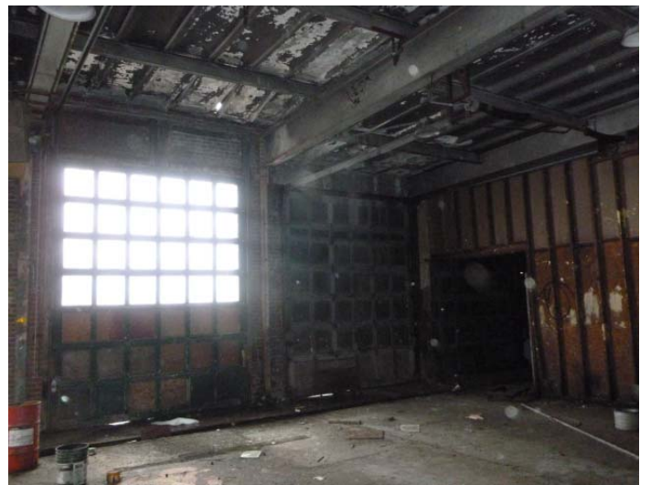
Shop area of Main Building.
