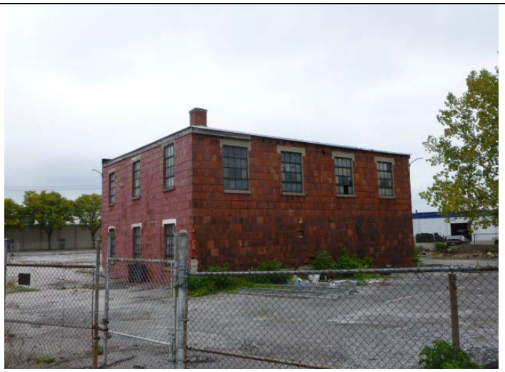
South and west sides of the Vacant Garage.
