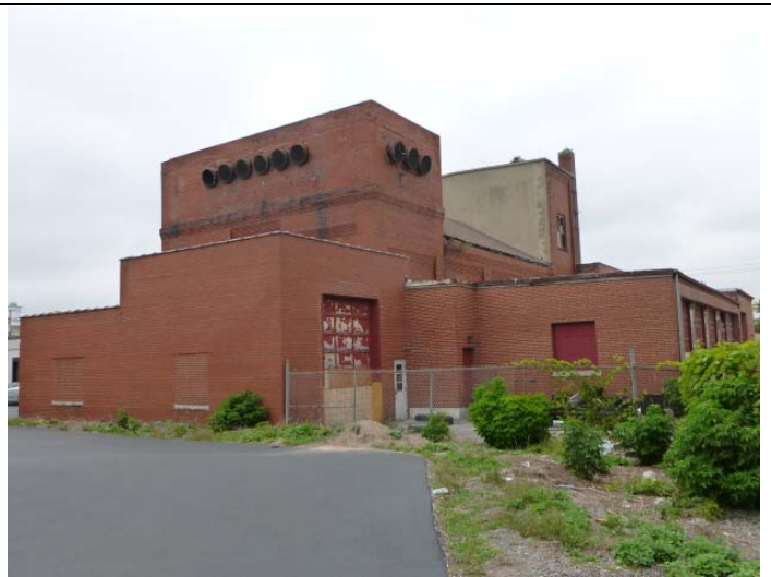
South side of the Main Building.
