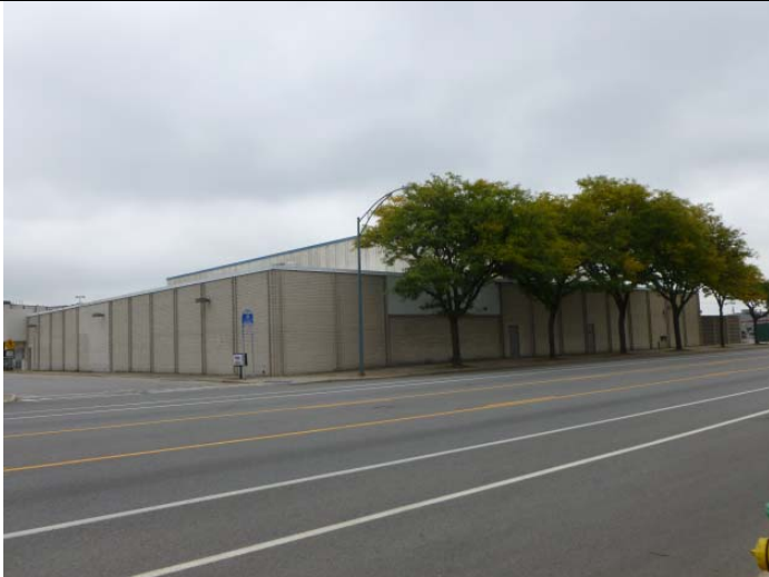
North adjacent property.
