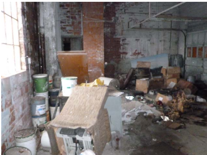
First floor former storage area in Main Building.
