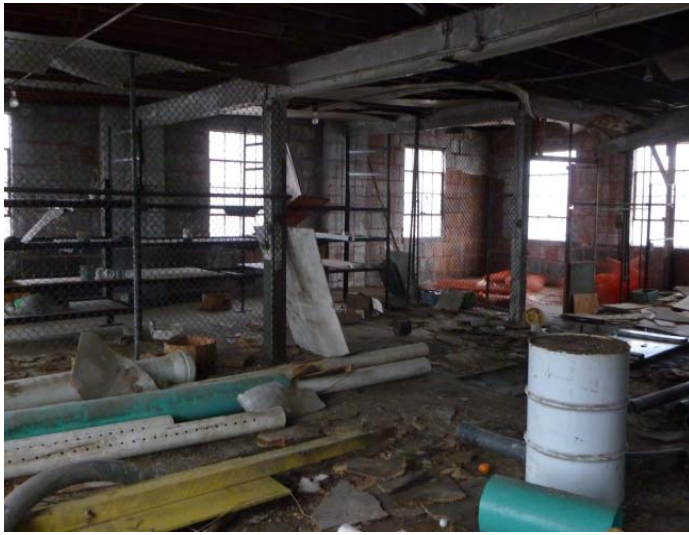
Second floor former storage area in Vacant Garage.
