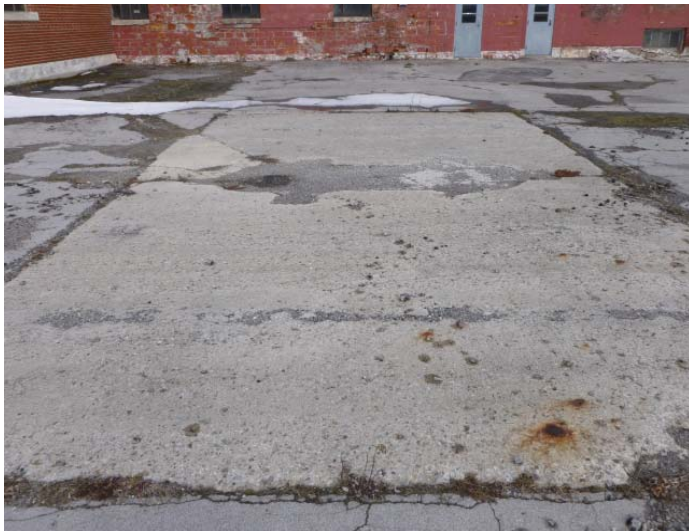
Area of gasoline and diesel UST northeast of Main Building.
