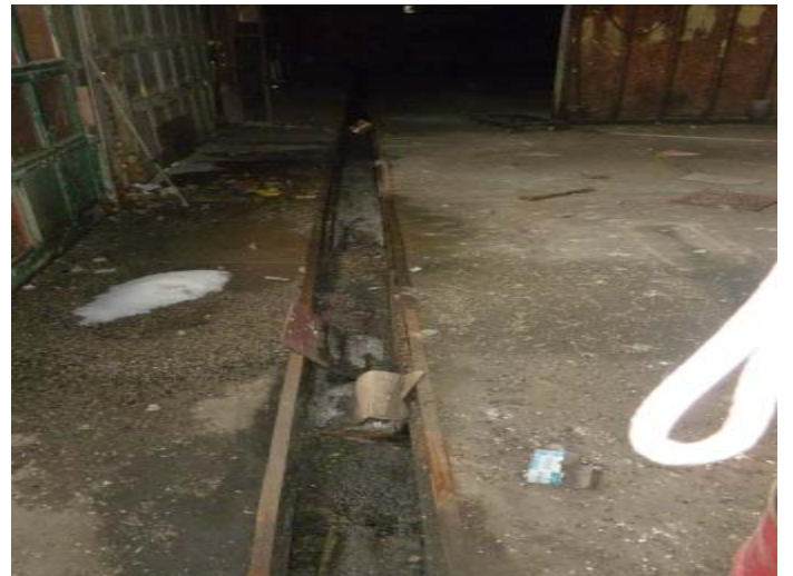
Former trench drain in shop area of Main Building.
