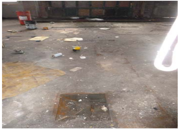
Former in-ground hydraulic lift in shop area of Main Building.
