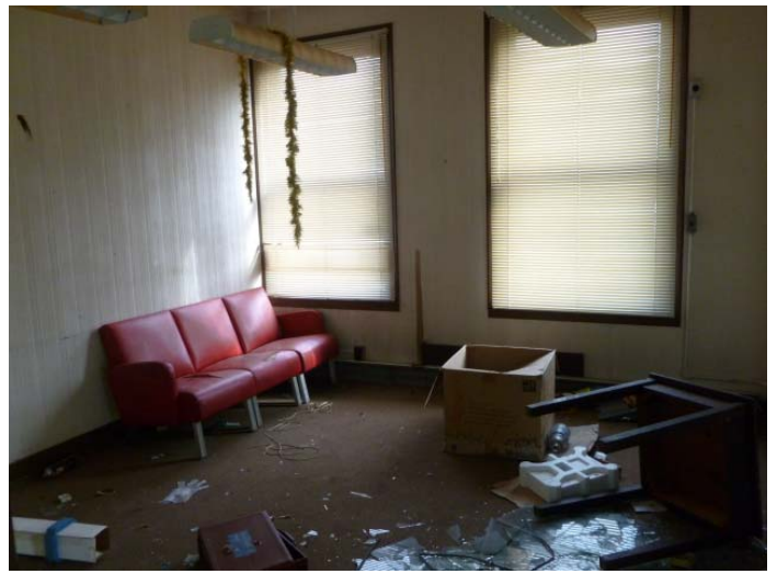
First floor former office area within Main Building.
