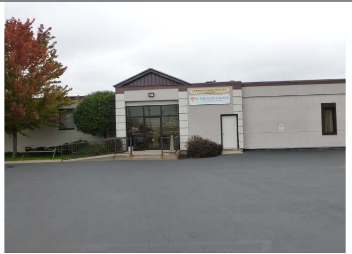
West adjacent property.
