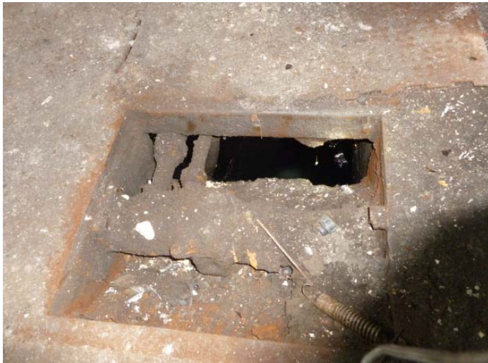
Former in-ground hydraulic lift in shop area of Main Building.
