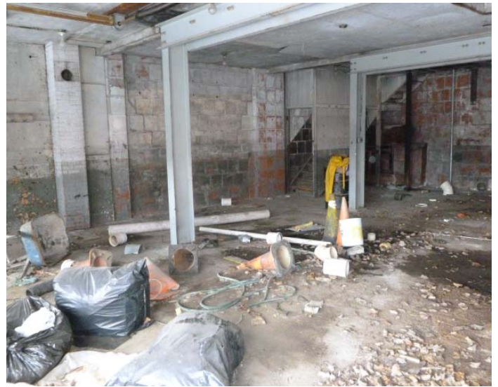
First floor interior of Vacant Garage.
