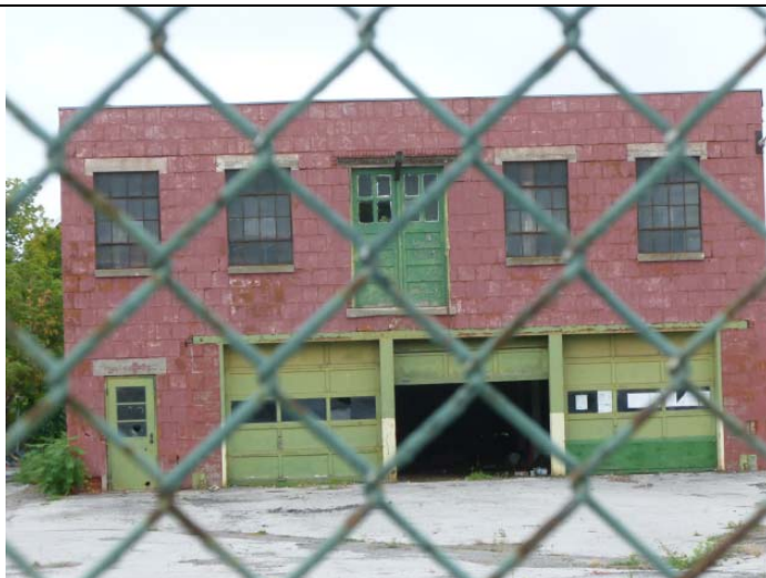
North side of the Vacant Garage.
