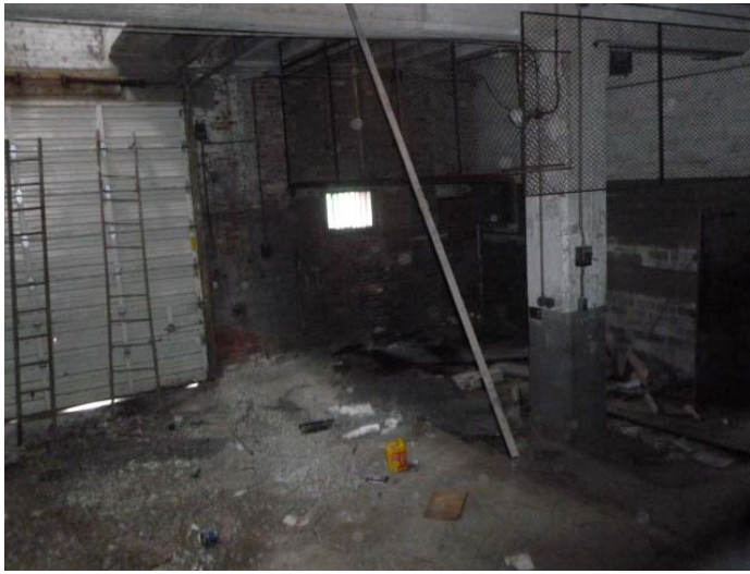
First floor in the rear portion of Main Building.
