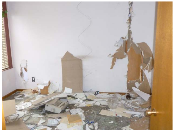
Second floor former office area in Main Building.
