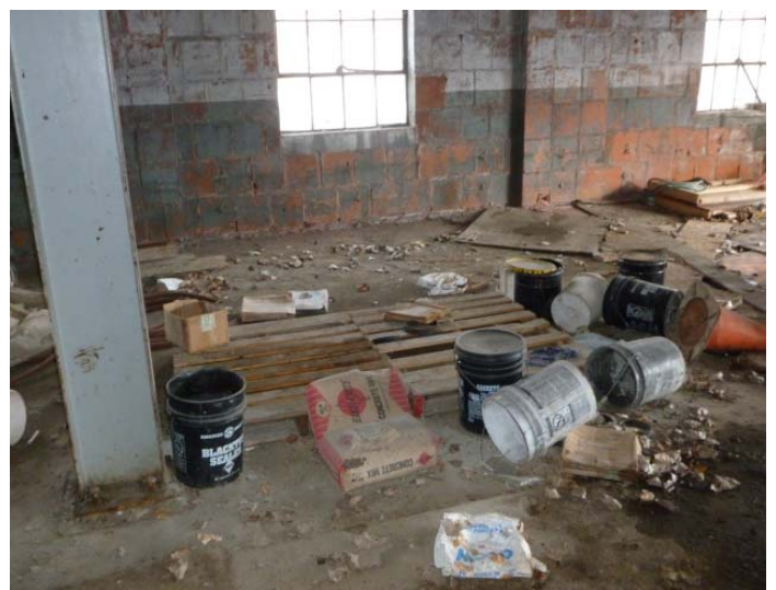
Buckets of blacktop sealer on first floor of Vacant Garage.
