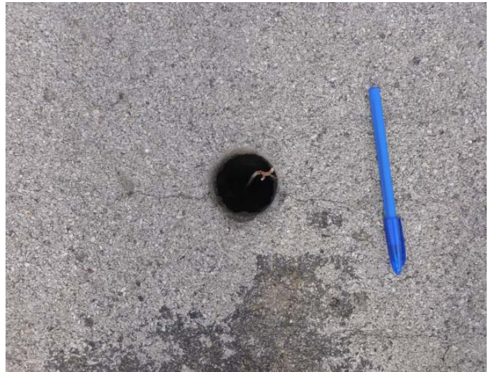
Former boring location east of Main Building.
