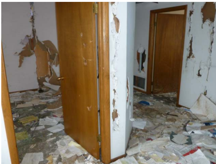
Second floor former office area in Main Building.
