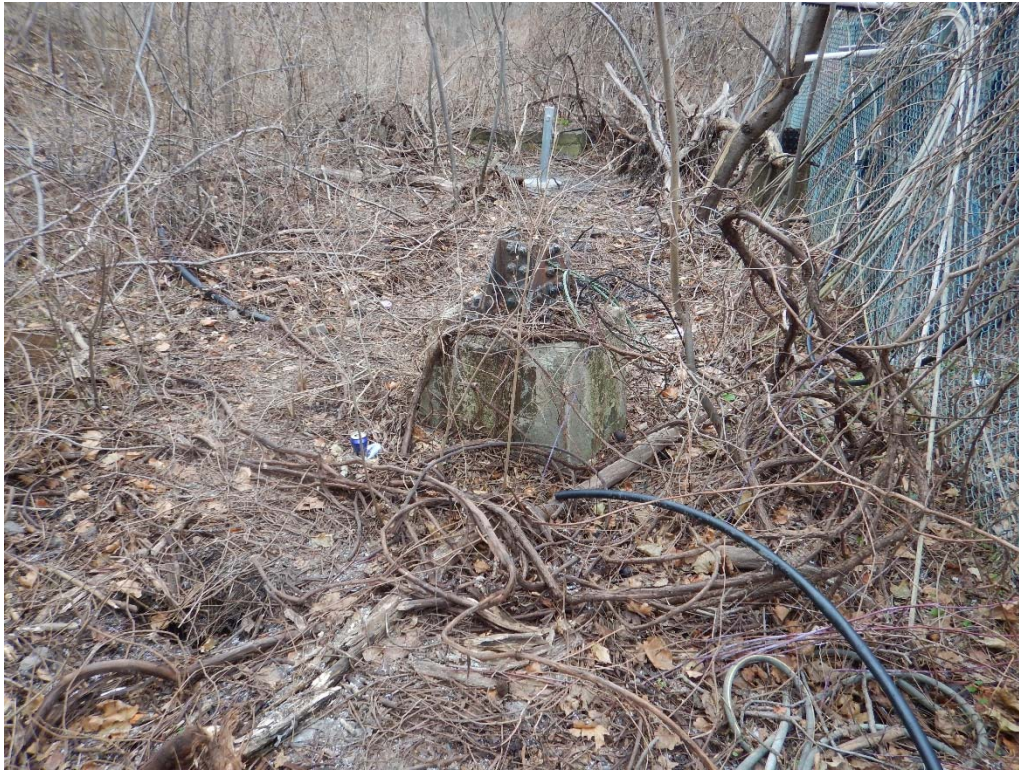
Photo 3. View northeast of a concrete piling located along the northeast side of the building. The piling is likely associated with the electric generating facility.
