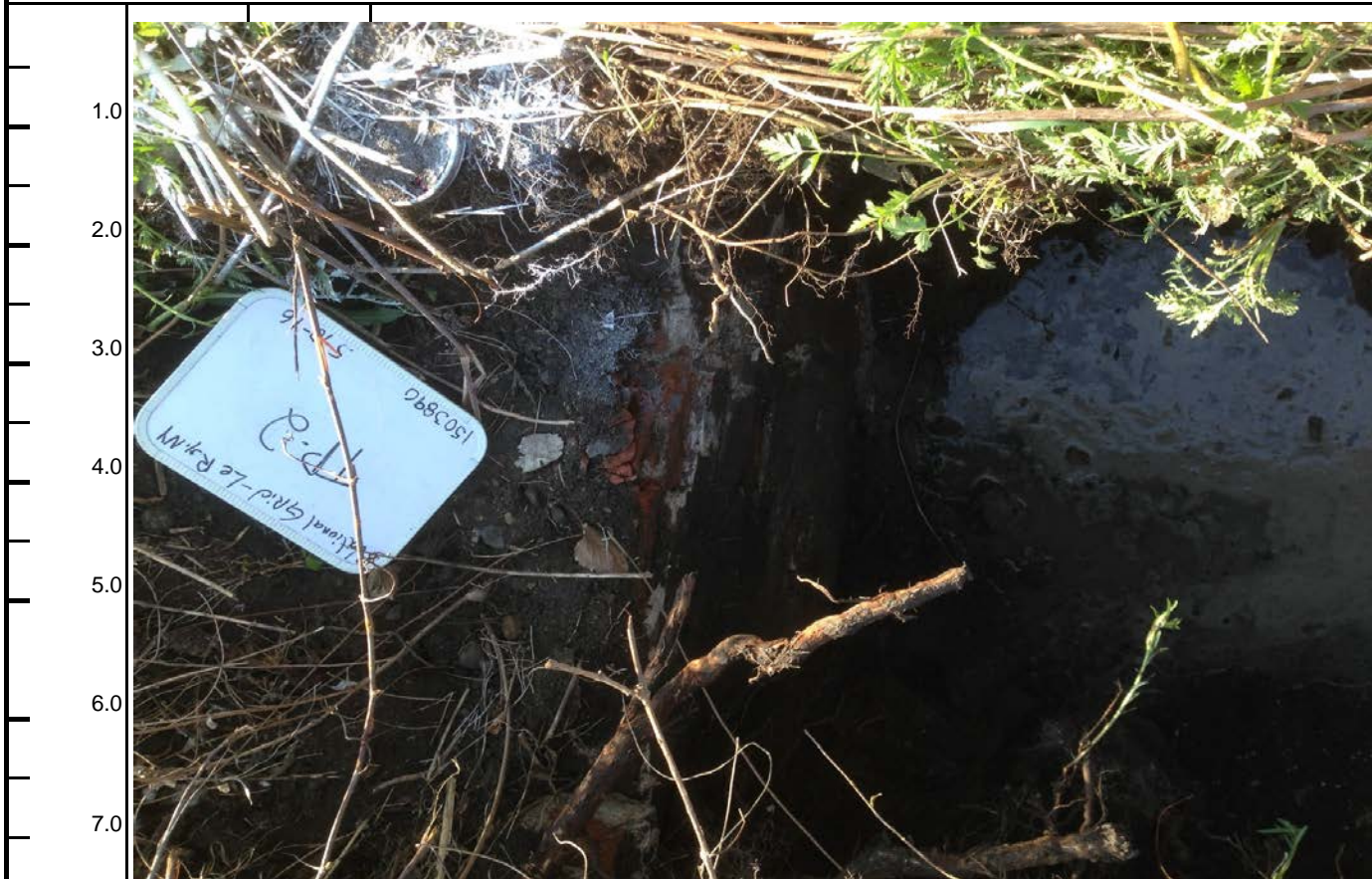
Caption: View to the southeast of the holder wall encountered in TP-2.
