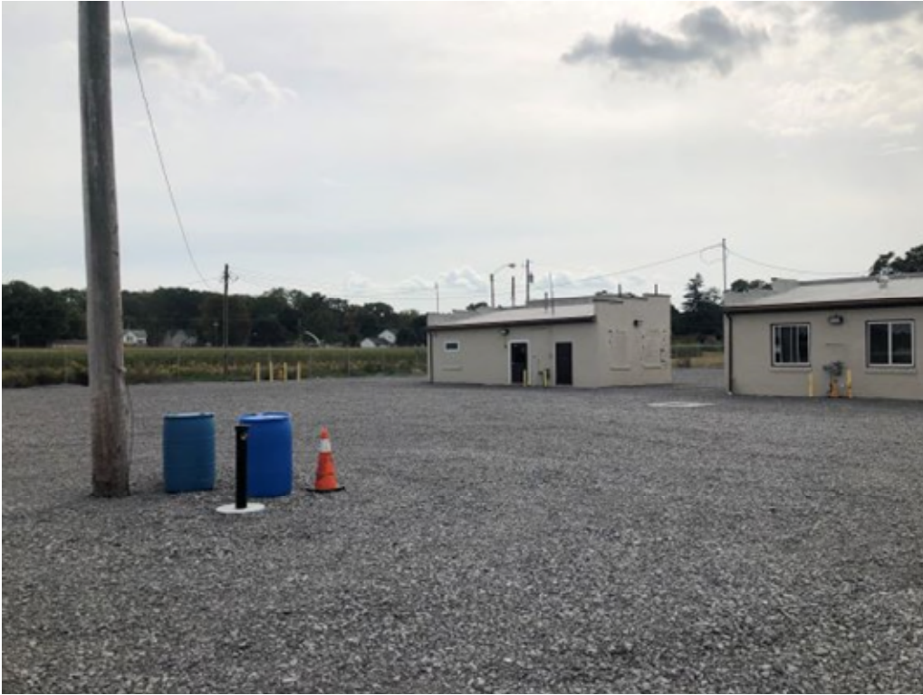
Locker Room Building, Eastern End of Office Building, and Plastic Drums Containing Purged Groundwater - Viewing Southeast
