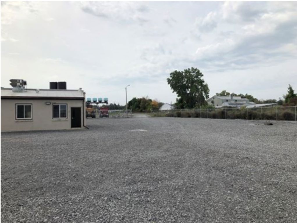
Western End of Office Building and Southwestern Portion of the Site - Viewing South
