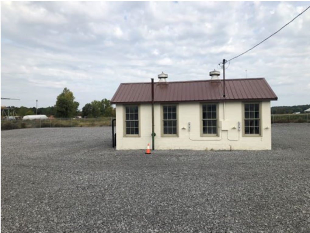
Gas Regulator Building and the Northern, Central Portion of the Site - Viewing North
