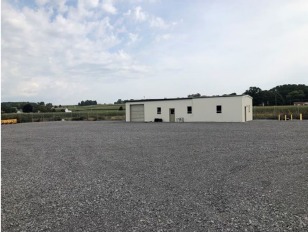
Training Building and the Northeastern Portion of the Site - Viewing Northeast
