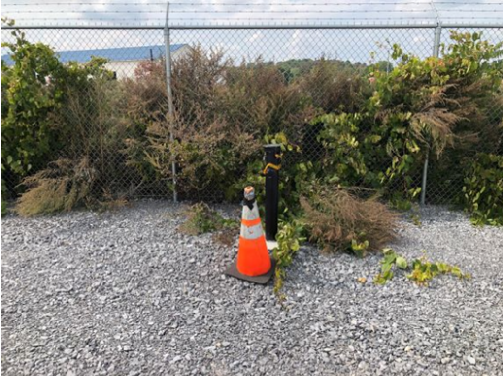
Typical “Stick Up” Groundwater Monitoring Well at the Site
