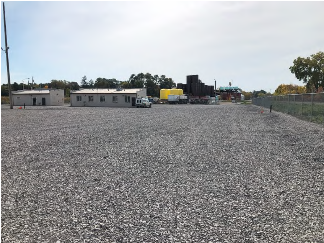
Office Building and Western Portion of the Site - Viewing South
