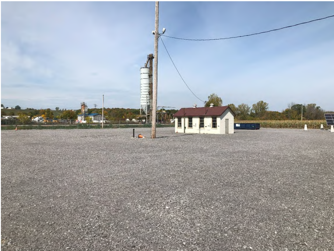
Gas Regulator Building and the Central Portion of the Site - Viewing Northwest
