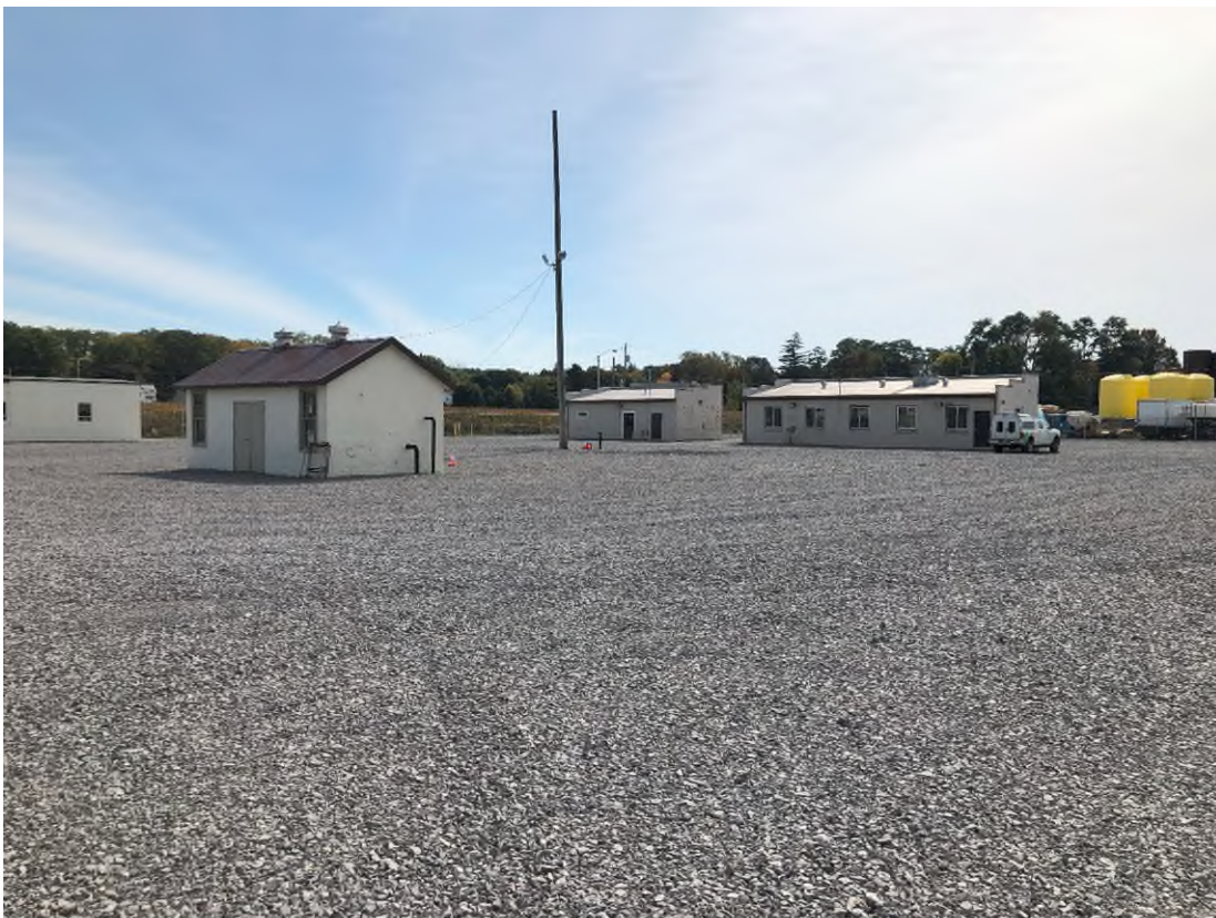
Gas Regulator Building and the Central Portion of the Site - Viewing Southeast
