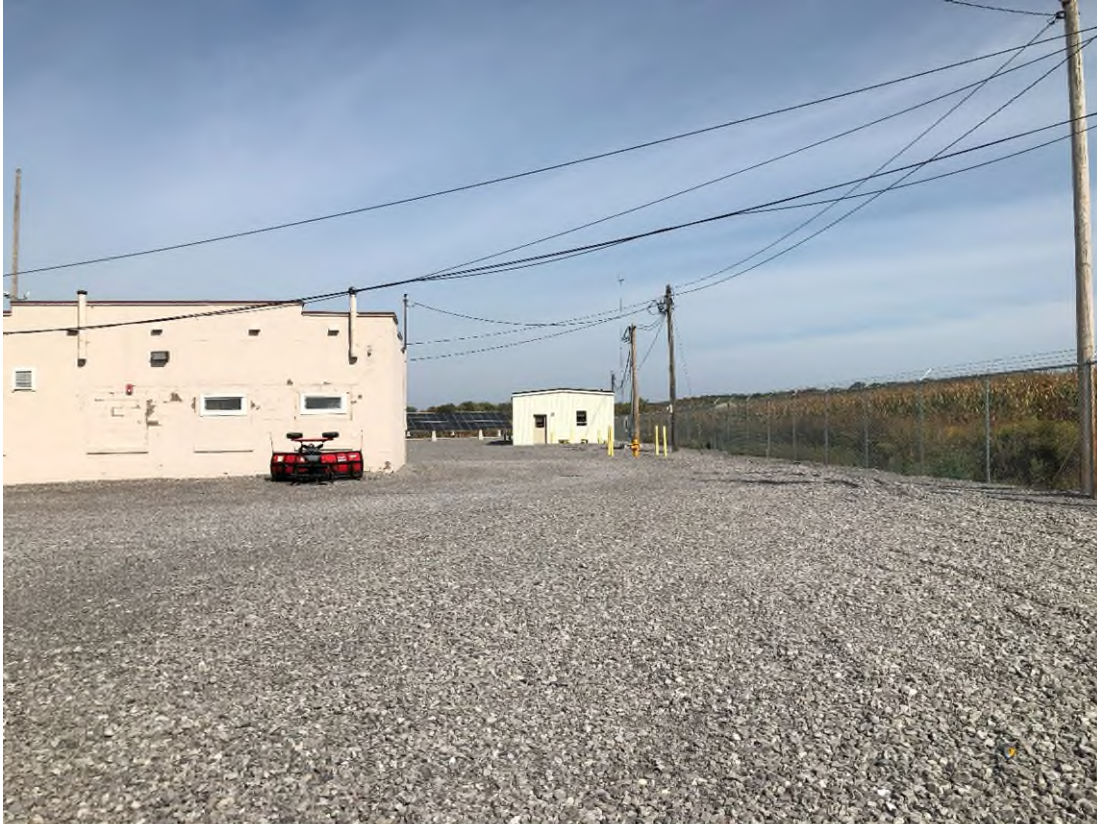
Eastern Portion of the Site – Viewing North
