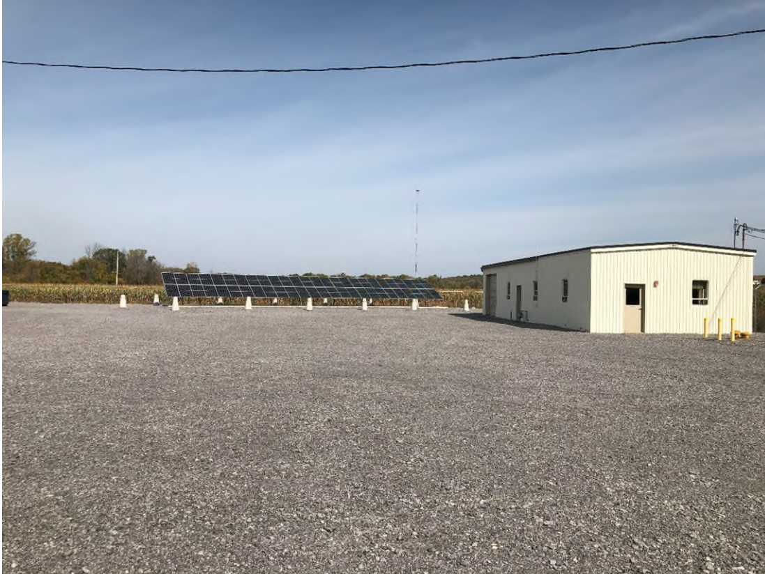
Training Building and Solar Panels on the Northeastern Portion of the Site - Viewing North
