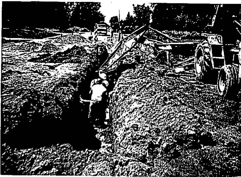
Photo 16- North Bloomfield, N.Y. 7/29/87. Gas service line encountered along Martin Road.
