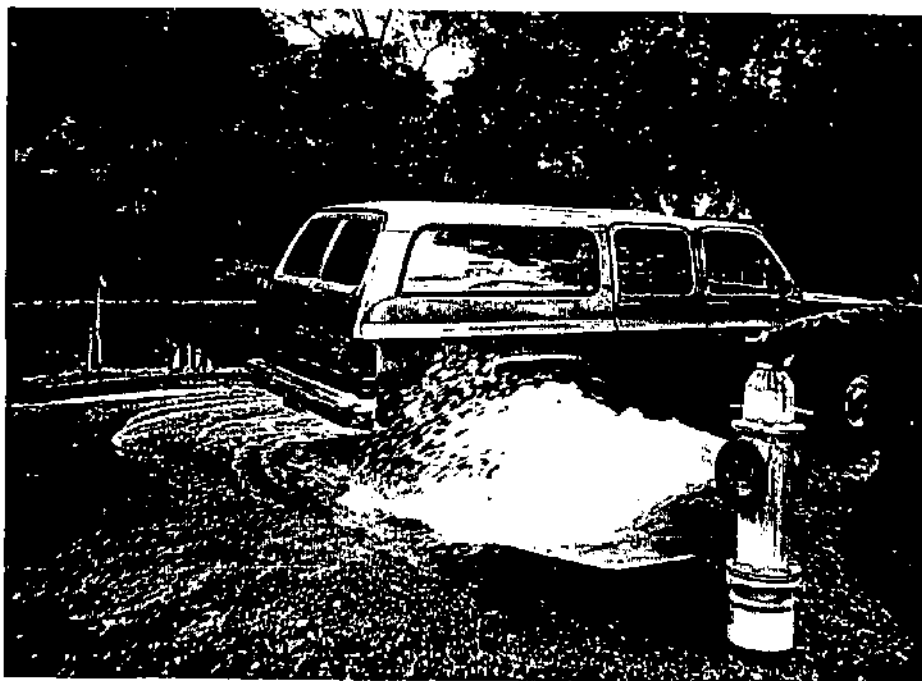
Photo 26- North Bloomfield, N.Y. 9/23/87. A water main is being flushed until clear water is visible.
