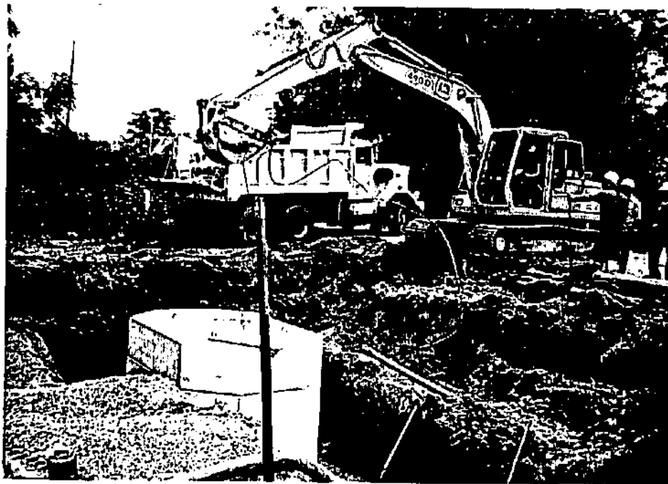
Photo 5 - North Bloomfield, N.Y. 7/16/87. A concrete meter vault in place at Martin Road.
