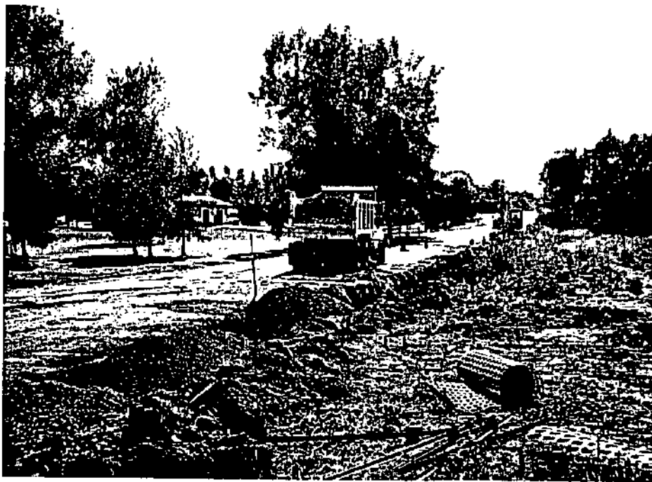
Photo 12- North Bloomfield, N.Y. 7/21.87. Backfilling operation along Martin Road.
