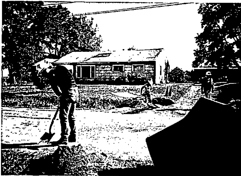
Photo 40- North Bloomfield, N.Y. 9/4/87. A copper service pipe installed underneath the road at two ends. One end being where the man in the foreground is holding a shovel. The other end being where the man is compacting soil with a hand-tamper.
