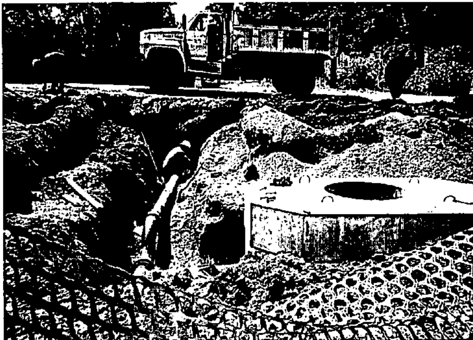
Photo 10- North Bloomfield, N.Y: 7/16/87. The RWW crew installing water main along Martin Road in the westerly direction.
