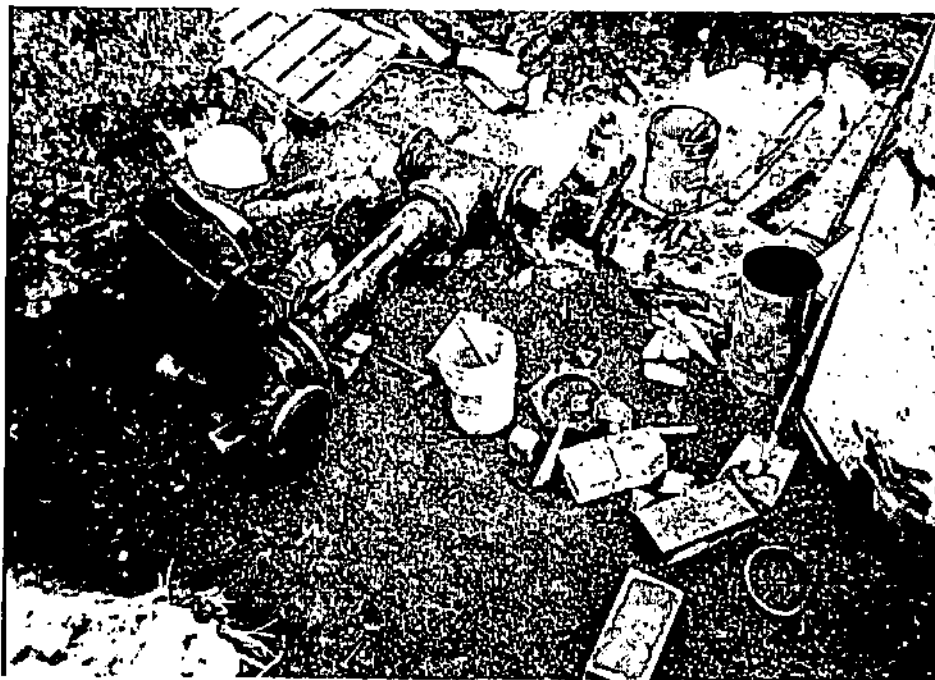
Photo 6 - North Bloomfield, N.Y. 1/12/88. By-pass connection is being made at the meter vault on Ontario Street.
