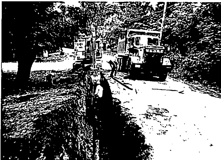
Photo 20- North Bloomfield, N.Y. 9/17/87. Rocking cutting operation along Martin Road.
