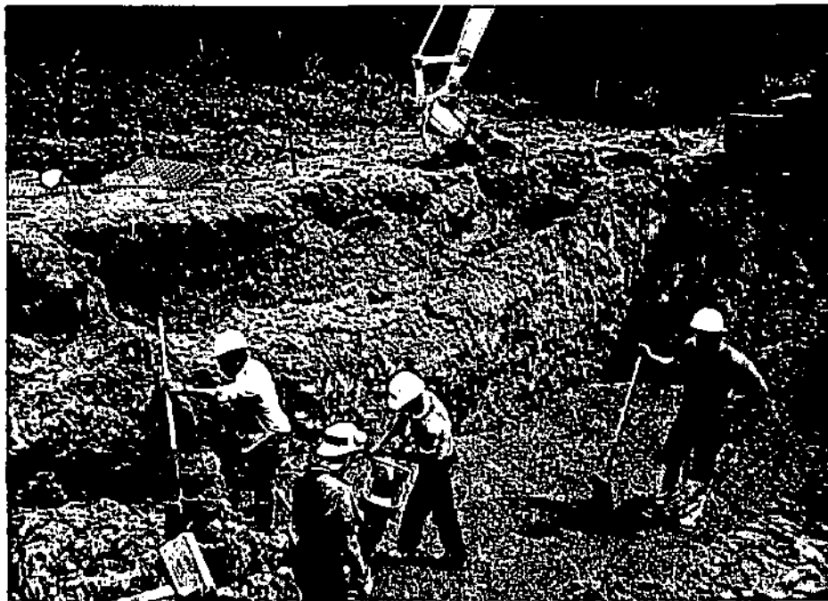
Photo 2 - North Bloomfield, N.Y. 7/16/87. Preparation of the subgrade for meter vault installation.
