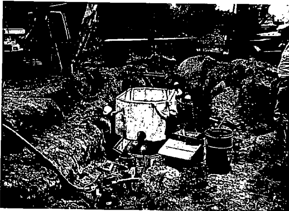
Photo 4 - North Bloomfield, N.Y. 7/16/87. The middle section of the meter vault is being placed.
