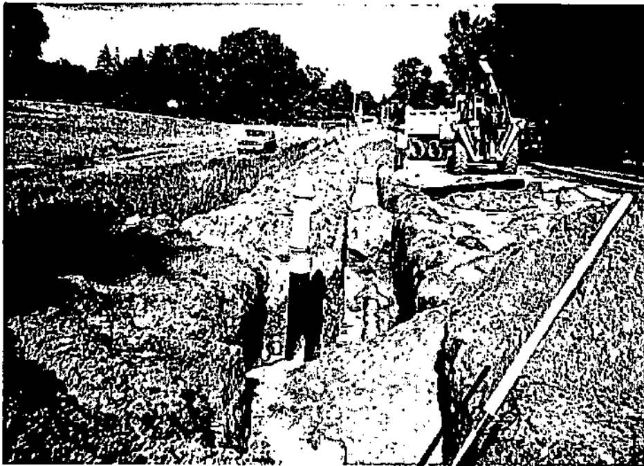
Photo 15- North Bloomfield, N.Y. 7/22/87. Overall view of installed fire hydrant, backfilling of the trench, and groundwater appearance.
