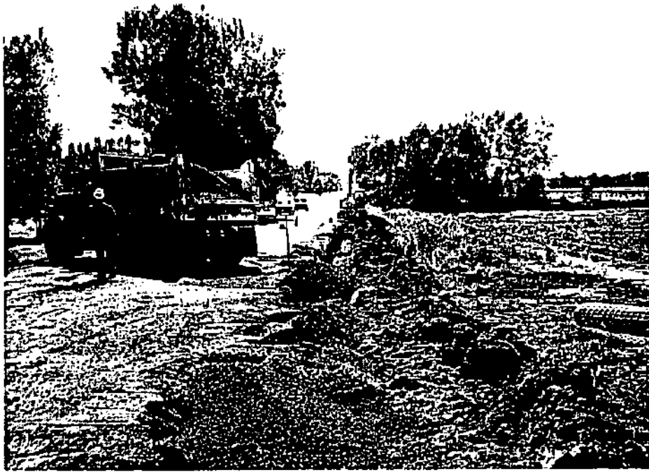
Photo 13- North Bloomfield, N.Y. 7/21/87. Backfilling of the trench in the westerly direction along Martin Road.
