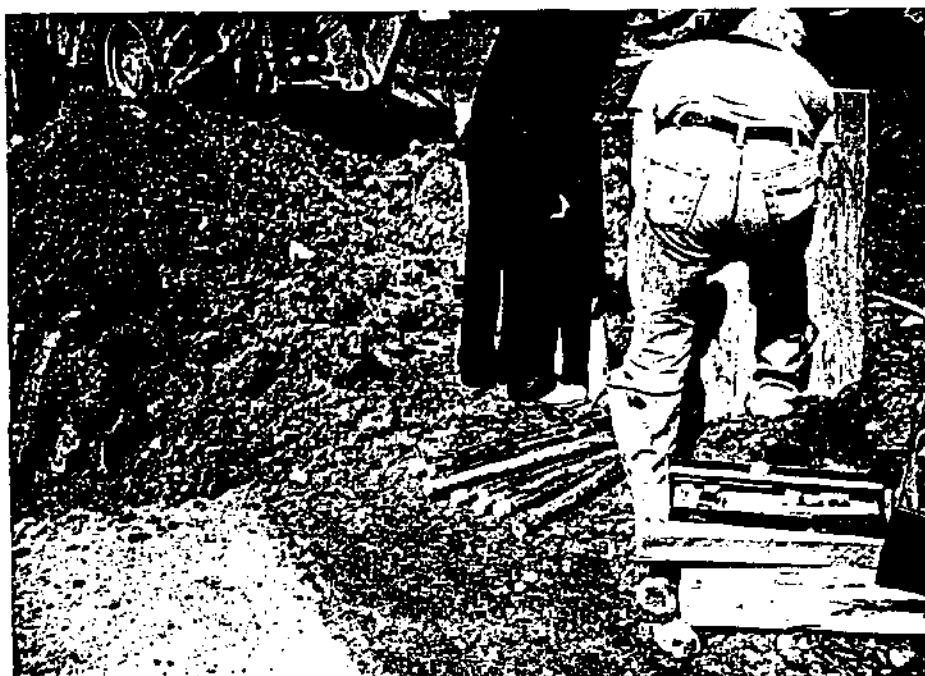
Photo 32- North Bloomfield, N.Y. 9/4/87. Rod used in conjunction with the Hole-hog equipment to push through the soil for copper pipe placement.
