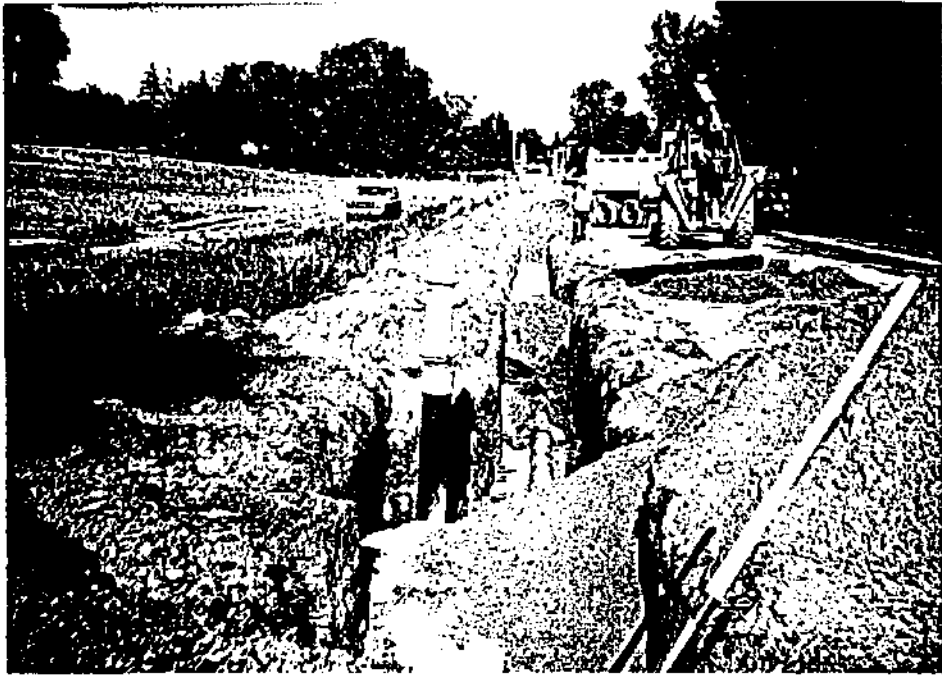
Photo 15- North Bloomfield, N.Y. 7/22/87. Overall view of installed fire hydrant, backfilling of the trench, and groundwater appearance.
