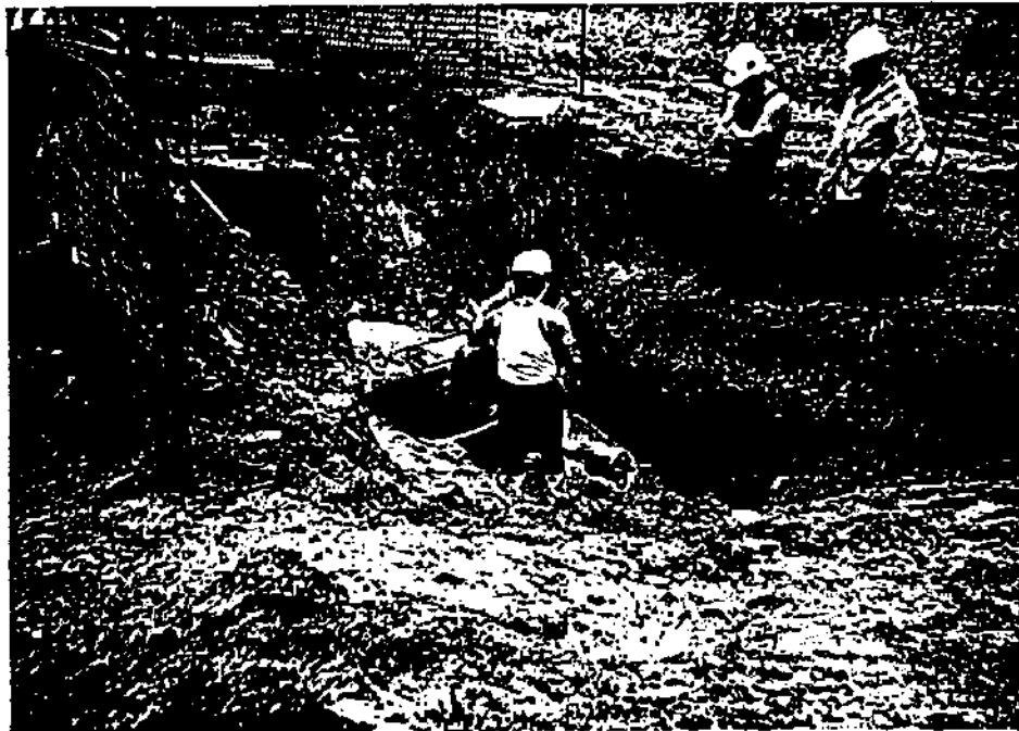
Photo 1 - North Bloomfield, N.Y. 7/14/87. The Rochester Water Works (RWW) crew tapping into the existing water main.
