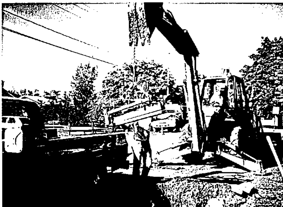
Photo 31- North Bloomfield, N.Y. 9/4/87. Hole-hog equipment being lowered into the trench.
