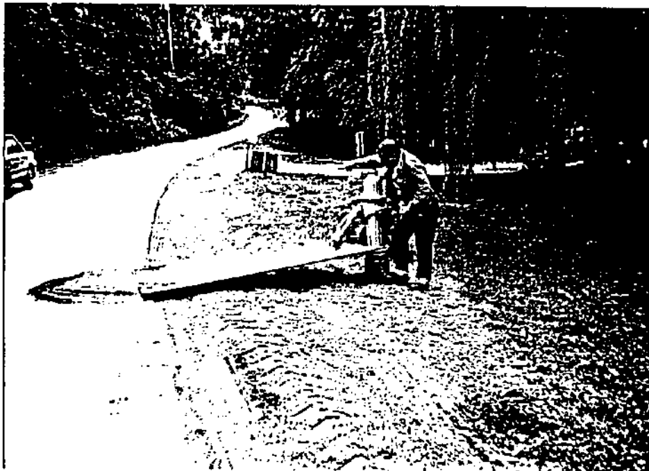
Photo 24- North Bloomfield, N.Y. 9/23/87. A hydrant valve is being opened to flush the water main.
