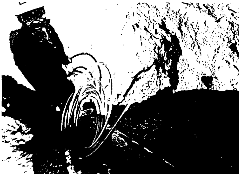
Photo 38- North Bloomfield, N.Y. 9/4/87. A copper service pipe being pushed along with the rods and rods are removed one by one at other end of the hole created by the Hole-hog device.
