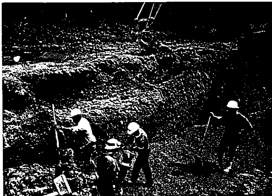
Photo 2 - North Bloomfield, N.Y. 7/16/87. Preparation of the subgrade for meter vault installation.
