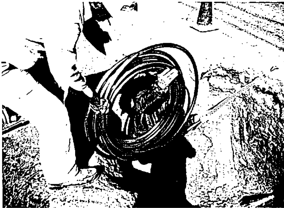
Photo 37- North Bloomfield, N.Y. 9/4/87. A copper service pipe being attached to the rod to be fed into the hole pushed through the soil by the Hole-hog.
