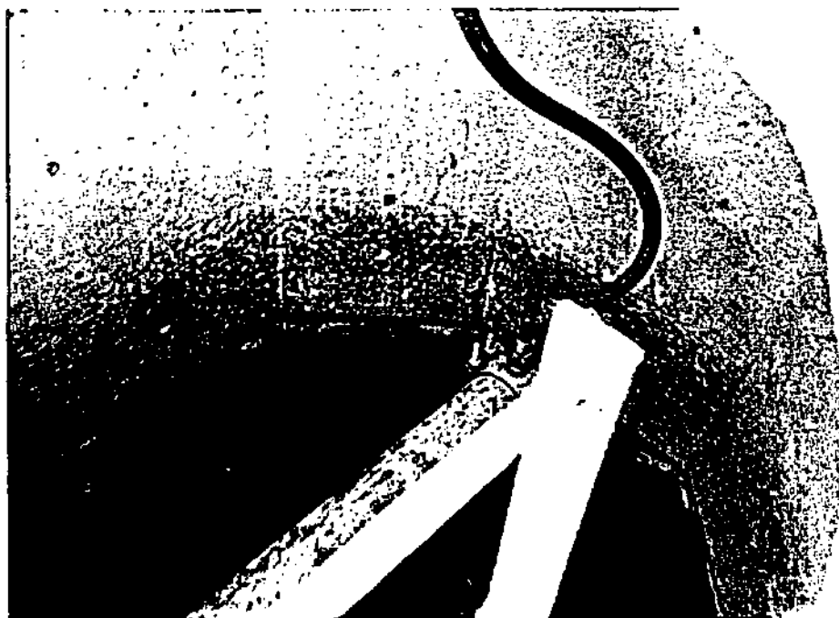
Photo 27- North Bloomfield, N.Y. 9/24/87. Connections inside the meter vault for the pressure testing operation.
