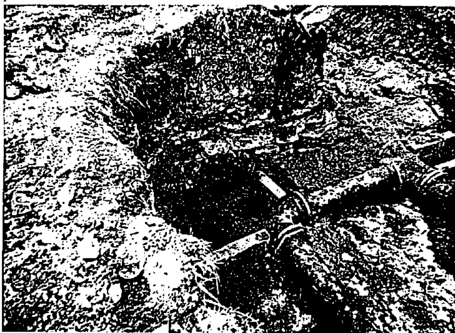
Photo 7 - North Bloomfield, N.Y. 1/12/88. Concrete thrust blocks are being placed at the by-pass connection system.
