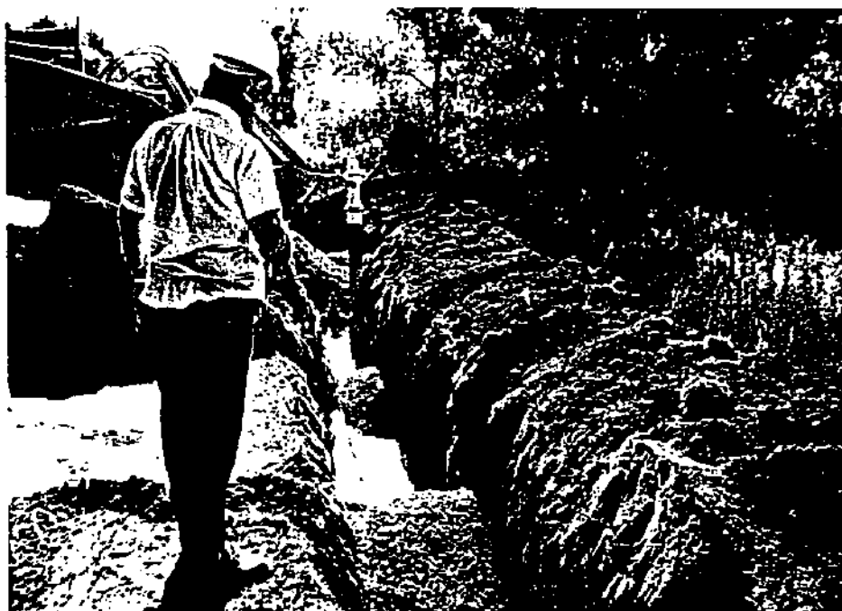
Photo 14- North Bloomfield, N.Y. 7/22/87. Installed fire hydrant on Martin Road. Note the appearance of groundwater in the trench.
