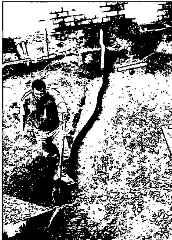
T-2 Horizontal piping installation
