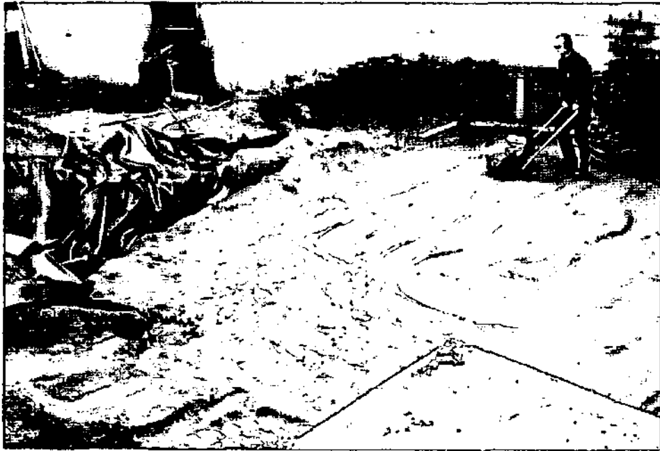
Compaction of sand layer over Geo-membrane
