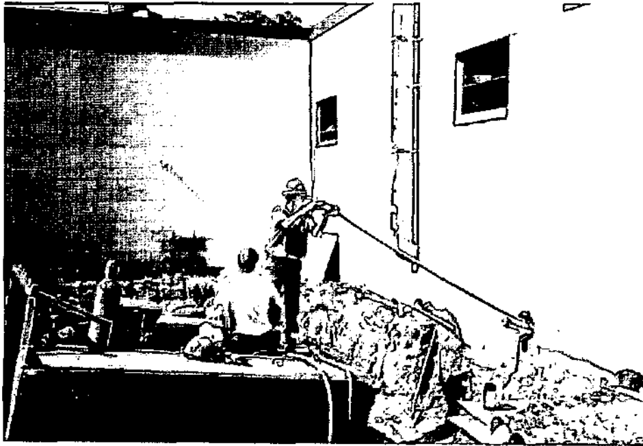
Placement of sand into tremie pipe for secondary sand pack
