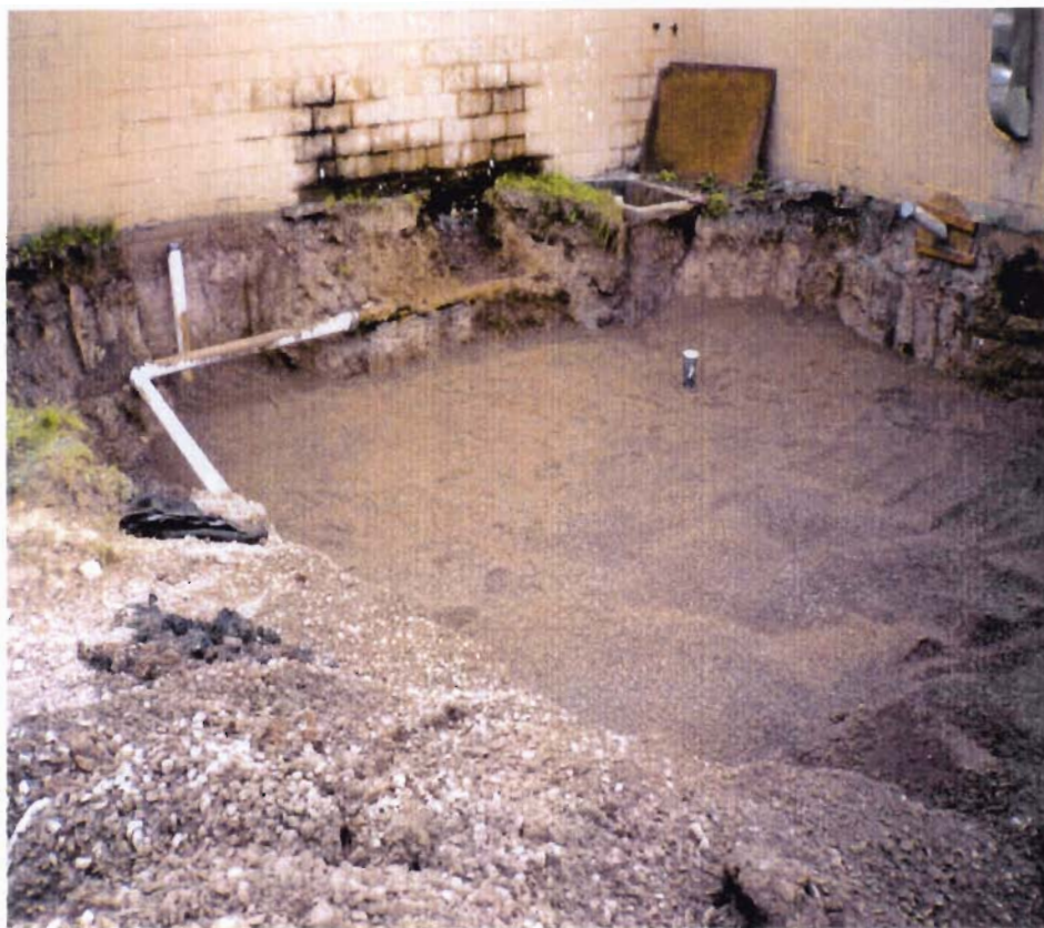
Pea stone Placement NOTE: Repaired SPDES out-fall piping
