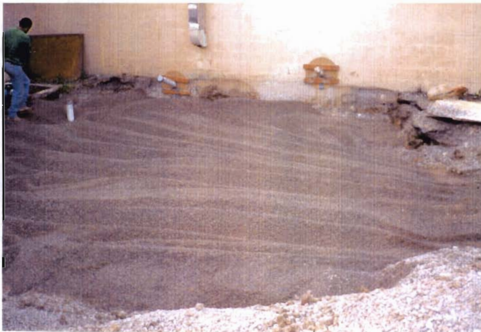
Placement of peastone layer over compacted sand
