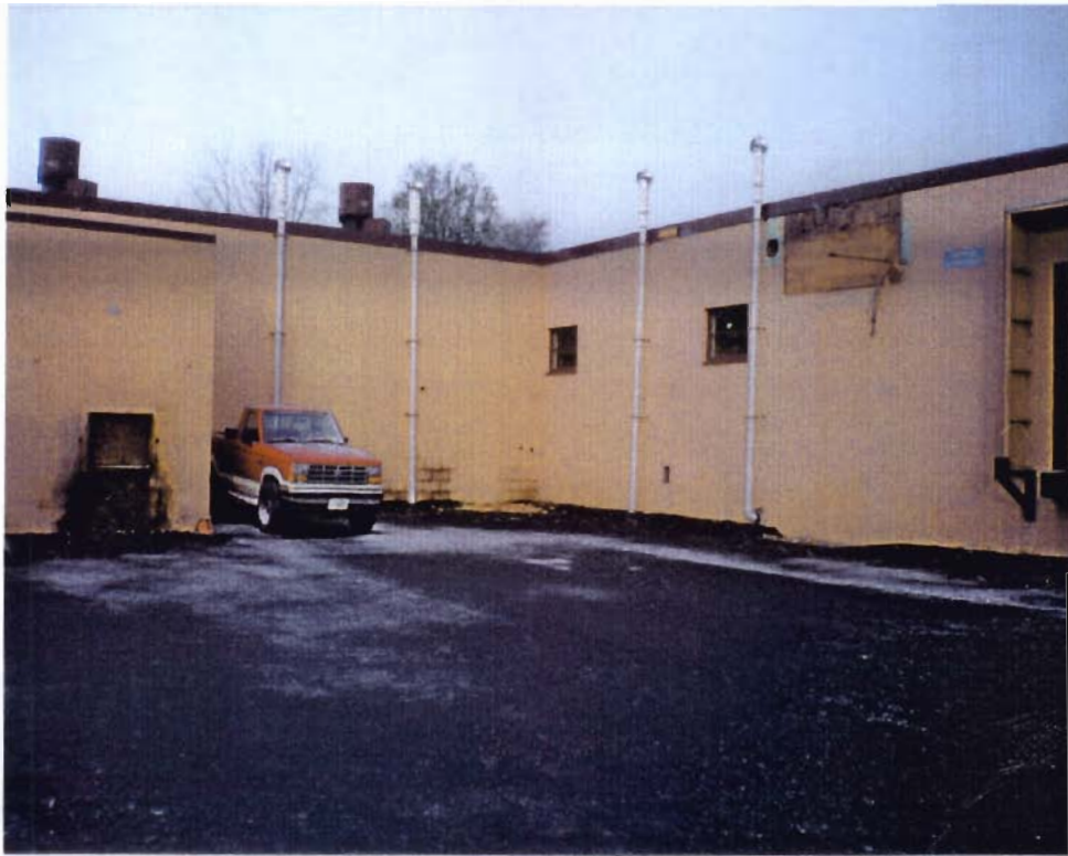
Excavation area following asphalt placement
