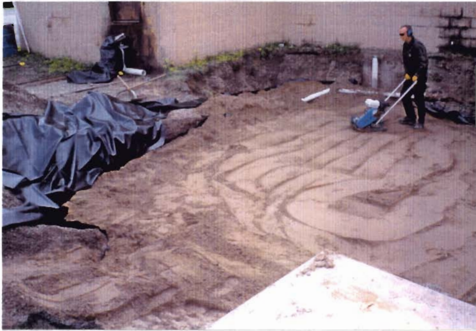
Compaction of sand layer over Geo-membrane
