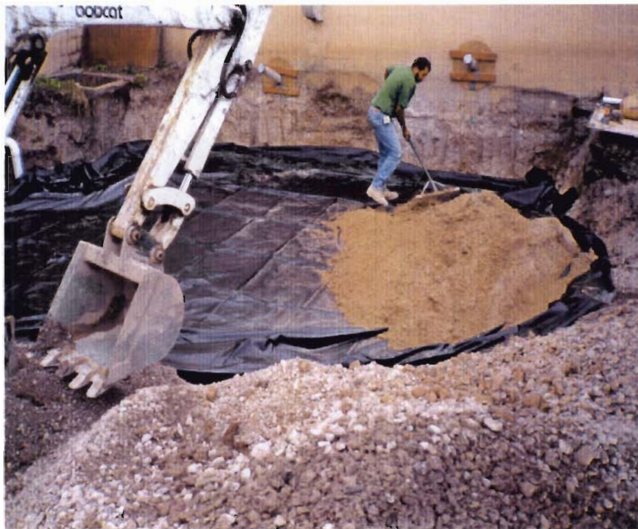
Northwest Geo-liner and Sand Placement
