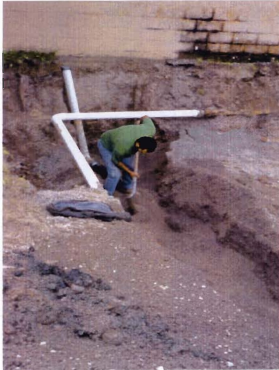
T-1 Horizontal piping installation
