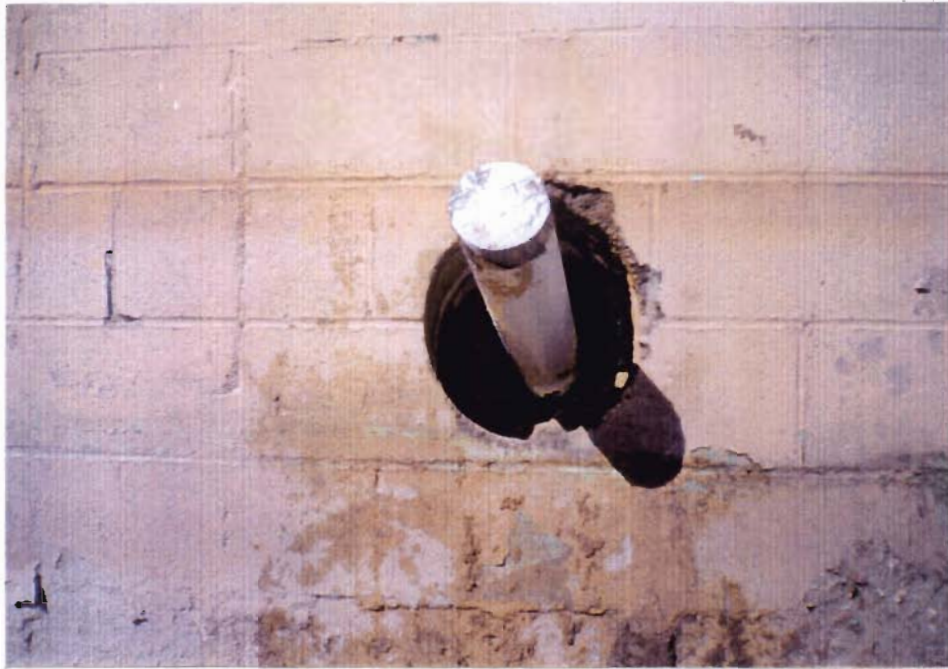
Well prior to surface seal placement
