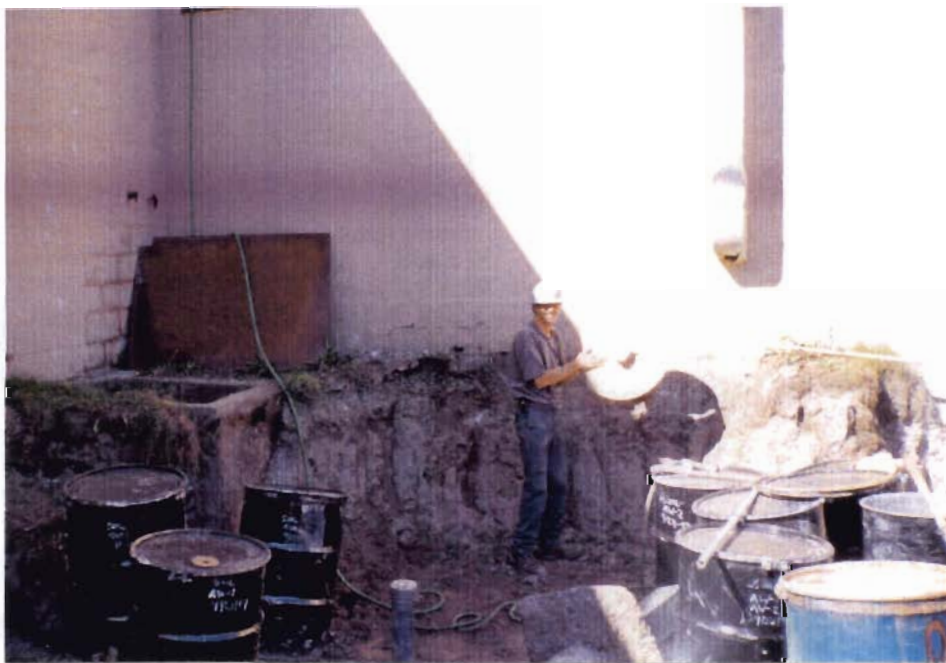
Placement of concrete form for surface seal placement
