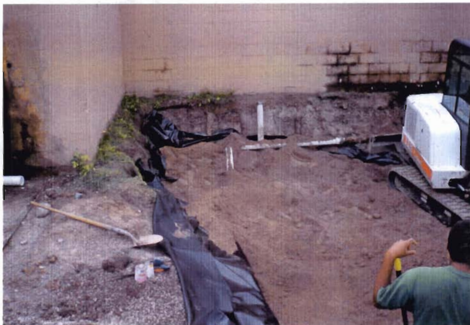
South west Geo-liner and Sand Placement
