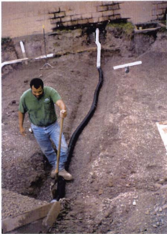
T-2 Horizontal piping installation
