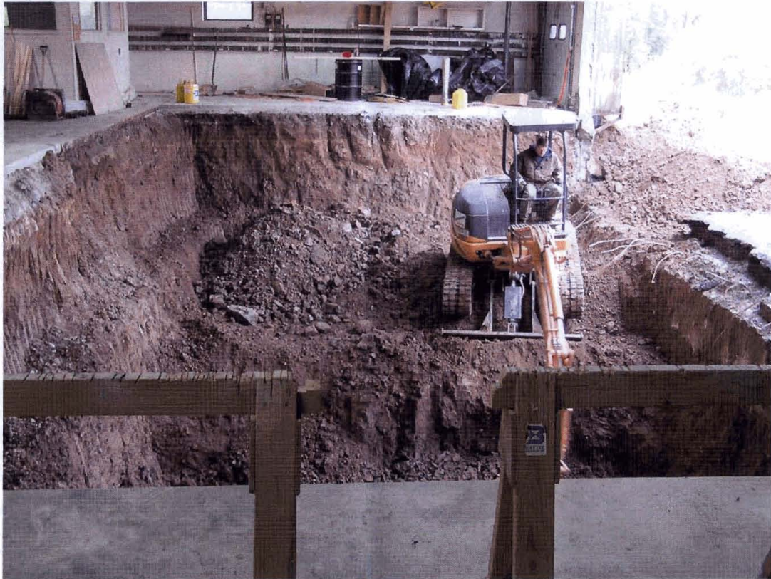
Photo #7. Deeper soil removal along west side of excavation, moving east.
