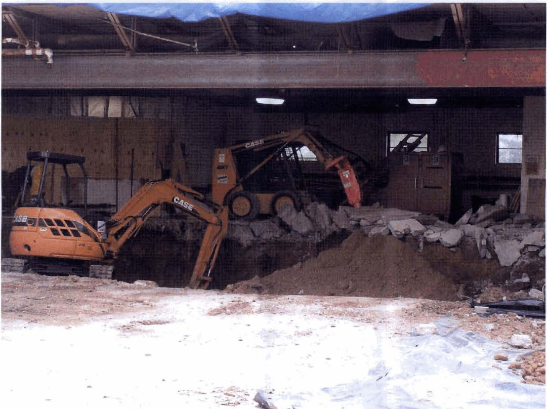
Photo #4. Soil removal activities in central area of the excavation.
