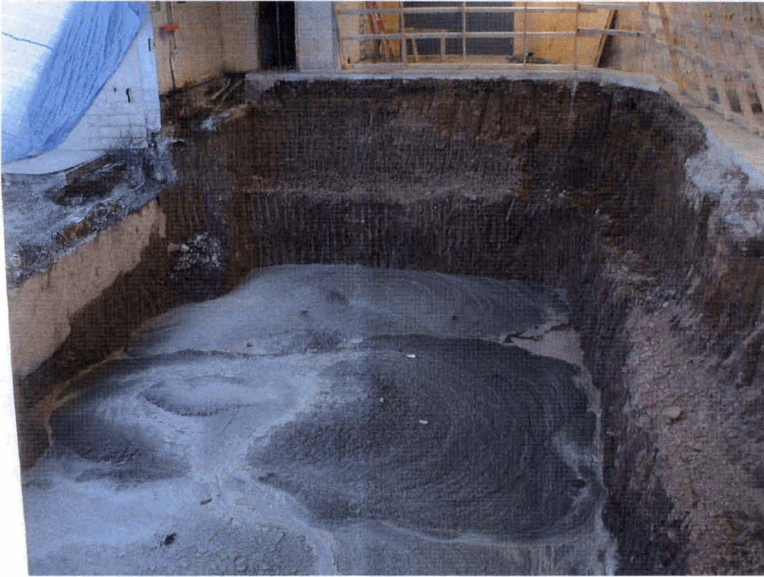
Photo# 9. Backfilling excavation with flowable concrete fill.
