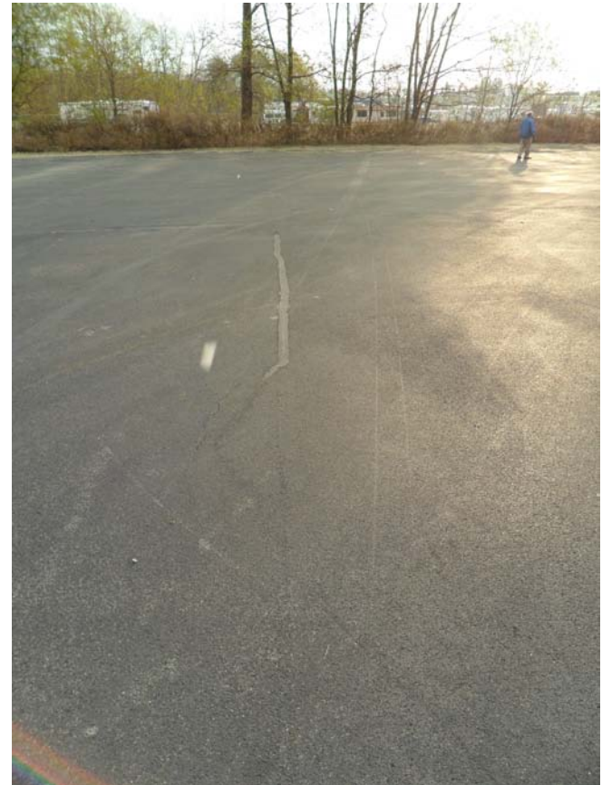
Crack filling repairs
