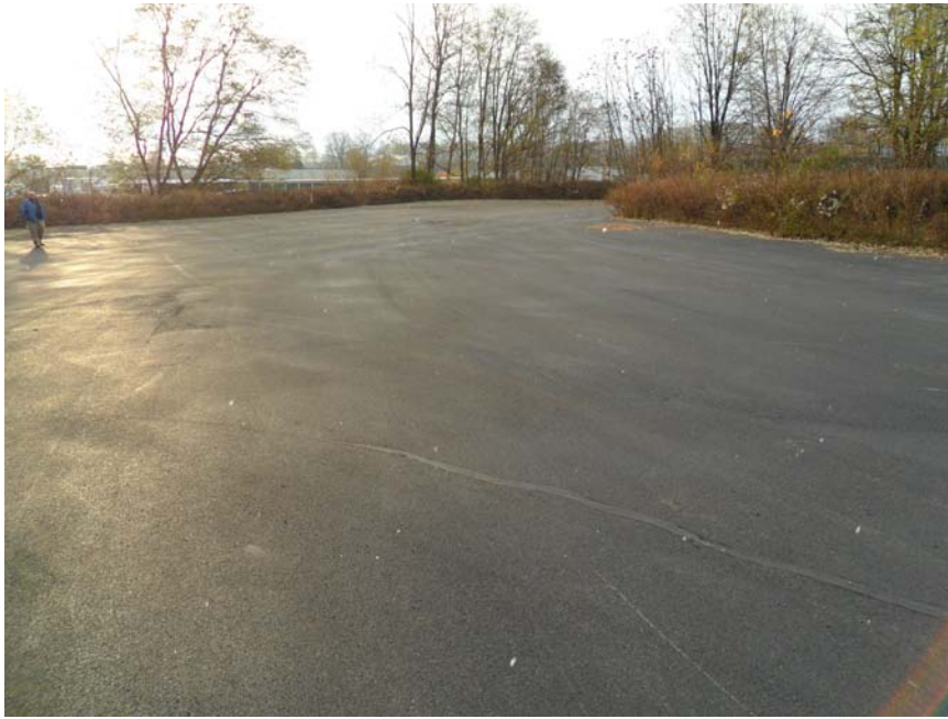
Crack filling repairs
