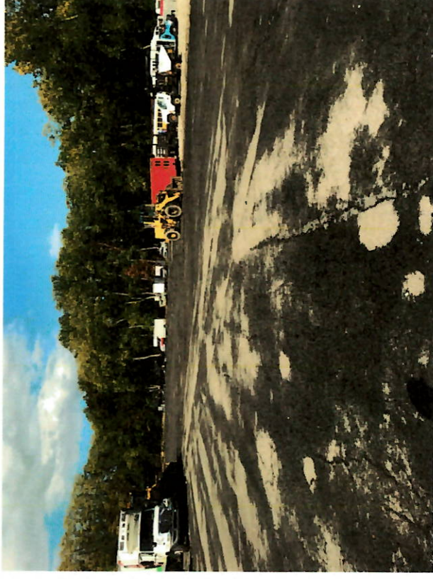
Photo 10: Some surficial cracking observed along pass lines
