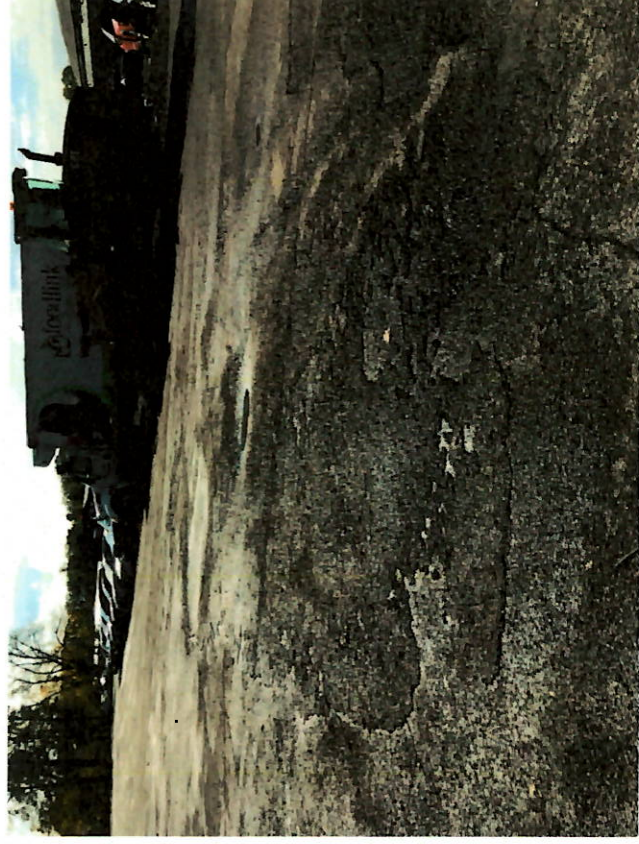
Photo 8: Cracking and spalling of surface. Deep settling observed in two areas.
