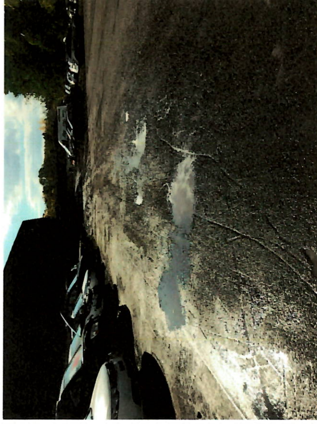
Photo 2: Surficial cracking, pooling of water on asphalt cover
