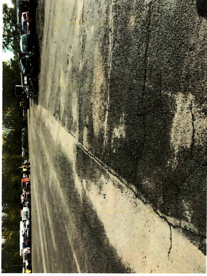
Photo 6: Surficial cracking observed along paving pass lines
