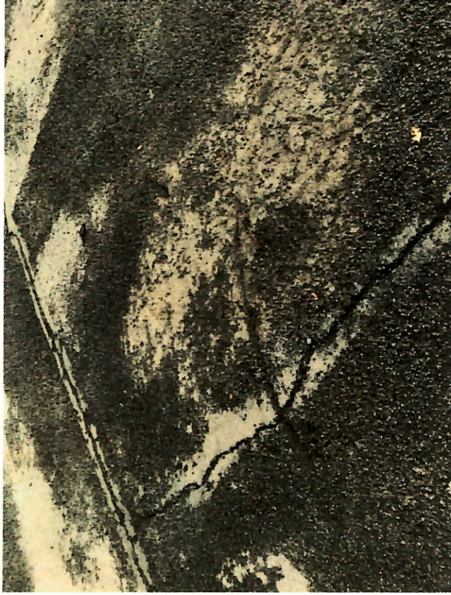
Photo 7: Close up of surficial cracking
