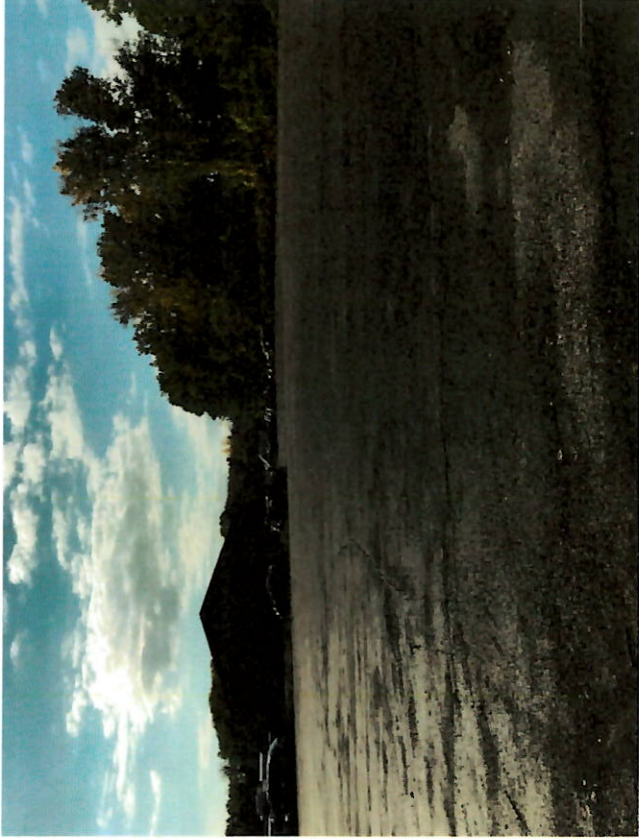
Photo 3: Surficial cracking throughout asphalt cap
