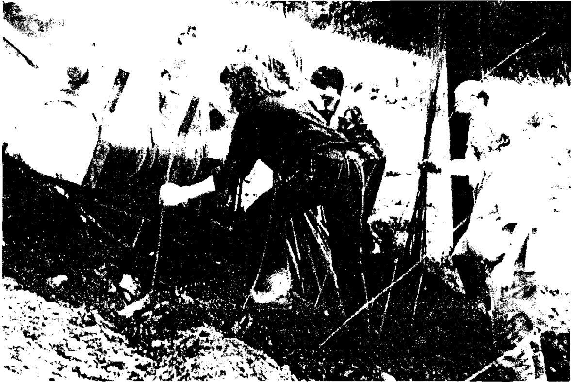
Figure 2: Planting 5 ft tall hybrid poplar whips into 4 ft of soil covering construction debris waste, Lakeside Reclamation Landfill, Beaverton, Oregon (1990).
