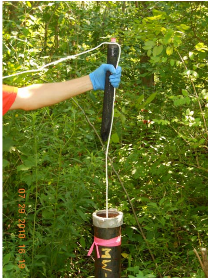
Photo #17: July 29, 2010 – PDB install at MW-13.
