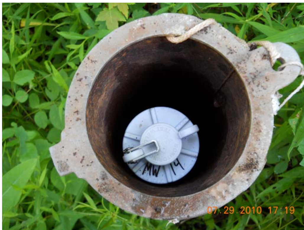
Photo #24: July 29, 2010 – PDB install complete at MW-14.
