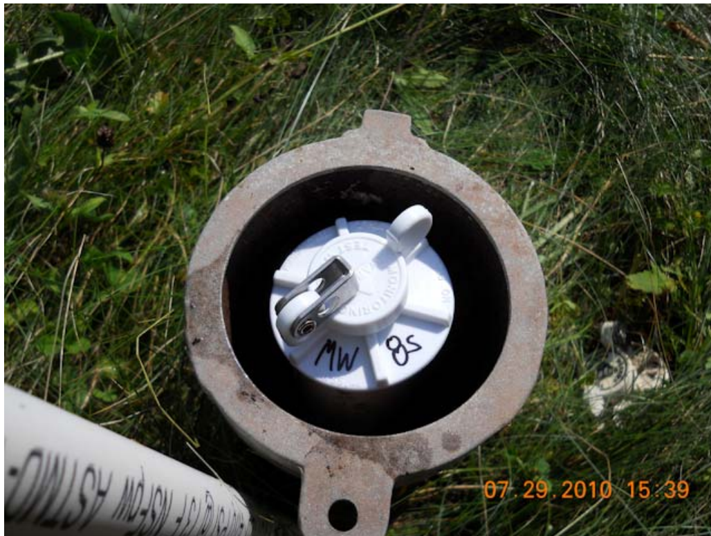
Photo #14: July 29, 2010 – PDB install complete at MW-8s.
