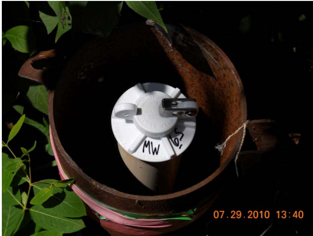
Photo #15: July 29, 2010 – PDB install complete at MW-6s.
