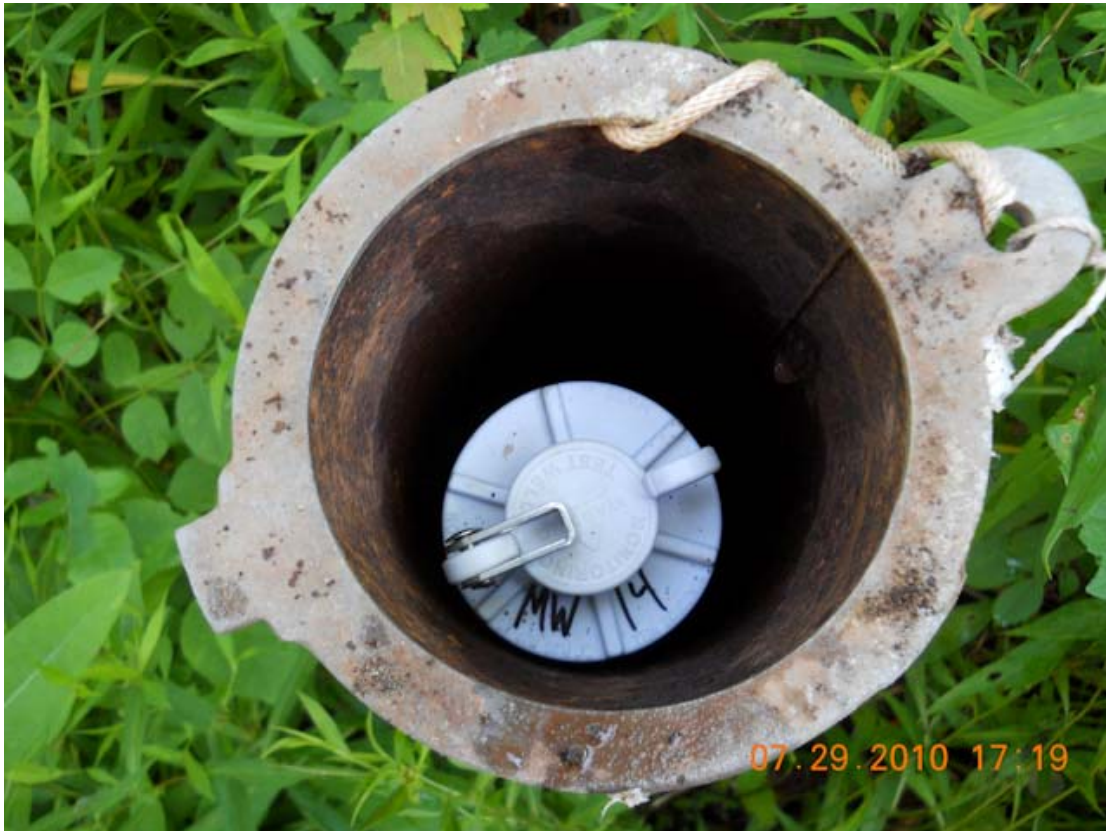
Photo #33: July 29, 2010 – PDB install complete at MW-14.
