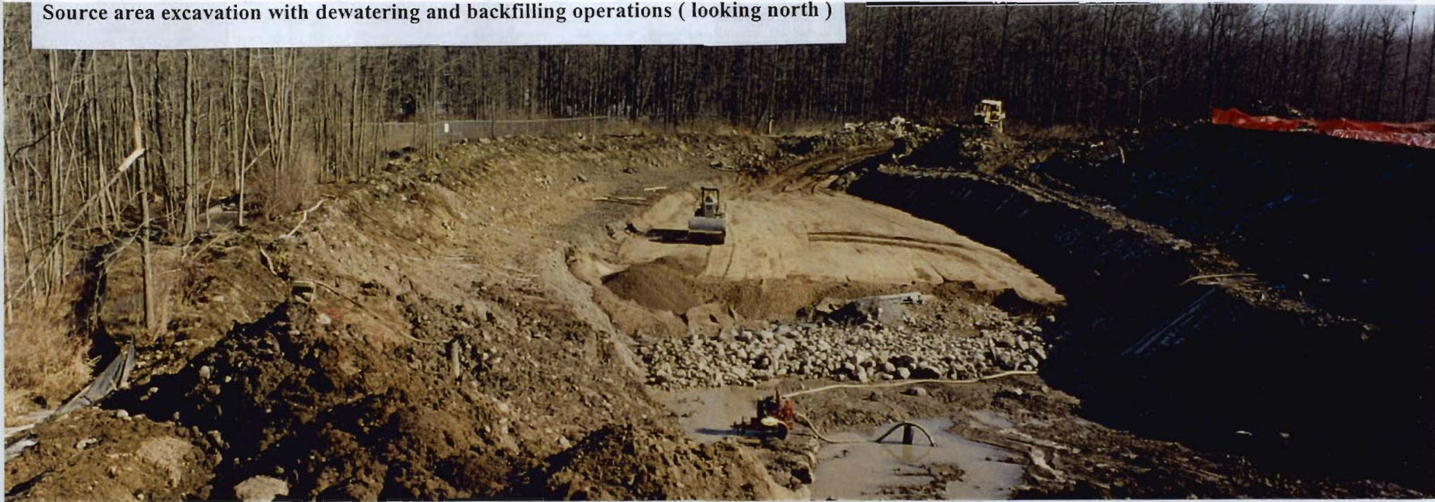
Source area backfilling operations and HDPE sump ( looking north )
