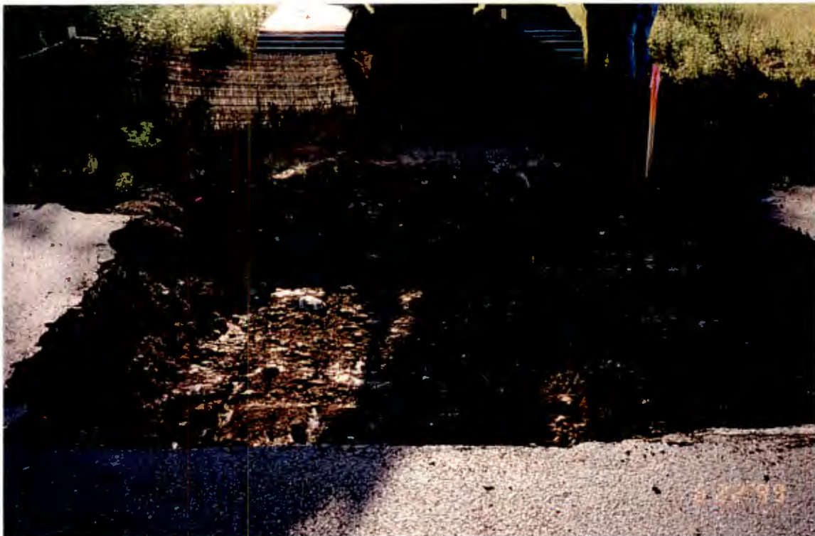
Photograph #8: Excavation of source area BL-11D in progress.
