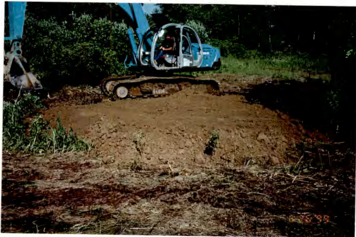
Photograph #4: Restoration of source area BL-16S.
