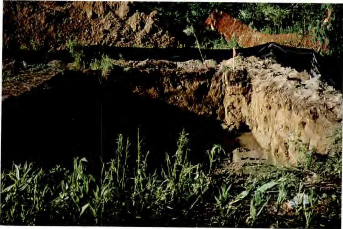
Photograph #5: Excavation of source area BL-9S in progress (Section 1).
