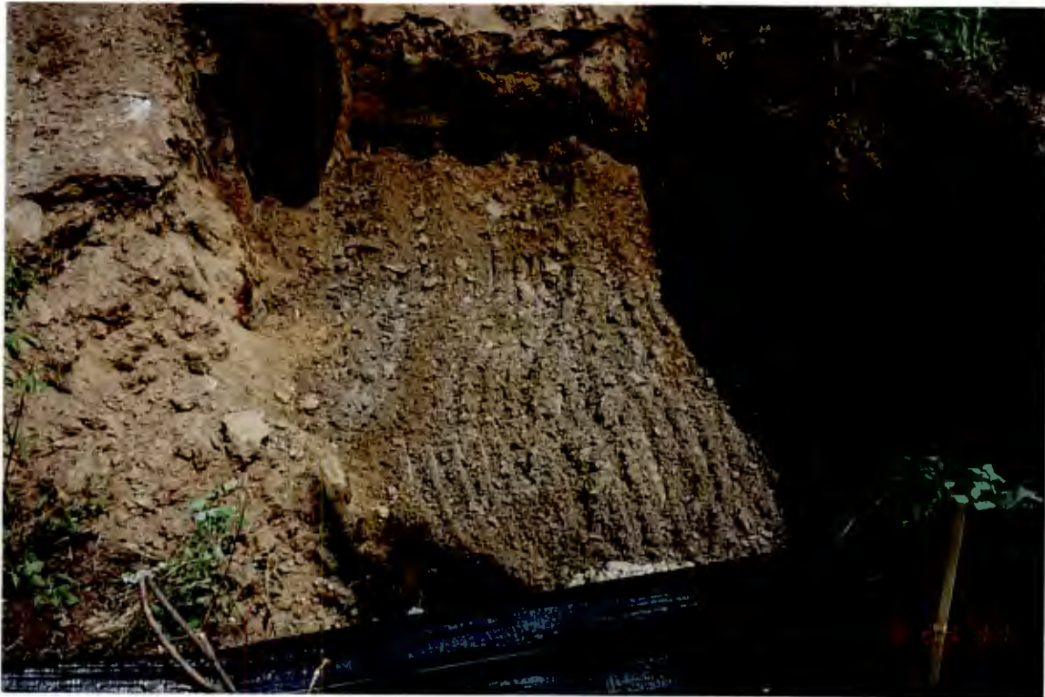
Photograph #3: Excavation of source area BL-16S completed.
