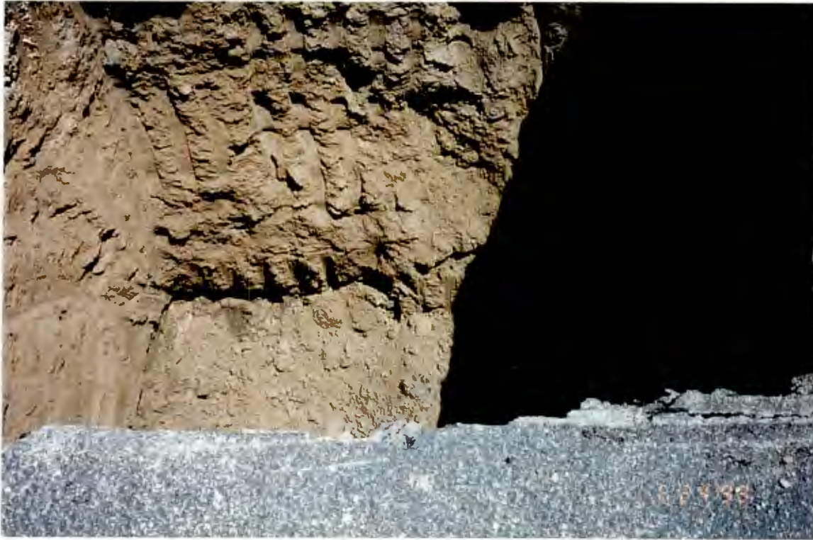
Photograph #9: Excavation of source area BL-11D completed.
