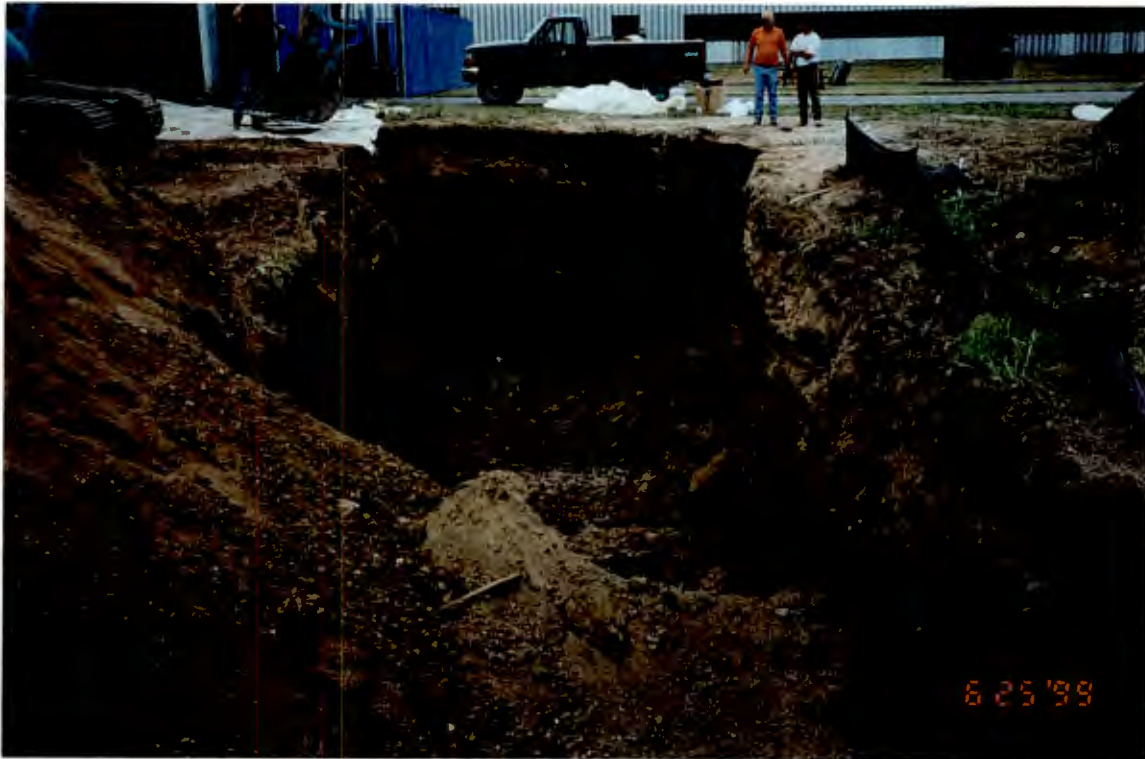
Photograph #7: Excavation of source area BL-9S in progress (Section 2).
