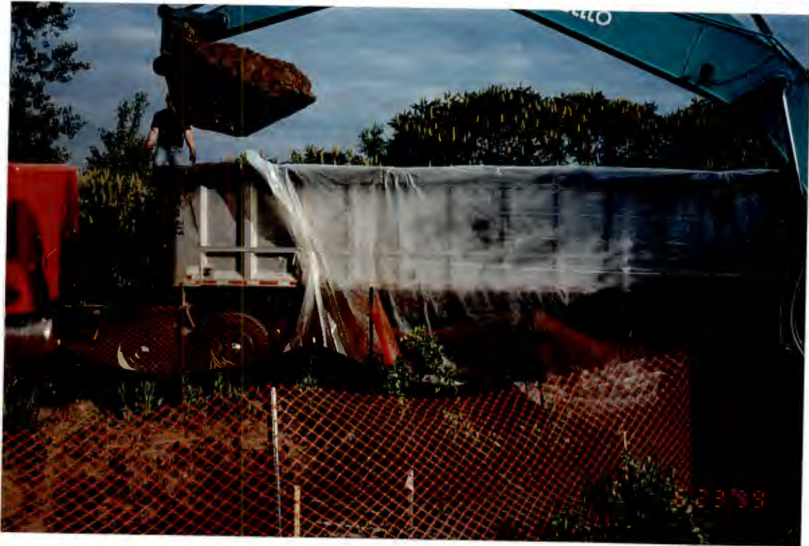
Photograph #1: Source area loaded into dump trailers for off-site disposal.
