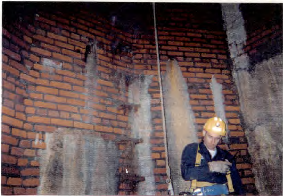
4. Ladder is on north wall of shaft.
