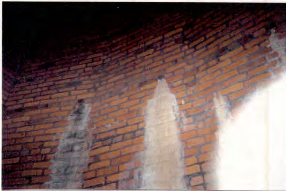
2. Built-in weep holes in south wall of shaft at Station 72+90.
