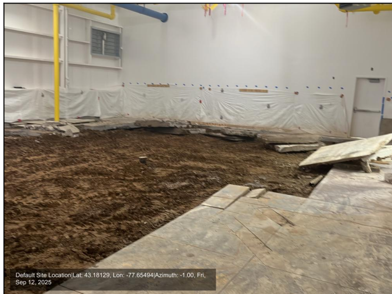
Photo Number: 6 Day 2 progress
