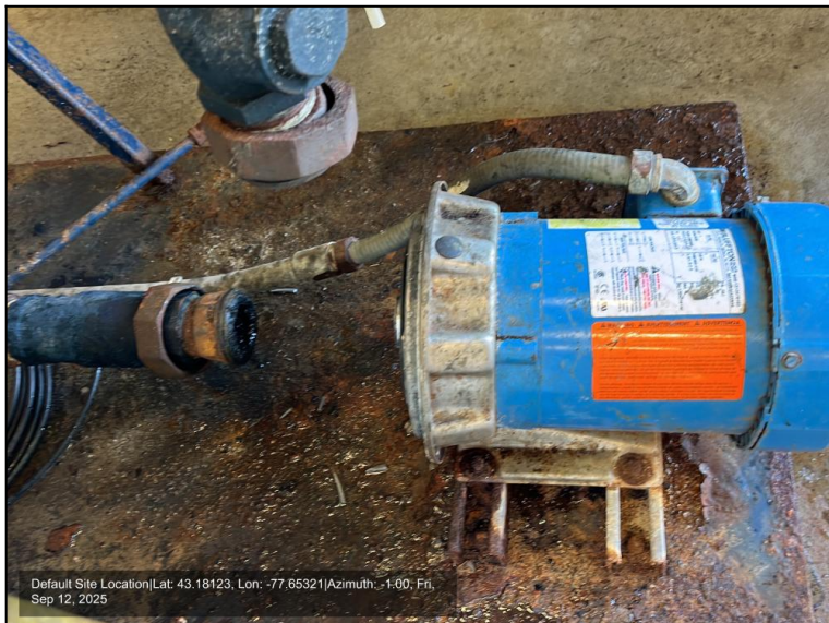
Photo Number: 3 EWTA, air stripper pump repairs
