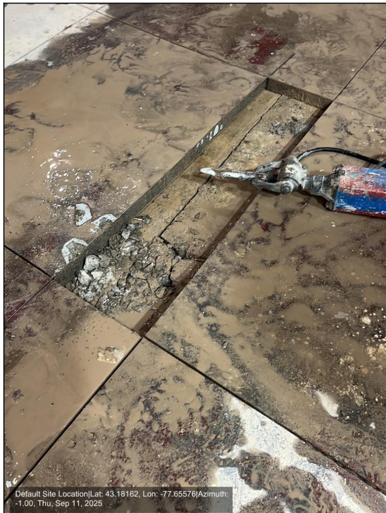
Photo Number: 1 second layer to concrete
