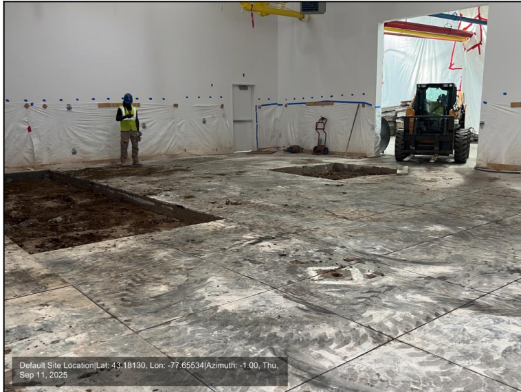
Photo Number: 6 Area removed, little to no VOC reading.
