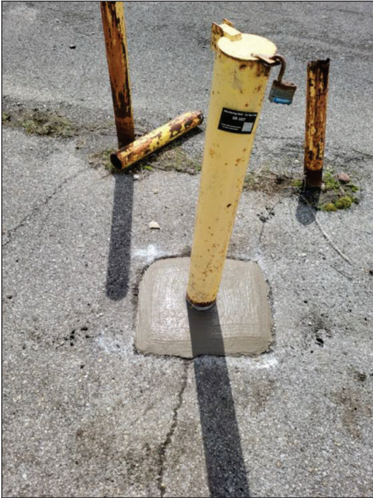
Photo Number: 17 SR-107 with new concrete seal.
