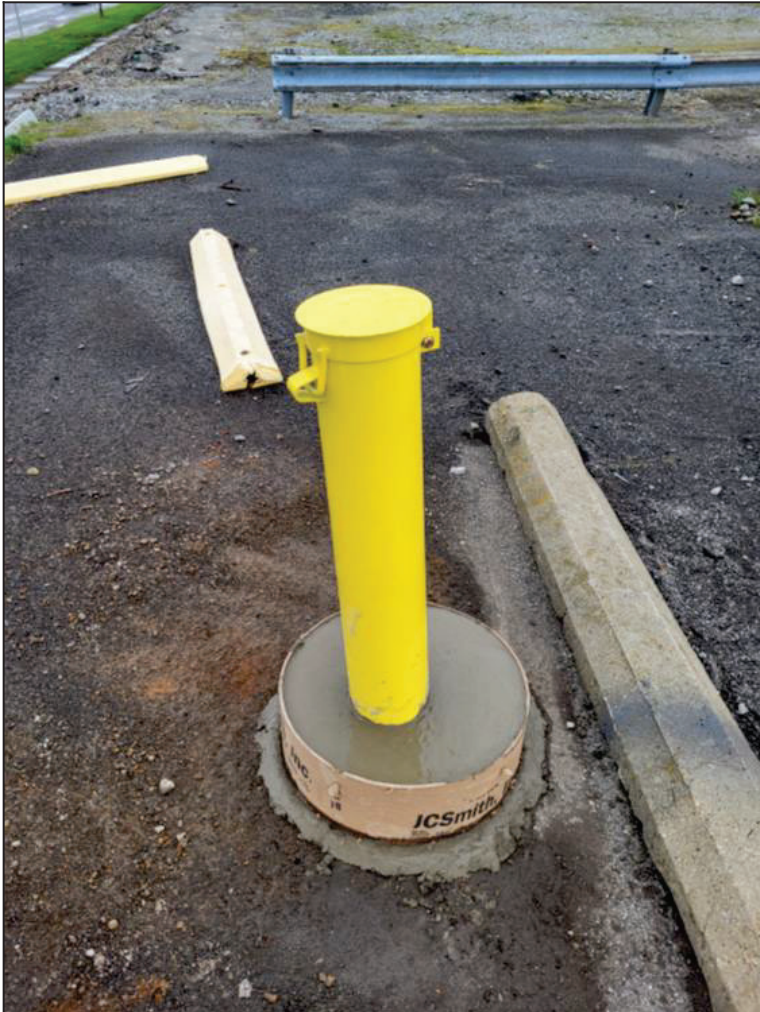
Photo Number: 6 DR-109 with new outer casing and concrete seal.
