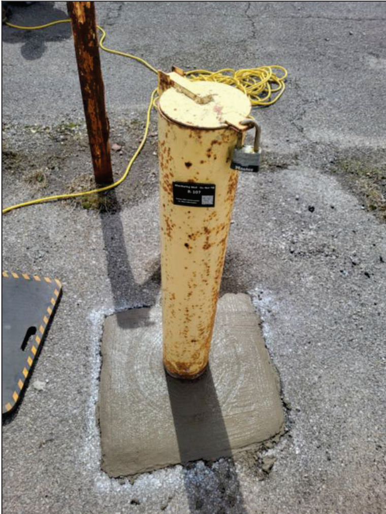
Photo Number: 18 R-107 with ne concrete seal.
