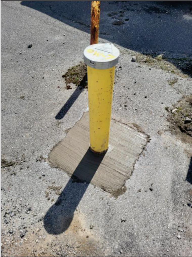
Photo Number: 19 OW-7 with new lid and concrete seal.
