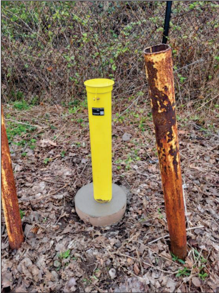
Photo Number: 2 R-2 with new outer casing and concrete seal.
