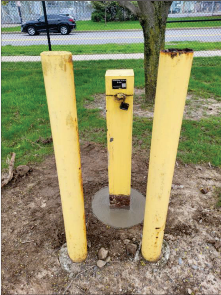
Photo Number: 13 R-235 with new concrete seal.
