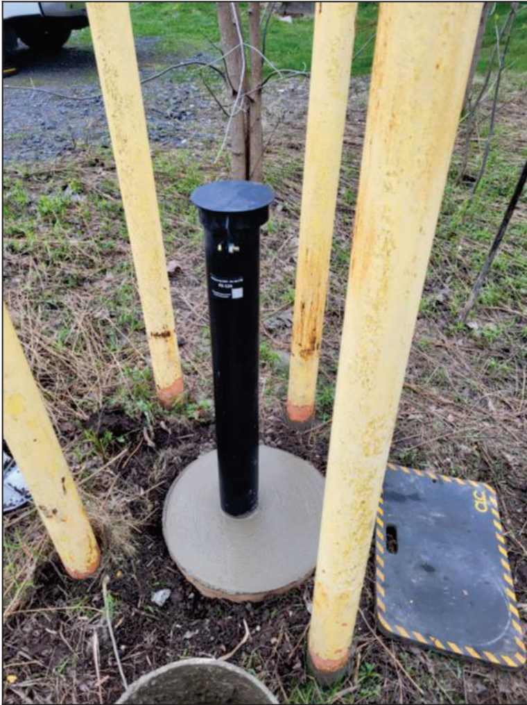
Photo Number: 5 PZ-124 with new casing and concrete seal.
