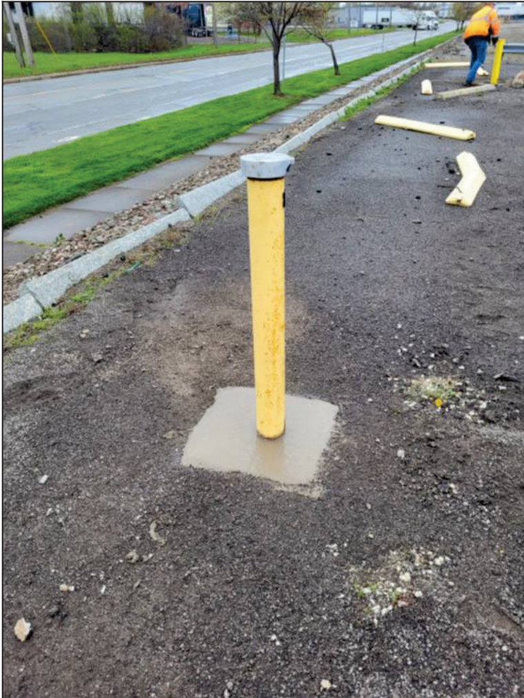
Photo Number: 5 SR-9 with new concrete seal.
