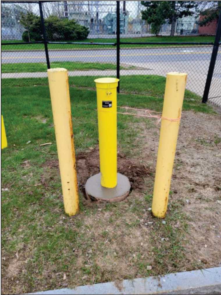
Photo Number: 12 SR-235 with new casing and concrete seal.
