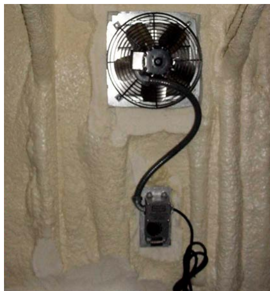
Complete Exhaust Fan (Interior View)
