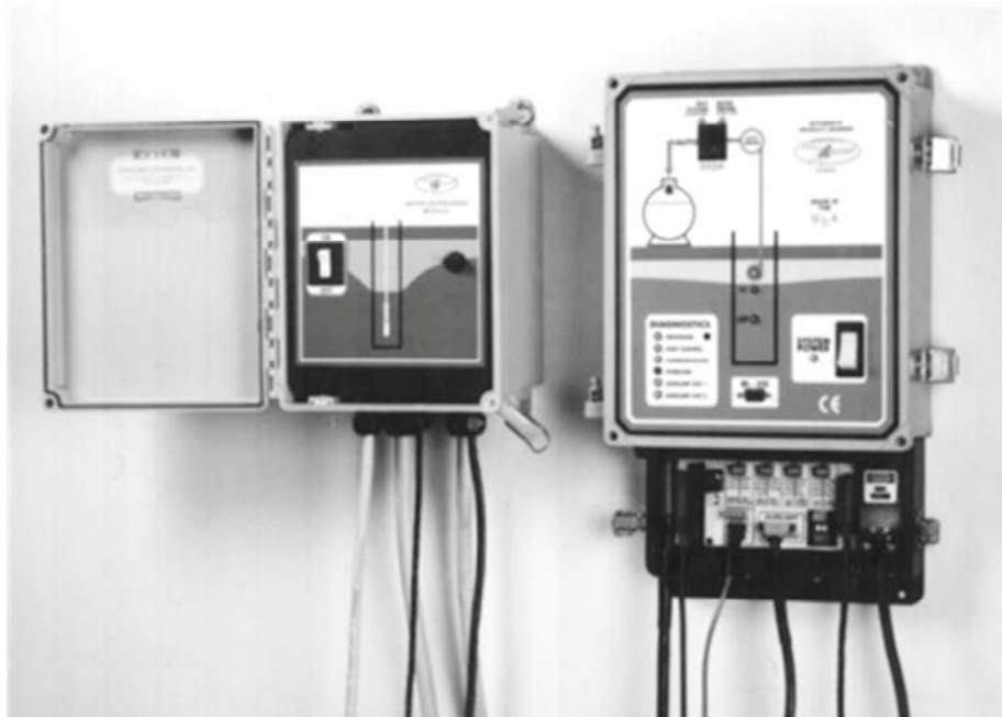
Typical installation of a Water Depression Control Module alongside a Magnum Spill Buster Control Panel
