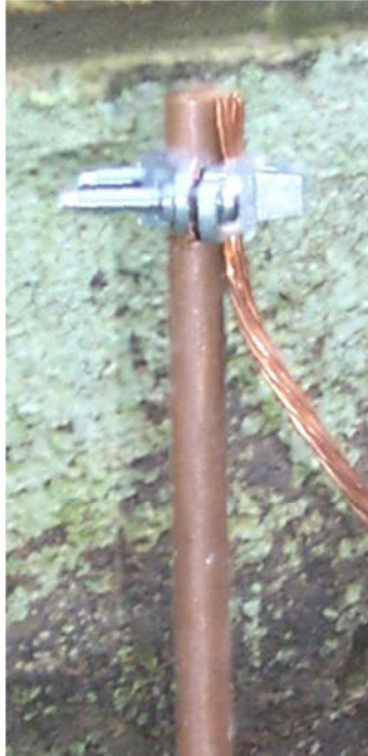
A grounding rod employing a 5/8" copper rod, 8 gauge wire and copper clamp.
