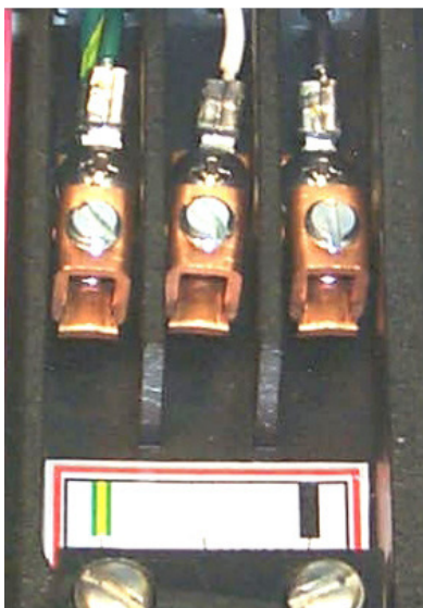
Terminal Block shown with the protective cover removed
