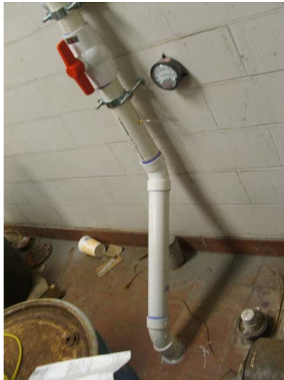
SSD – Typical Stack to Fan with Manometer
