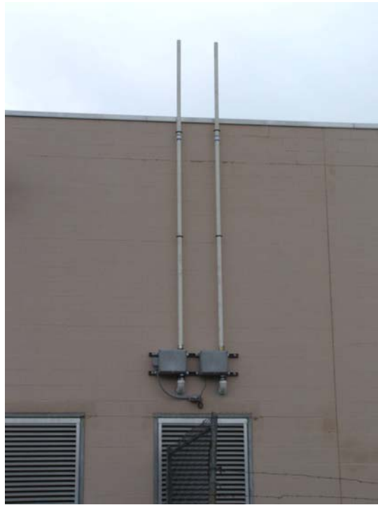
Northern Exterior Wall – SSD Fans and Exhaust
