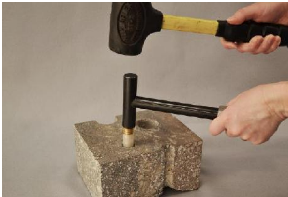
Figure 2. Installing the Vapor Pin™.
