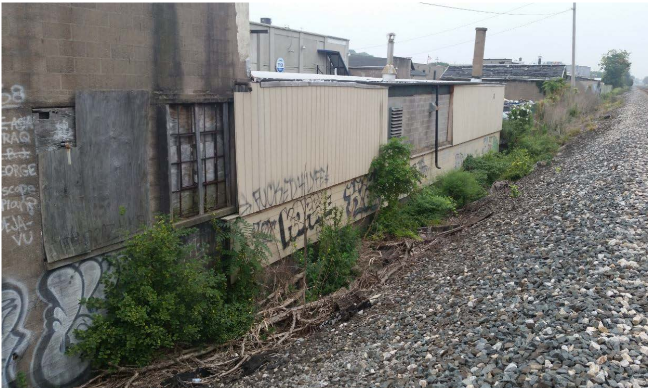
Exterior of North Side (exterior of kiln fan in center) - 2015
