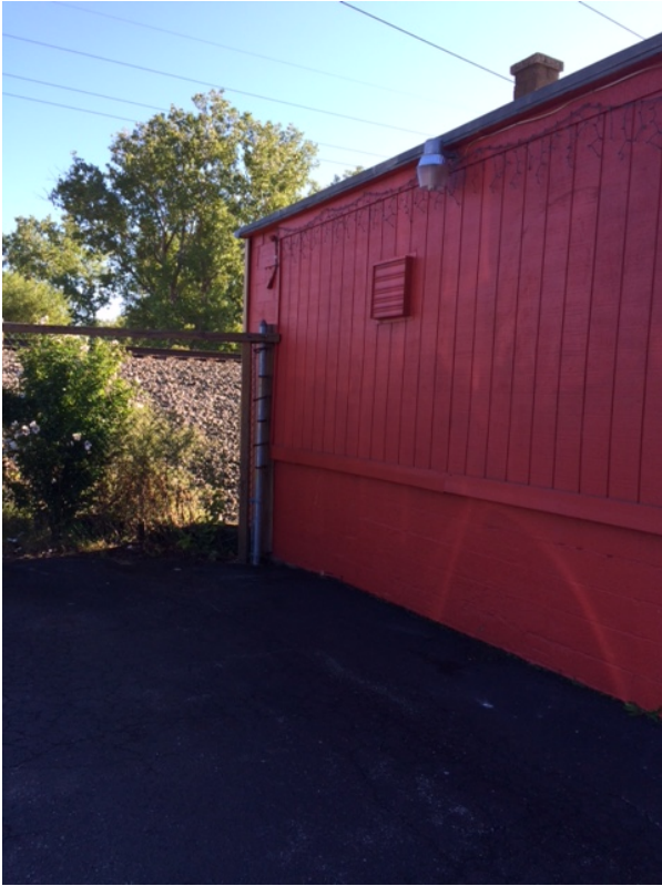
Exterior West Wall (outside of fan in photo to right) -2015
