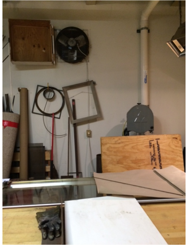
Interior Tool Room (inside fan) (New Suction Point 5 – September 2015
