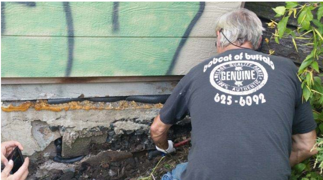
Sealing gaps with rigid insulation September 2015
