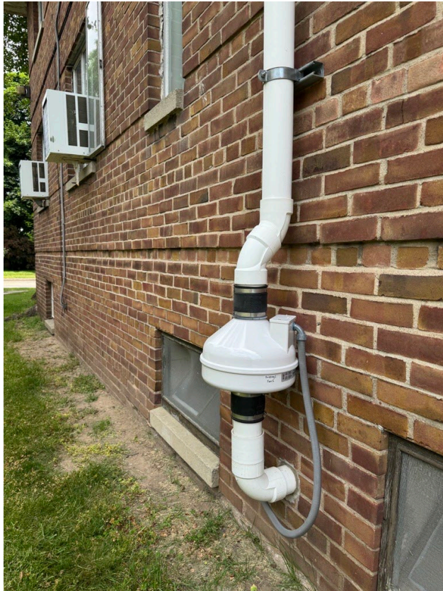
Above – Image of fan after replacement at Building 2 Fan 1.
