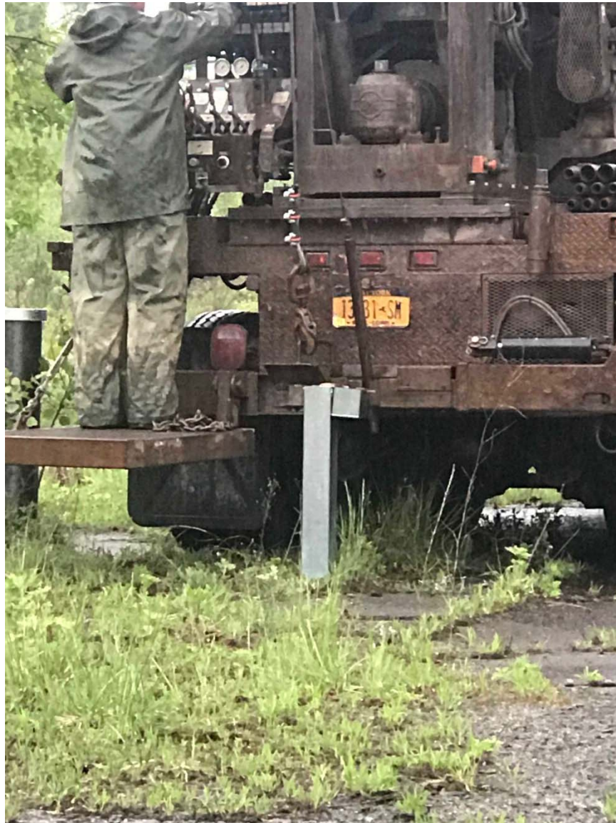
Photo No. 1 – Driller set up on URS-03 to begin well abandonment
