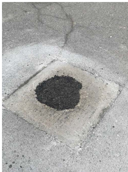
Photo No. 2 – OW-10S after completion of abandonment and asphalt patched at surface
