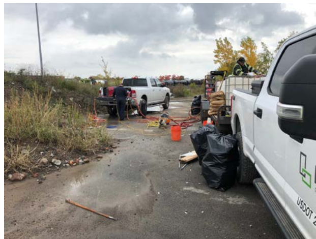
Facing east. Injection setup showing air tank connected to bladder system, injection hose running from 250-gallon cube to well, air compressor, and pump. (10/27/2020)
