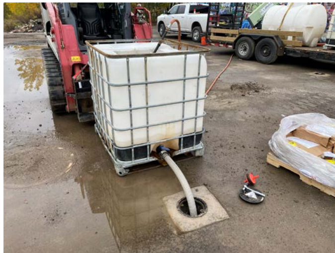
Facing east. Gravity feeding PersulfOx solution from 250-gallon cube into monitoring well MW-17R. (10/28/2020)
