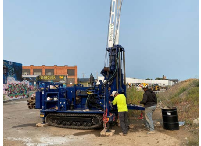
Facing west: LaBella using an auger at MW-17R and containerizing soil cuttings. (9/15/2020)
