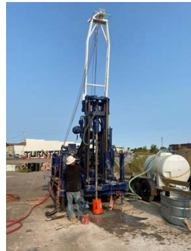
Facing west: LaBella using rotary drill bit at IW-01 to clear grout from rock socket before drilling with NX-core barrel. (9/16/2020)
