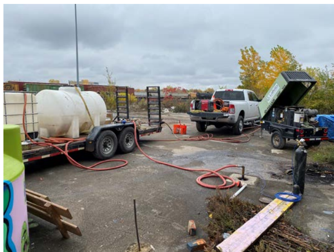
Facing northeast. Injection setup at MW-8R showing cube containing PersulfOx solution, generator, air compressor, air tank for the bladder packer system, and the injection hose in the well. (10/28/2020)
