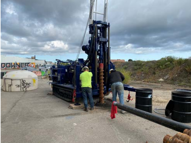
Facing northwest: LaBella using an auger to drill through overburden at IW-01. (9/14/2020)
