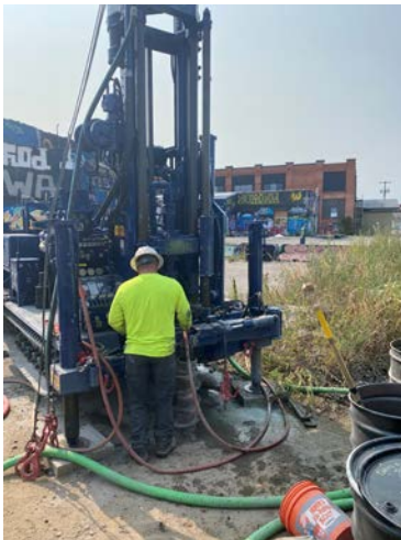
Facing southwest: LaBella deploying grout to secure the casing at MW-17R. (9/15/2020)
