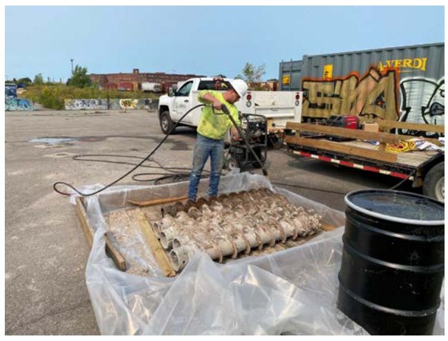
Facing northwest: LaBella deconning equipment on a decontamination pad with decontamination water. IDW drum in foreground. (9/16/2020)
