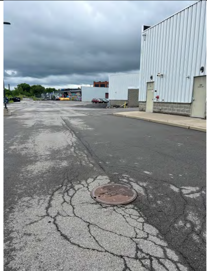
Photo 2: Looking East, manhole west of Site
