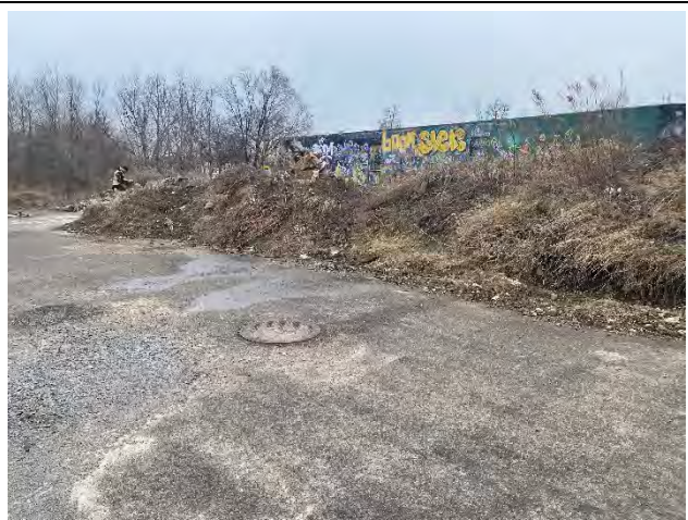
Photo 14: Pile of debris and brush in the middle of the site that has been asked to be removed
