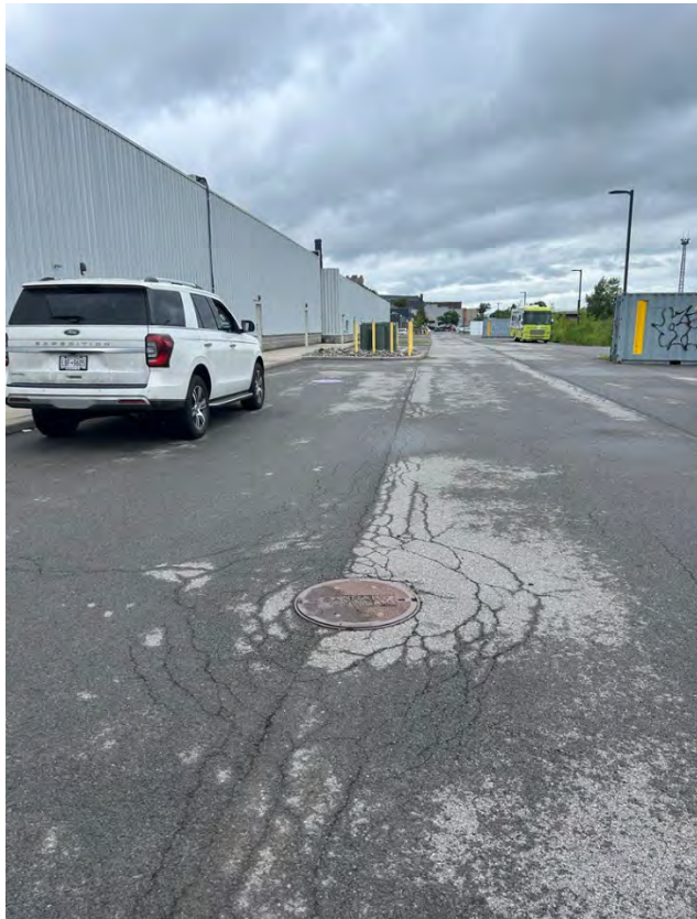
Photo 1: Looking West, manhole west of Site
