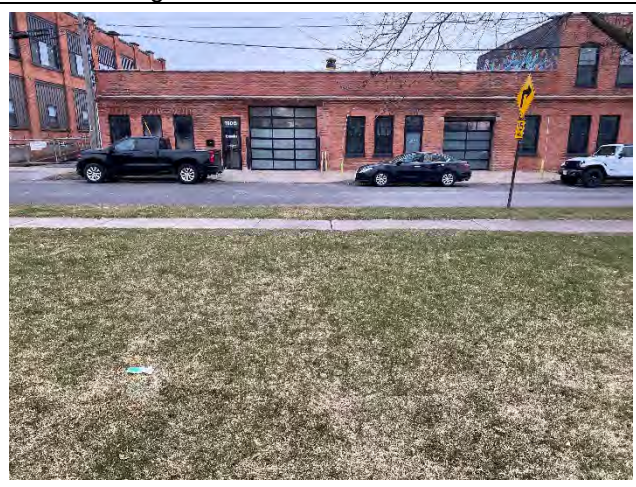
Photo 28: Front view of Anderson Ave buildings with entrance gate to site to the left. Gate has a lock but was unlocked and able to access
