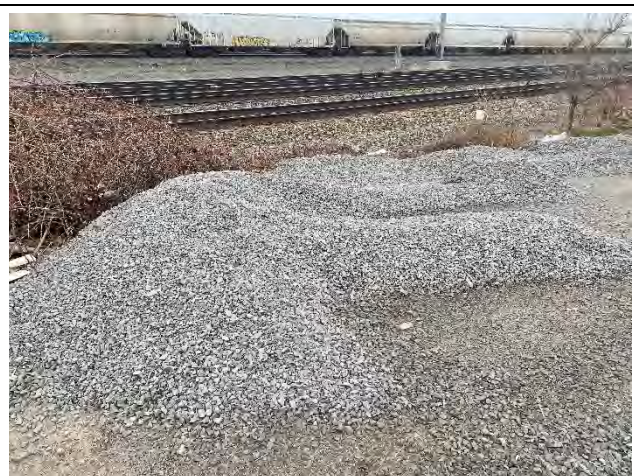
Photo 12: Staging pile of stone that has been asked to be removed
