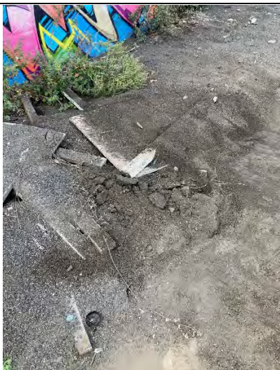
Photo 21: MW-8R buried under pile
