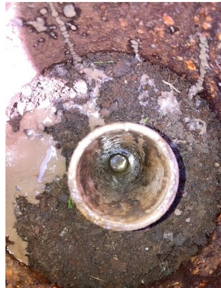
Picture of MW-11K showing sediment obstruction at ~2 feet.
