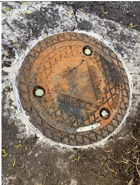
MW-10K with added sealant
