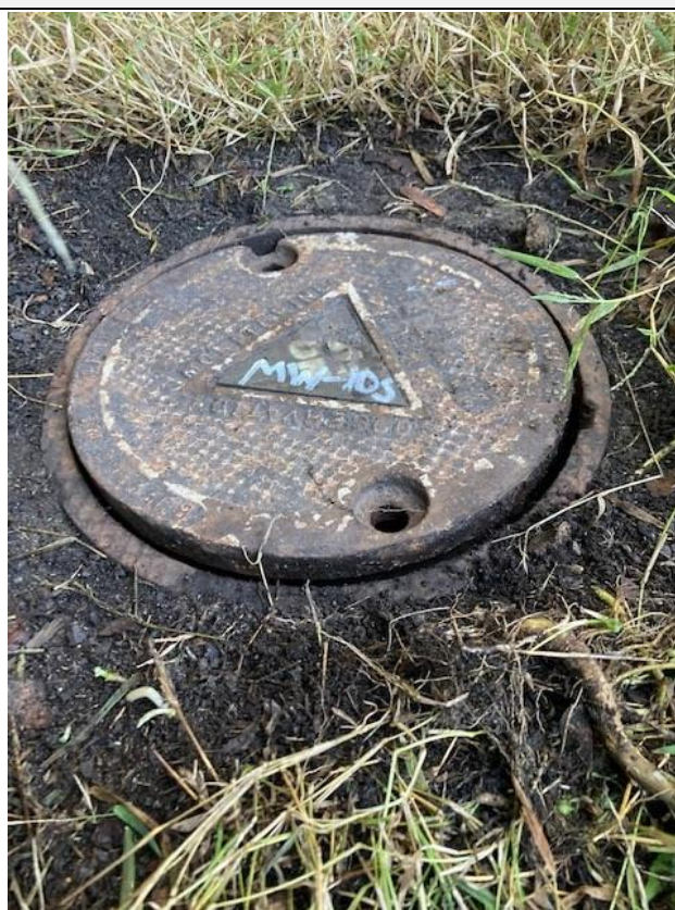
MW-10S not flush with J-plug
