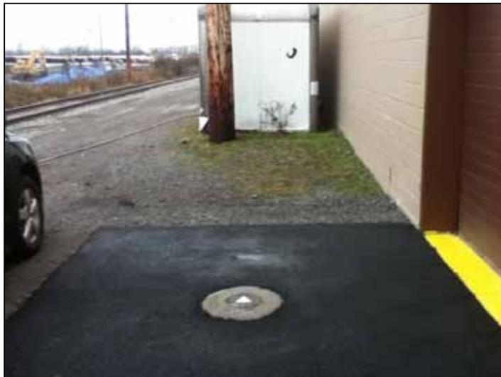
Excavation Area 4 located on western side of site building. The curb box shown in the center of asphalt patch was the access point for manual injection of permanganate solution.
