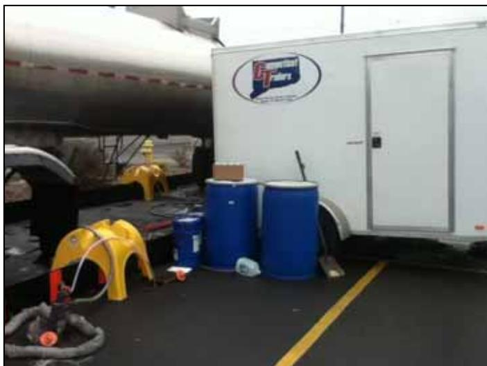
Storage Trailer and spill response staging area. Poly drums contain spill booms, spill pads and sodium thiosulfate neutralizing agent for addressing a potential sodium permanganate release. MW-16i is shown in the bottom left corner of the picture
