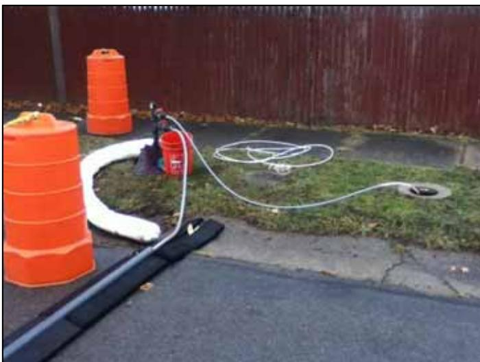
MW-17i (on the left) and MW-17s located on southern side of Jay Street. Hose ramps were used to protect injection solution while in transport from the tanker to injection well. The overflow valve on the wellhead manifold was retrofitted to direct solution to MW-17s.
