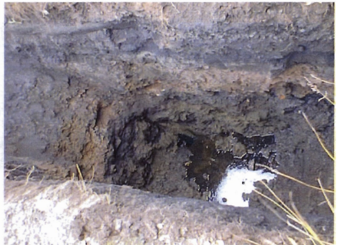
Photograph No. 6 - Dark product was observed on top of water that accumulated at base of test pit TP-3. A sample of this product mixed with water was collected for full TCL/TAL laboratory analysis.
