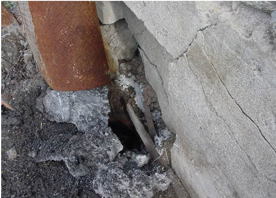
Photo 2: Closer view of access hatch/fill port rim beneath rubble.
