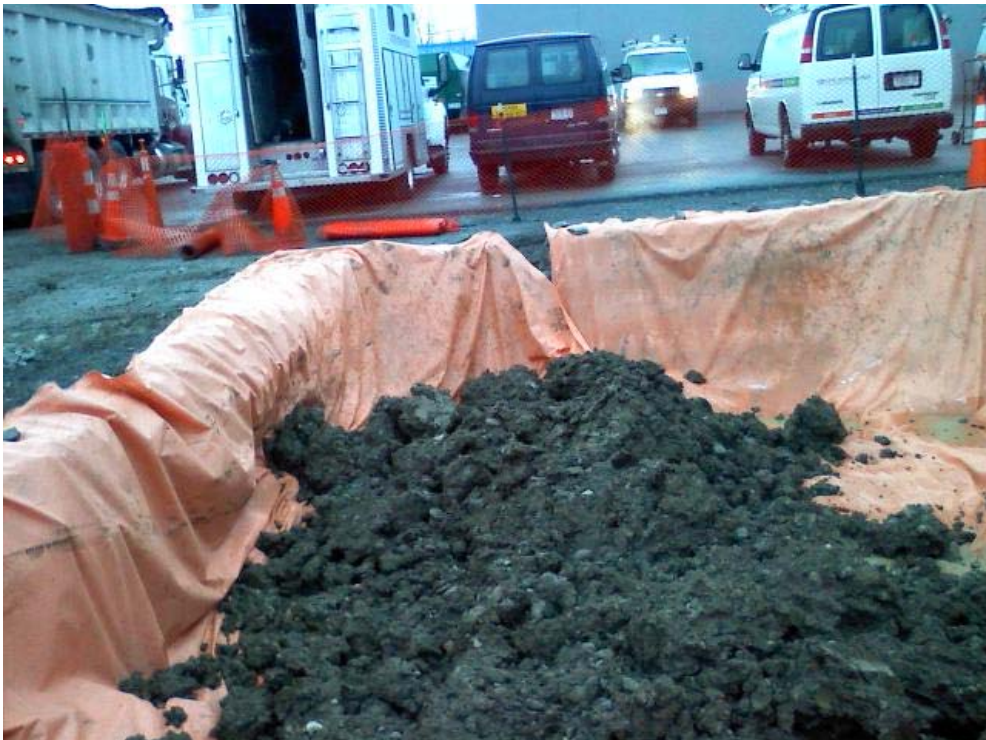
Photo #20, view to the east: depicting placement of orange demarcation fabric and backfilling activities in Area 1A.
