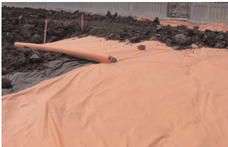
Placing Mirafi® Orange delineation fabric.
