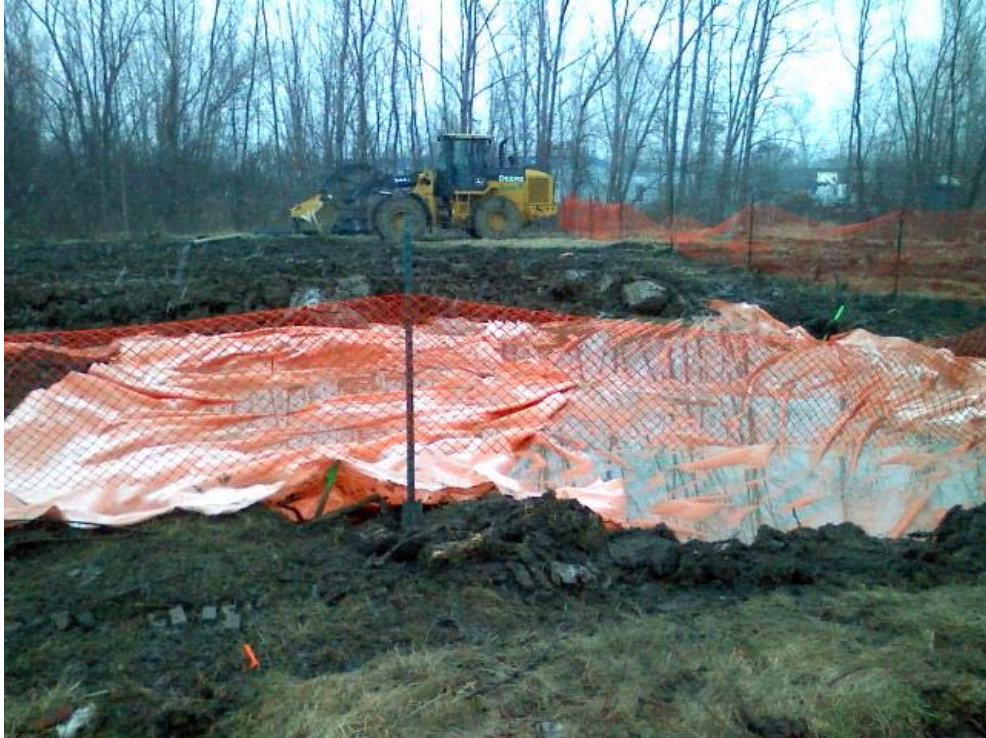
Photo #21, view to the north: depicting placement of orange demarcation fabric in the eastern and southern portions of Area 2C.
