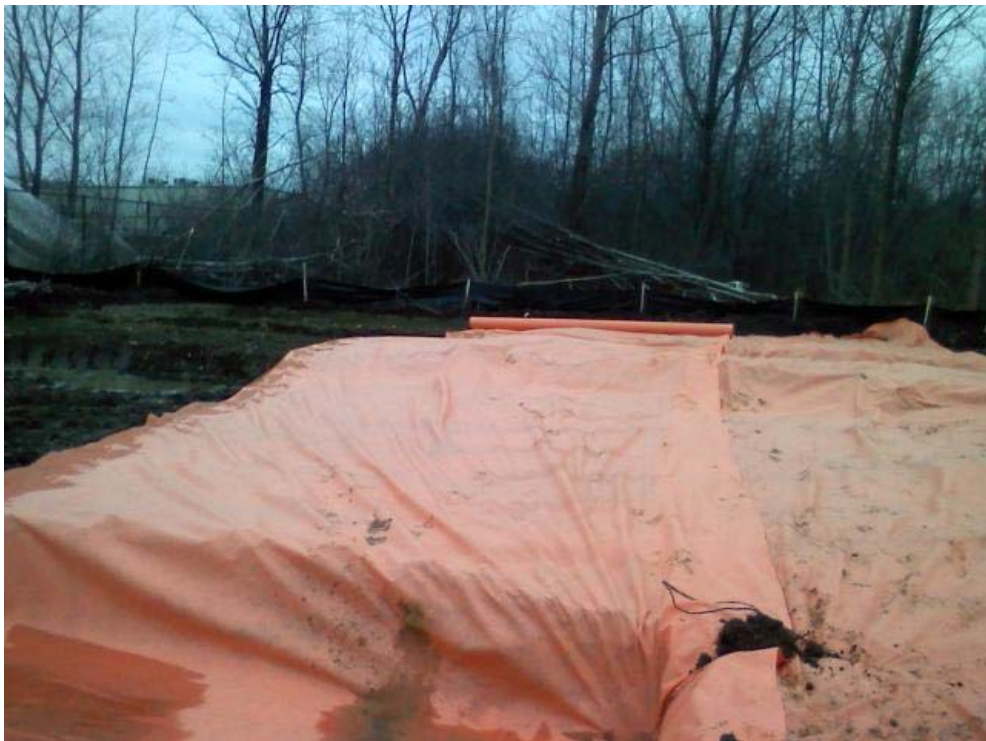
Photo #18, view to the north: depicting placement of orange demarcation fabric over areas 2A, 2B, and 1C.
