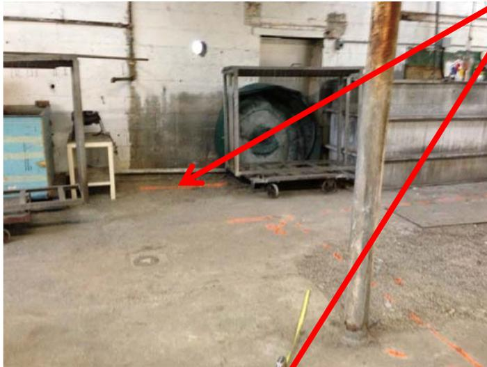
Location of Temporary Steel H-Columns to maintain 20.5-ft and 26.5-ft beam spans (spacing between the existing live electrical panels and temporary column locations can be increased as needed by reducing temporary beam length, up to 2-ft can be reduced, i.e., install 24.5-ft temporary beams)
