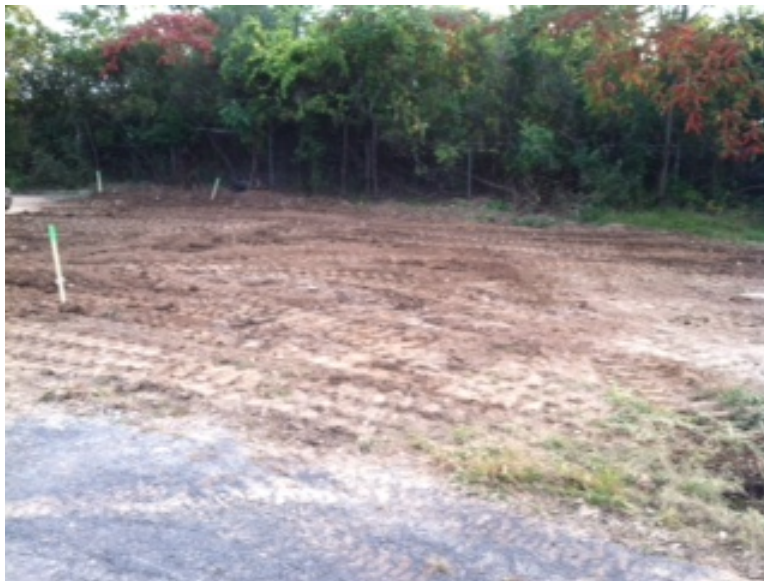
Operable Unit 01C (Outside Disposal Area) after backfilling is completed, and area is graded.
