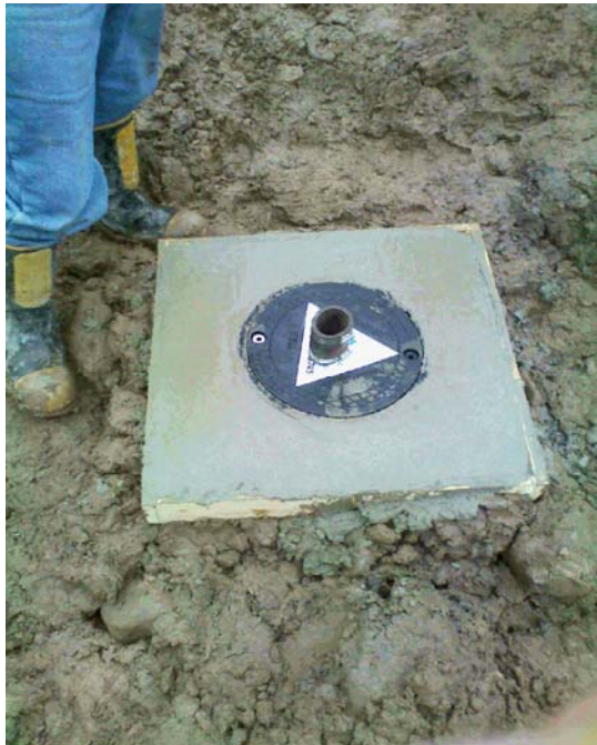
Completed well pad of INJ-2.
