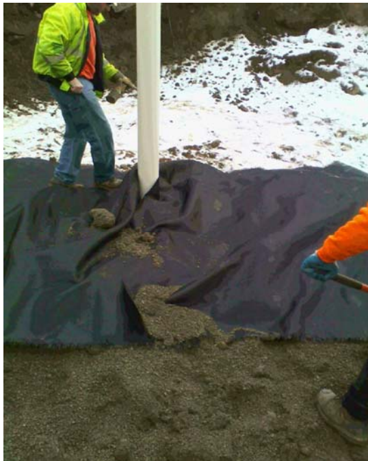
Construction of Injection Well INJ-1 within Operable Unit 01A (Former Drum Storage Area) excavation.
