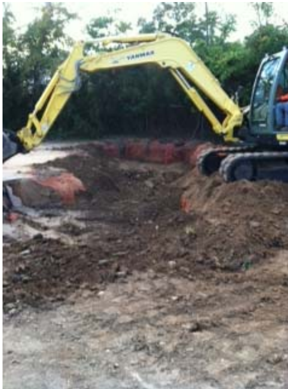
Backfilling Operable Unit 01C (Outside Disposal Area) extended excavation in September 2012.
