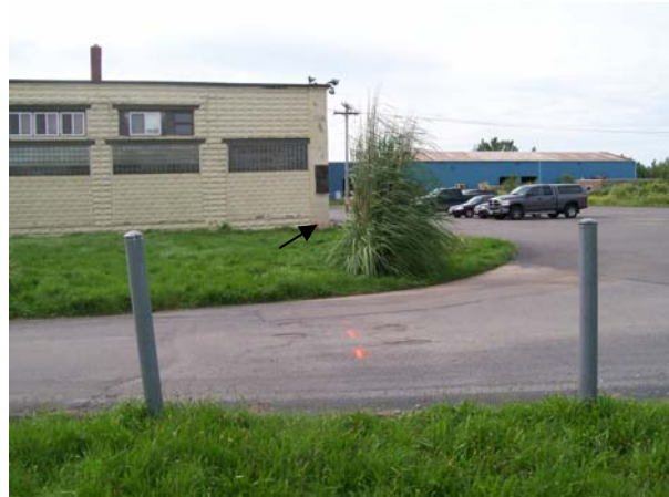
Photo No. 22. Northeast collection pit and piping to eastern collection pit.
