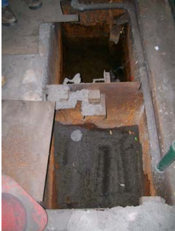
Photo No. 1. Catch basin along east wall of Welding Room.
