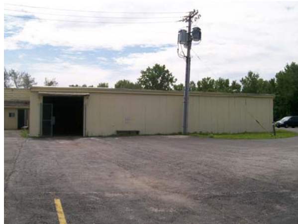
Photo No. 20. Northwest exterior wall.
