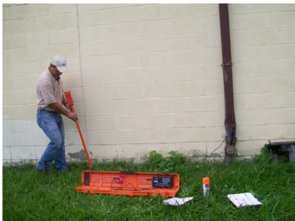
Photo No. 11. North-south pipe along the western exterior wall.
