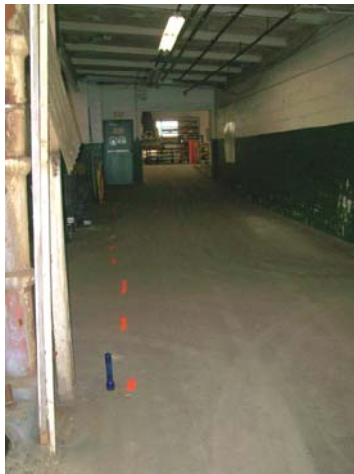
Photo No. 9. Pipe from Shear Room to Loading Dock, looking south.
