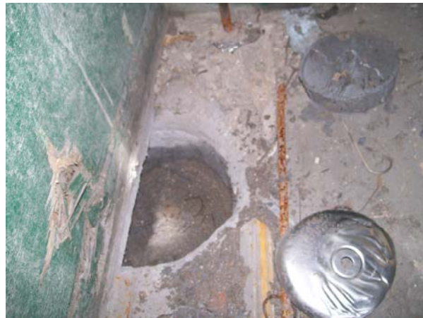
Photo No. 10. Floor drain by Paint Storage Area.
