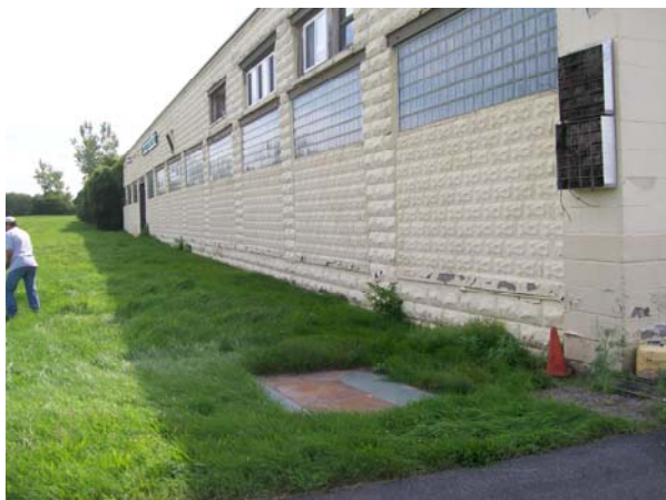
Photo No. 23. Northeast collection pit and eastern exterior wall looking south.
