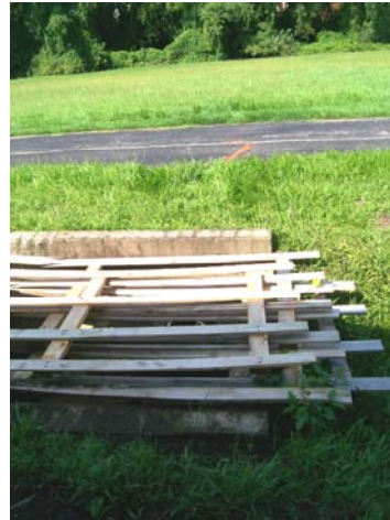
Photo No. 16. Central collection pit and piping looking west.
