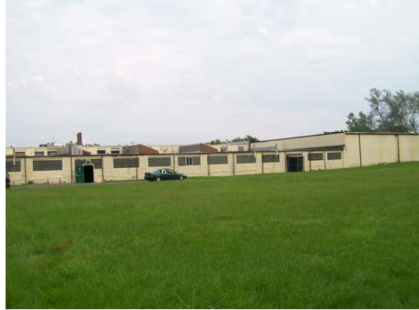
Photo No. 20. West exterior portion of the building.
