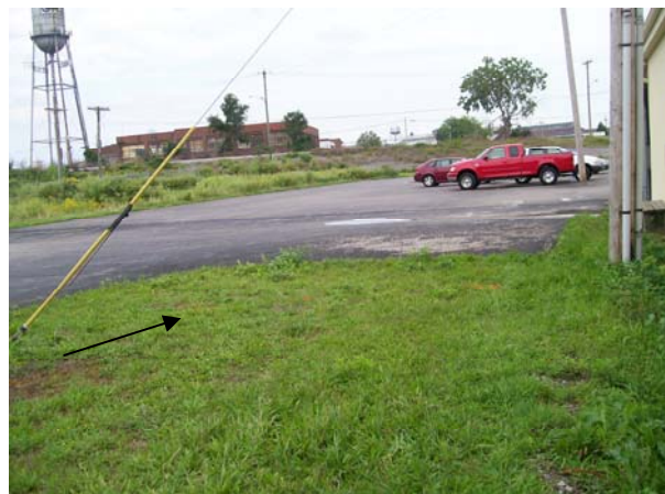
Photo No. 24. Piping northwest-southeast from the northwest exterior of the
