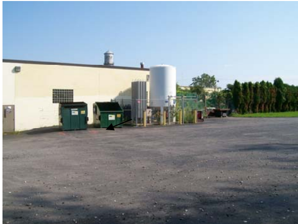
Photo No. 21. South exterior pipes and portion of the building.
