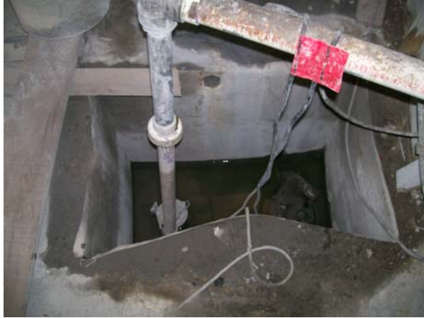
Photo No. 7. Catch basin in former Degreaser Area.
