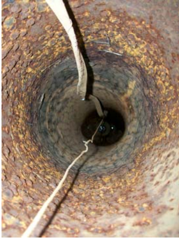
Photo No. 13. Production well interior.
