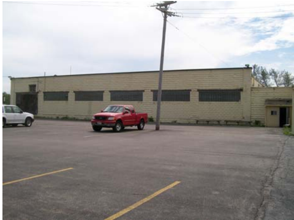
Photo No. 19. Northeast building exterior wall.
