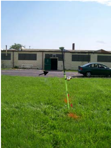
Photo No. 15. Pipes east-west from Welding Area exterior door.
