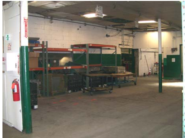
Photo No. 4. Piping/anomalies found in Welding Storage area, looking east.
