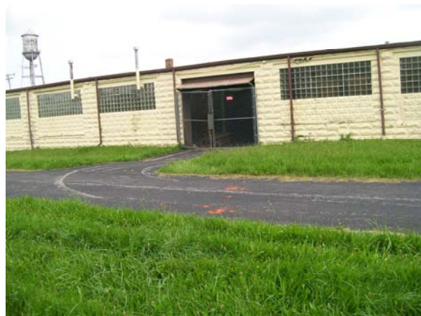
Photo No. 18. Pipes east-west from the overhead door in the Whistler Area.
