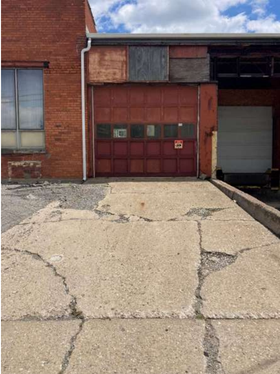
Photo 6 – At grade concrete slab (taken 7/26/22)
