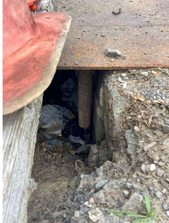
Photo 2 – Unknown pit block walls (taken 7/26/22)
