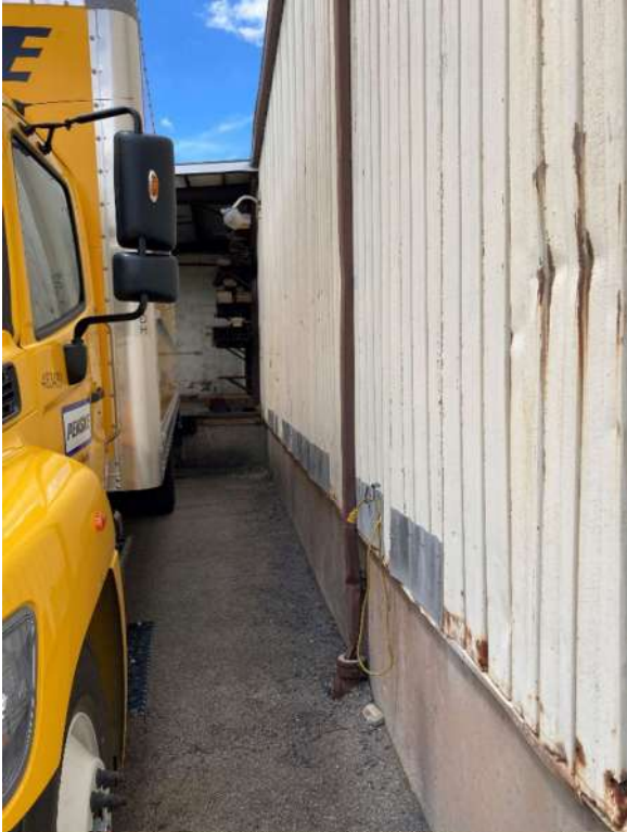
Photo 9 – Wall on north side of lot (taken 7/26/22)
