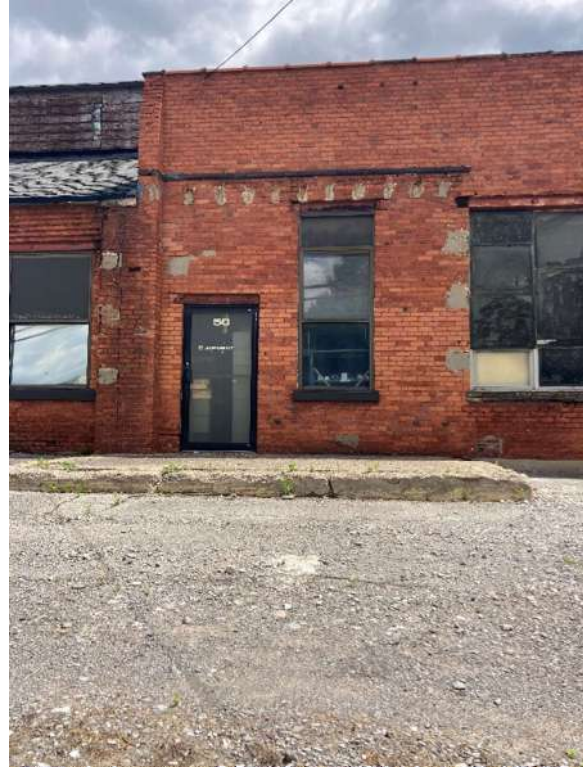
Photo 7 – Above grade conc. landing (taken 7/26/22)
