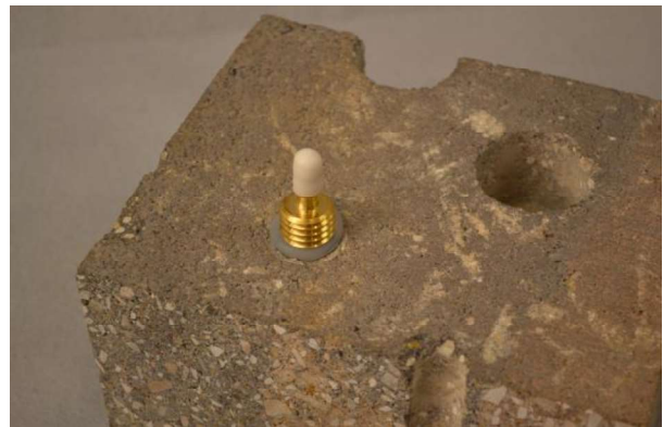
Figure 3. Installed VAPOR PIN®
