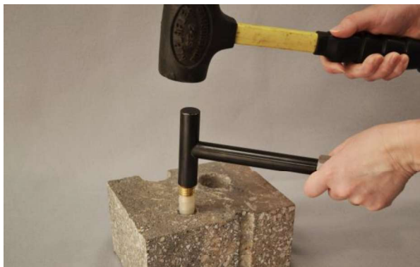
Figure 2. Installing the VAPOR PIN®
