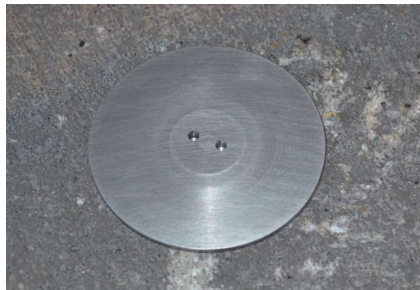
Figure 4. Secure Cover Installed
