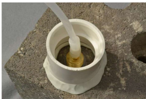
Figure 6. Water dam used for leak detection
