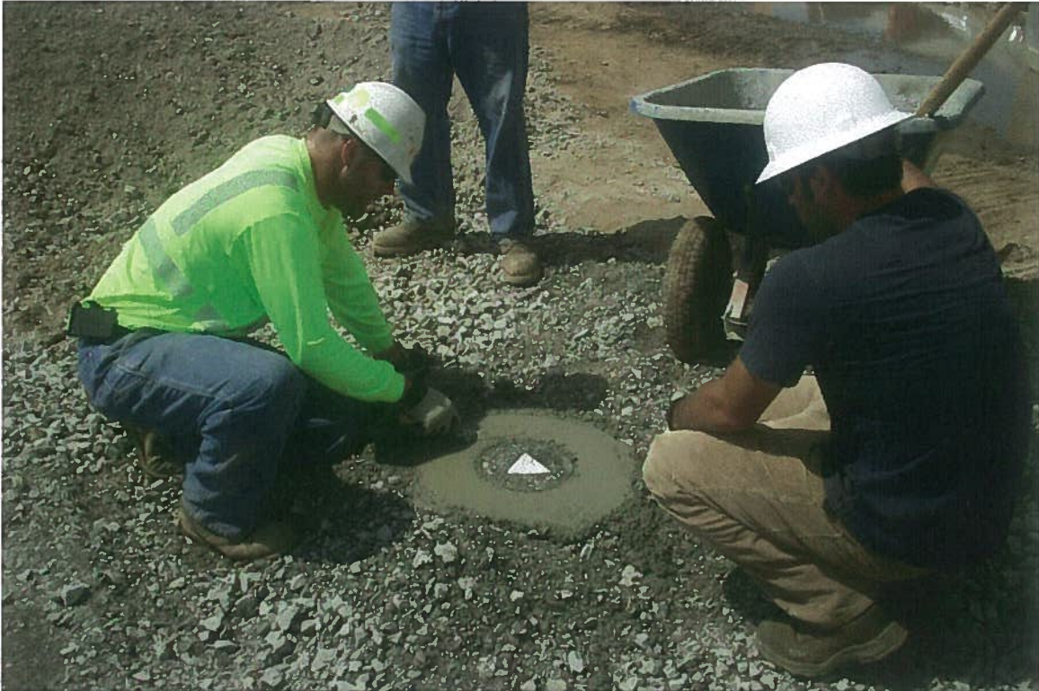
August 12, 2011: Retrofit of Monitoring Well MW-3 Flush Mount Completed
