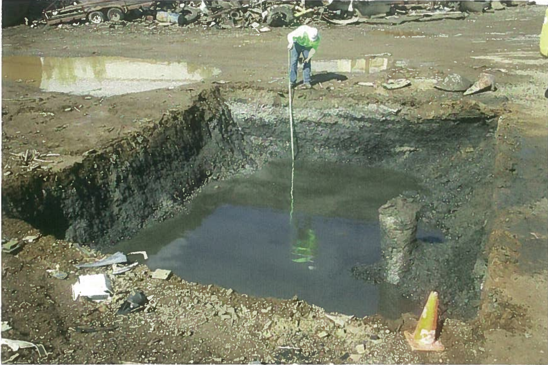
August 10, 2011: Soil Removal Excavation in Progress. Monitoring Well is in the Lower Right of the Photograph
