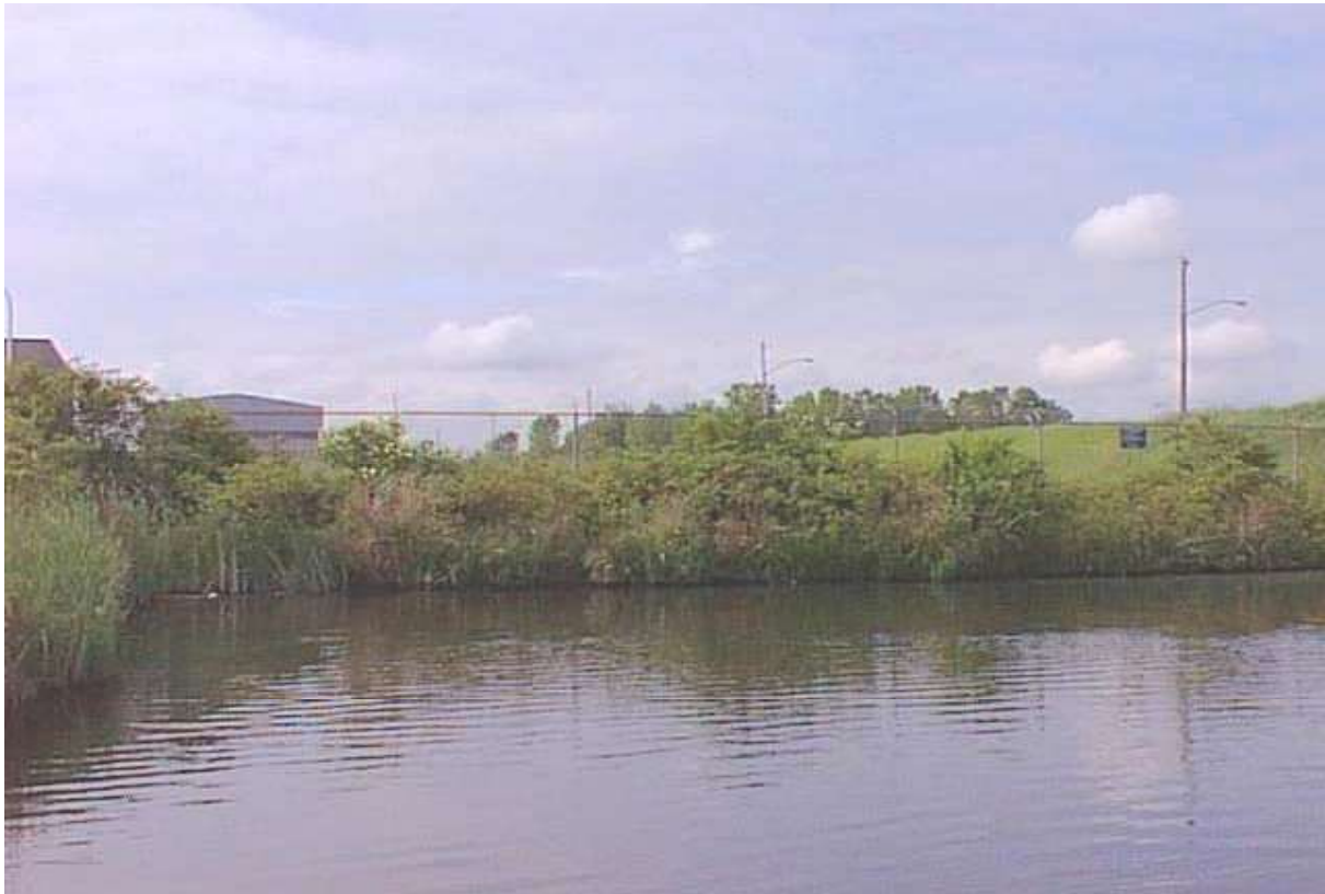
View of the downstream portion of Round Pond Creek North of Former Air Force Plant No. 51
